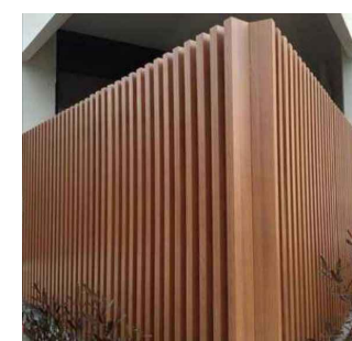
F 2" X 4" X 6" H. ALUM. FENCE 45° ANGLE FOR VISUALIZATION PRIVACY. COLOR: BROWN
