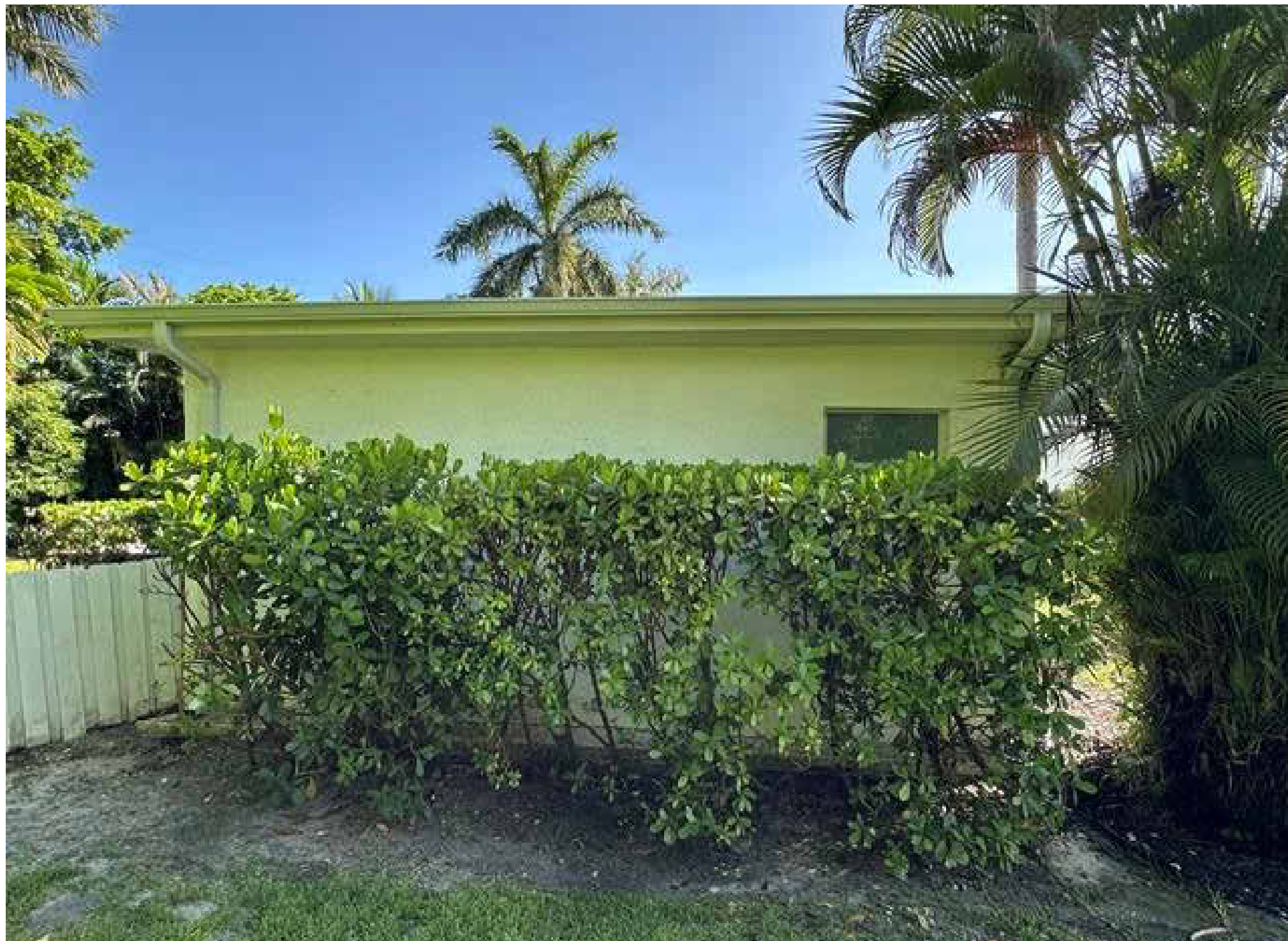
EXISTING FRONT NORTH EAST
