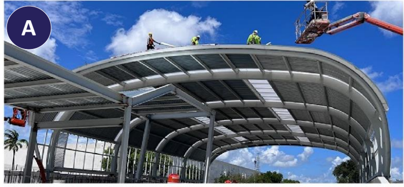
South Corridor: Bus Transit, under construction
