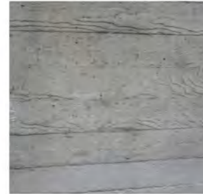
BOARD FORMED CONCRETE WALLS
