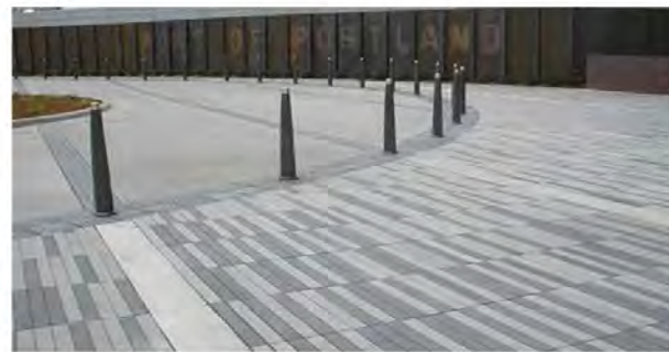
CONCRETE PAVER DRIVEWAYS
