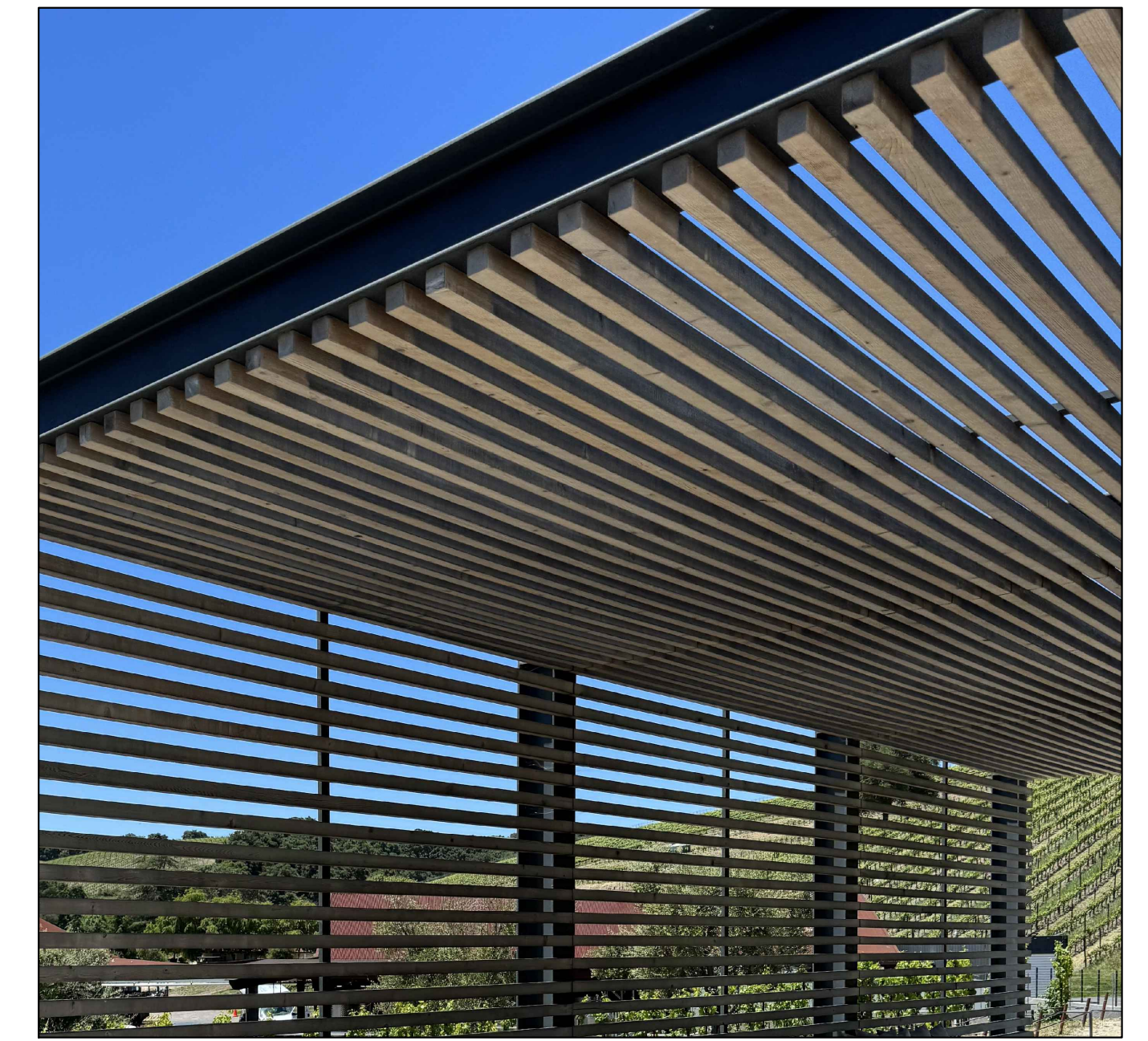
PHOTO FOR REFERENCE ONLY : FINISH MAY VARY ALUM. LATTICE (GRAY E.S.P. FIN.) ROOF TERRACES
