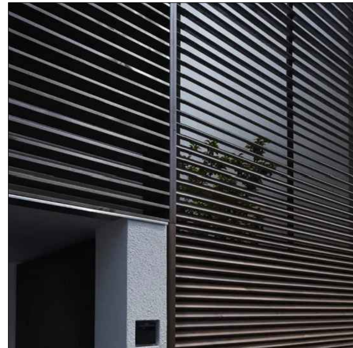
PHOTO FOR REFERENCE ONLY : FINISH MAY VARY ALUMINUM LOUVERS (GRAY E.S.P. FIN.)
