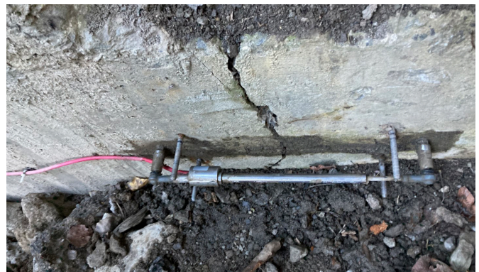
Model EDJ-40V Crack meter installed
