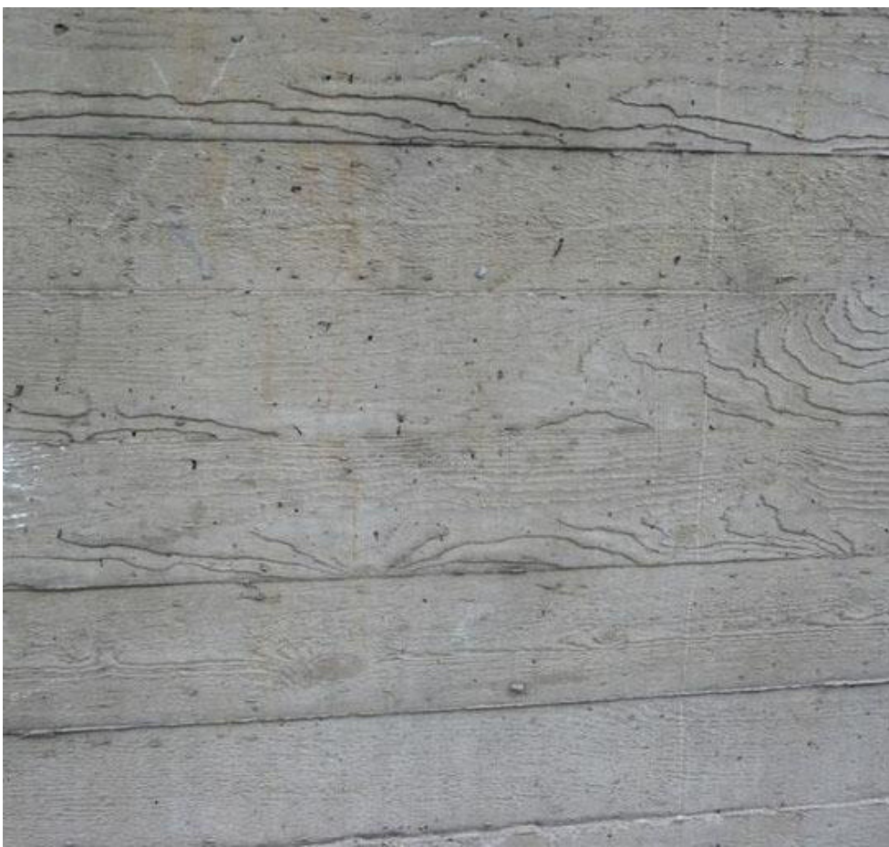
BOARD FORMED CONCRETE WALLS
