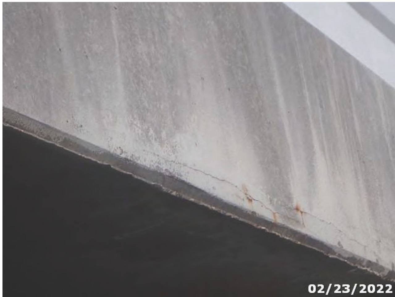
Photo 07 Element/Env 8099/4: PS Conc Slab (Sonovoid)
