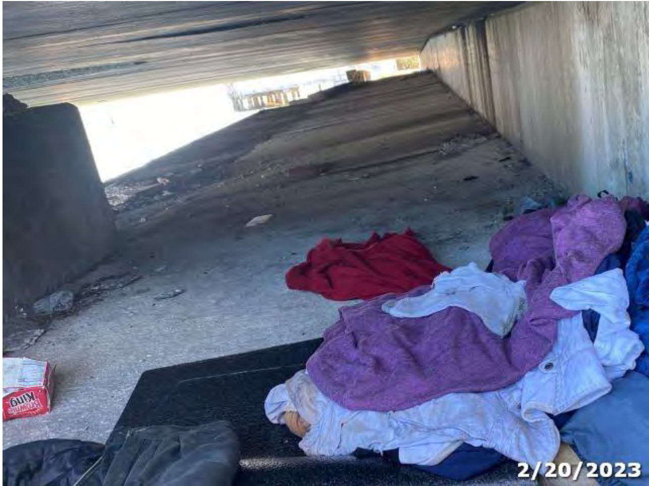
Photo 21 Element/Env 8394/4: R/Conc Abut Slope Protection
