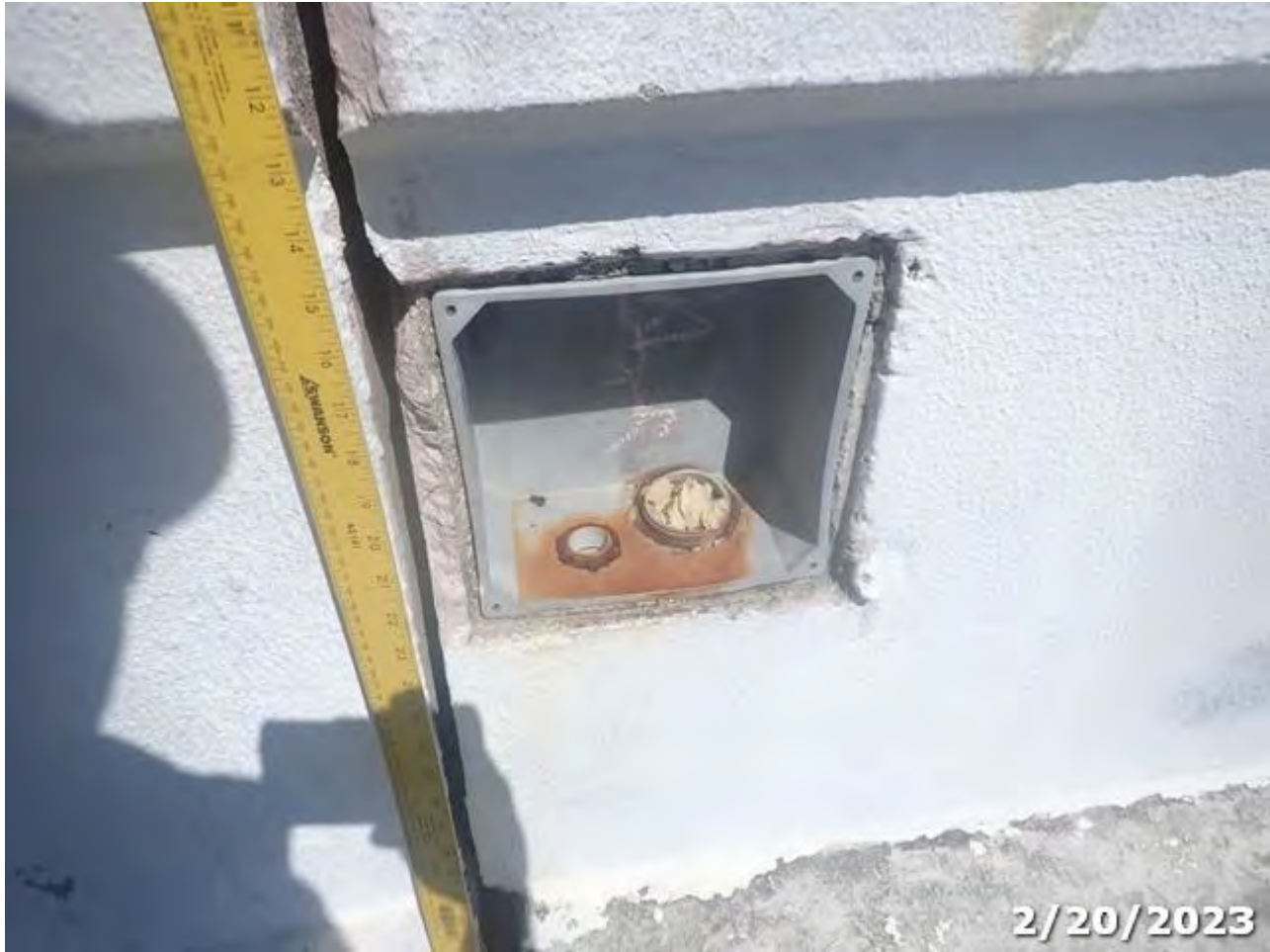
Photo 22 Element/Env 333/4: Other Bridge Railing
