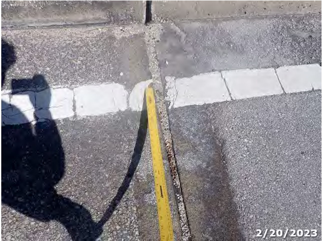
Photo 09 Element/Env 301/4: Pourable Joint Seal
