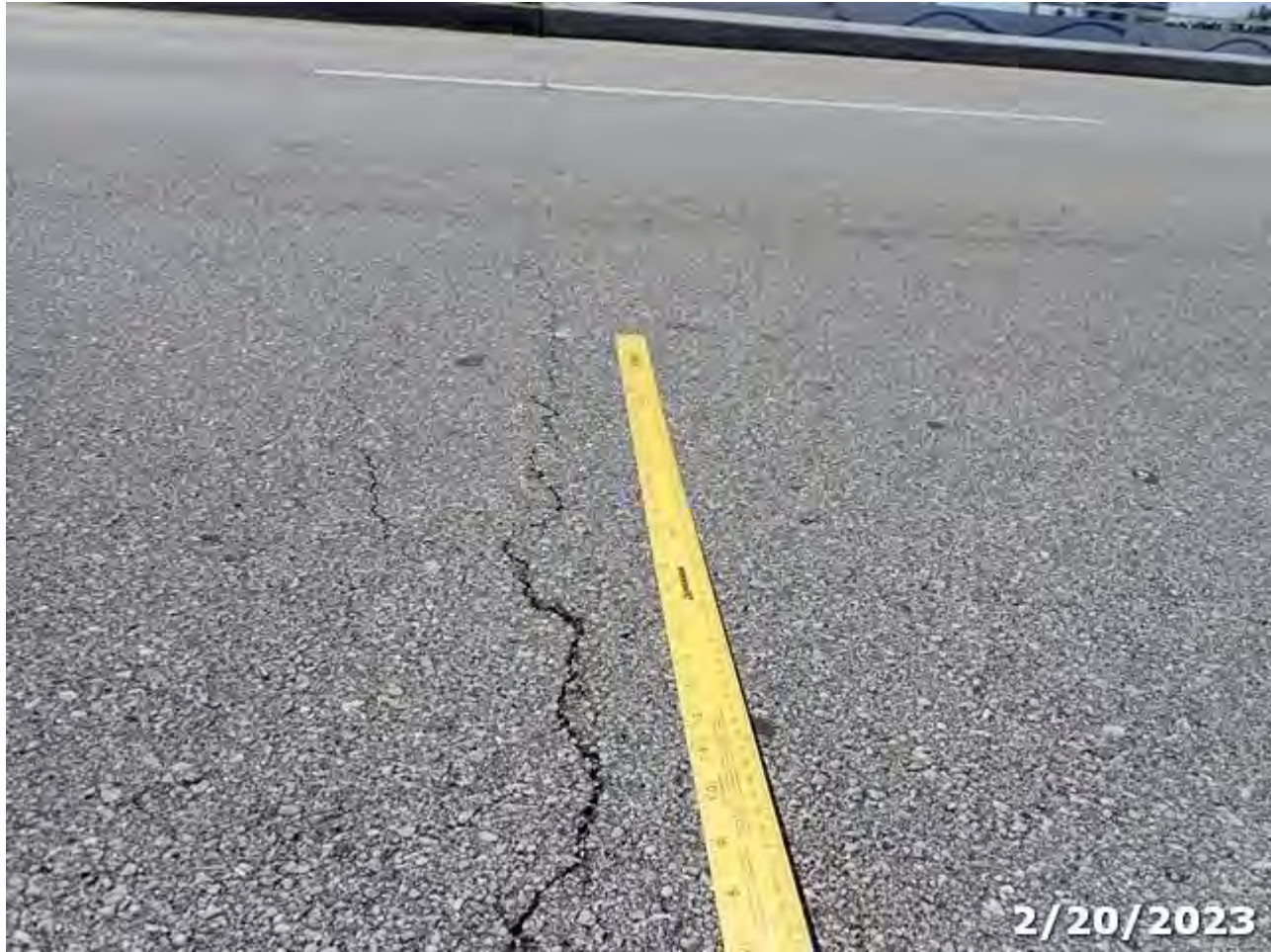
Photo 11 Element/Env 321/ 510/4: R/C Approach Slab/ Wearing Surfaces
