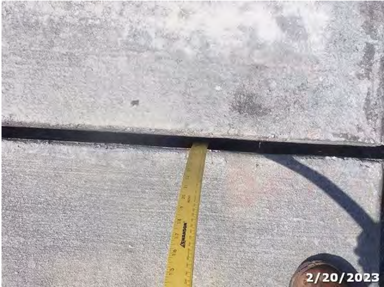
Photo 08 Element/Env 301/4: Pourable Joint Seal
