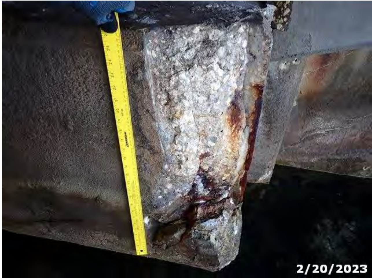
Photo 19 Element/Env 8393/4: Bulkhead Seawall Any Material
