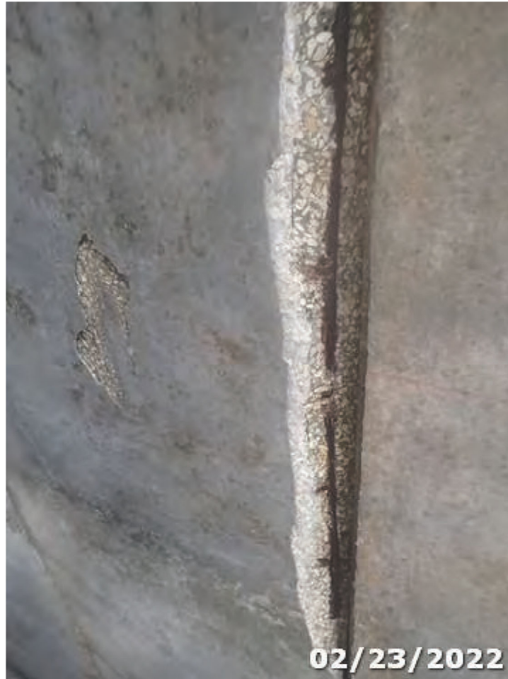
Photo 06 Element/Env 8099/4: PS Conc Slab (Sonovoid)
