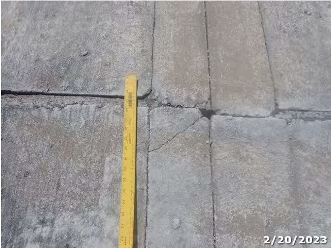
Photo 02 Element/Env 8099/4: PS Conc Slab (Sonovoid)
