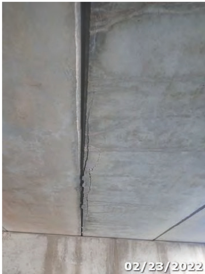
Photo 03 Element/Env 8099/4: PS Conc Slab (Sonovoid)
