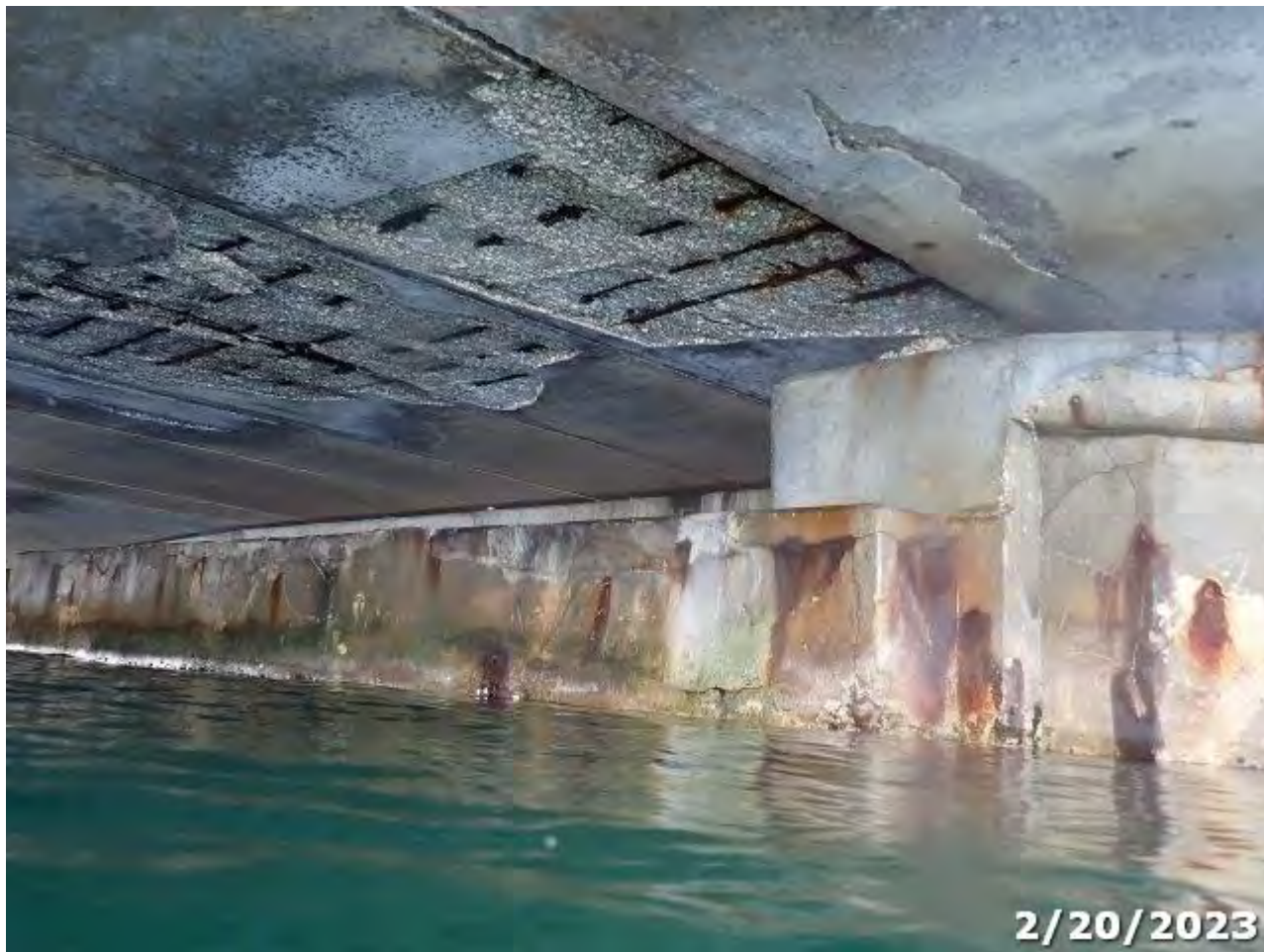
Photo 20 Element/Env 8393/4: Bulkhead Seawall Any Material
