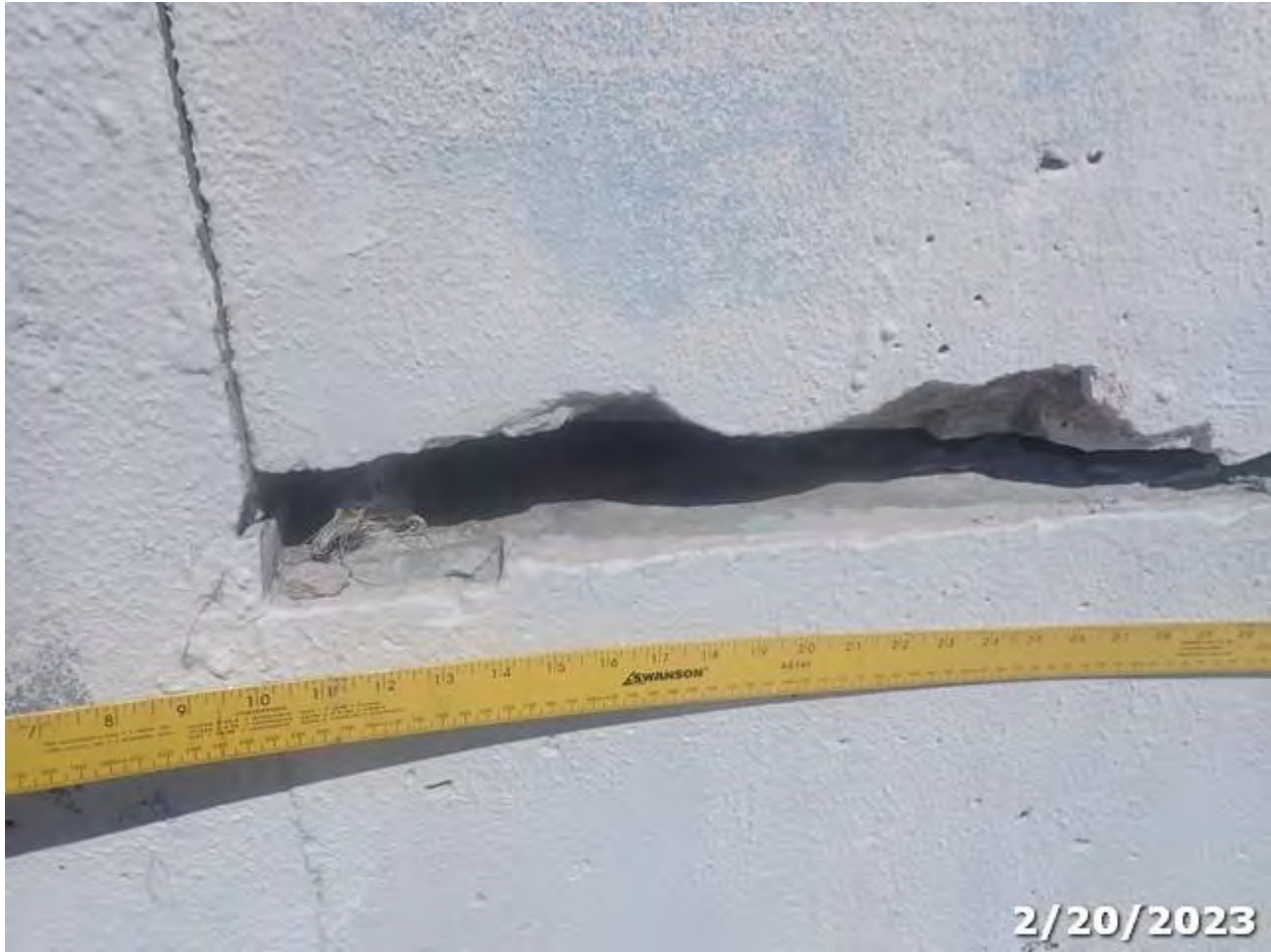
Photo 12 Element/Env 8475/4: R/Conc Walls
