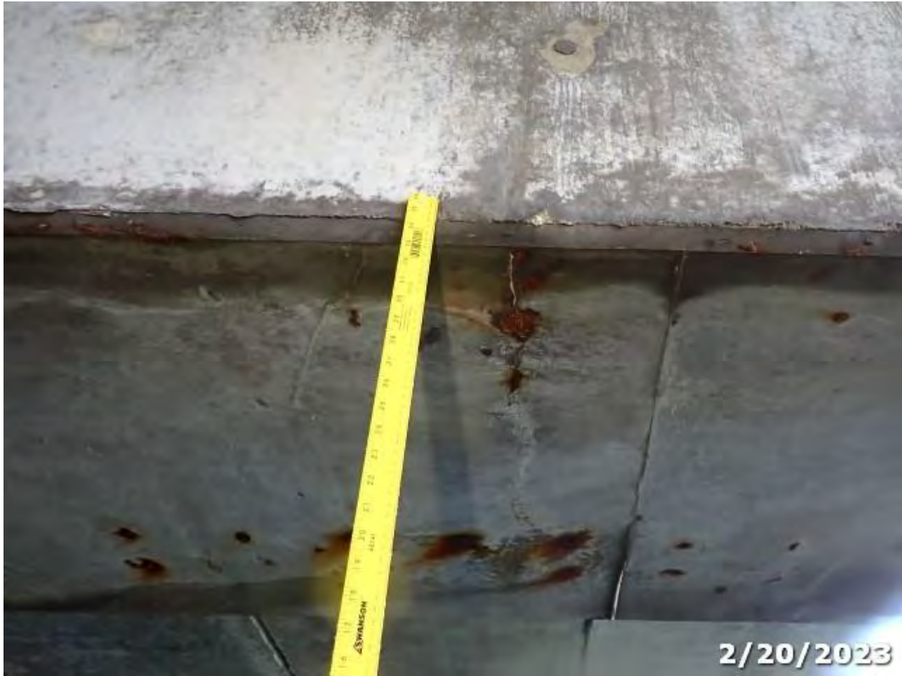
Photo 16 Element/Env 234/4: Re. Concrete Pier Cap
