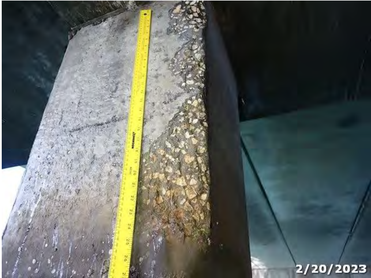
Photo 15 Element/Env 226/4: Pre. Concrete Pile
