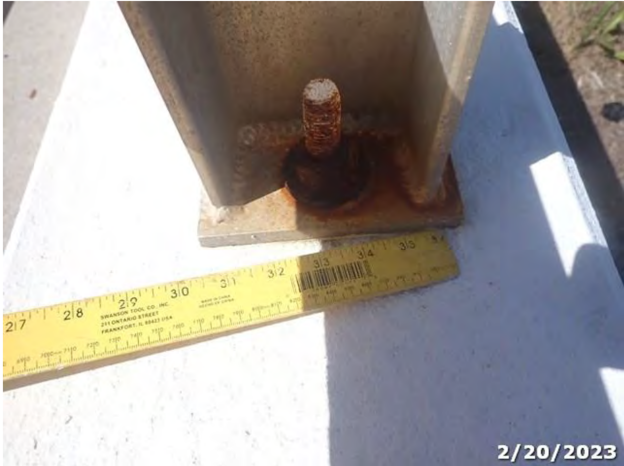
Photo 23 Element/Env 333/4: Other Bridge Railing
