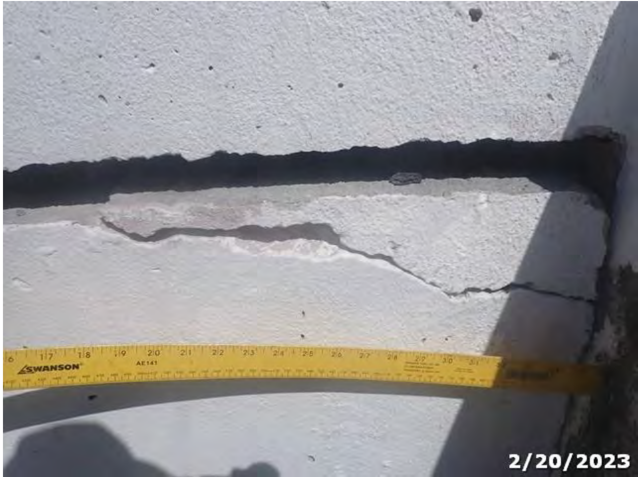
Photo 13 Element/Env 8475/4: R/Conc Walls
