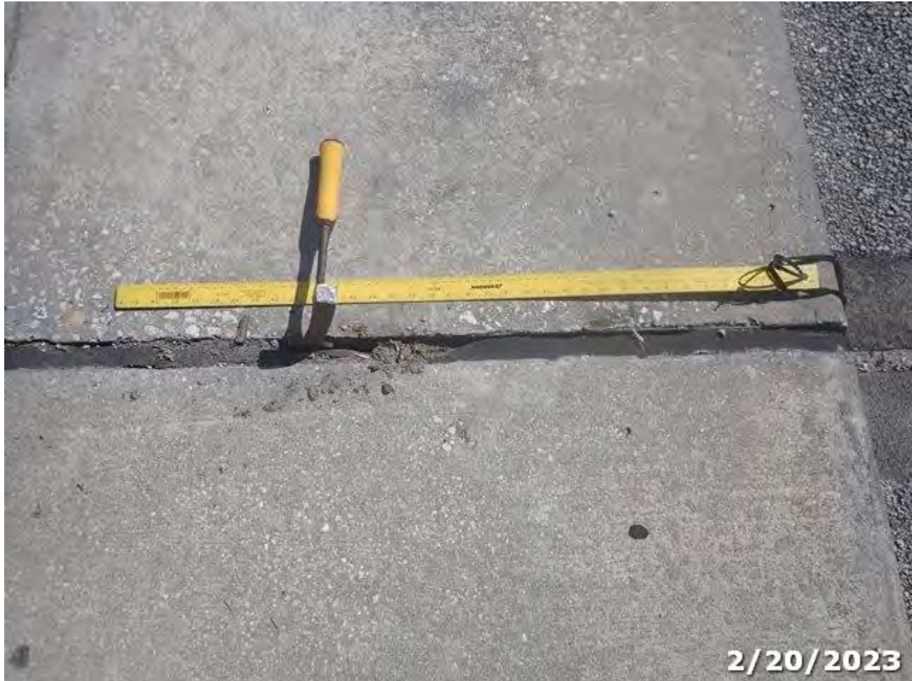
Photo 07 Element/Env 301/4: Pourable Joint Seal
