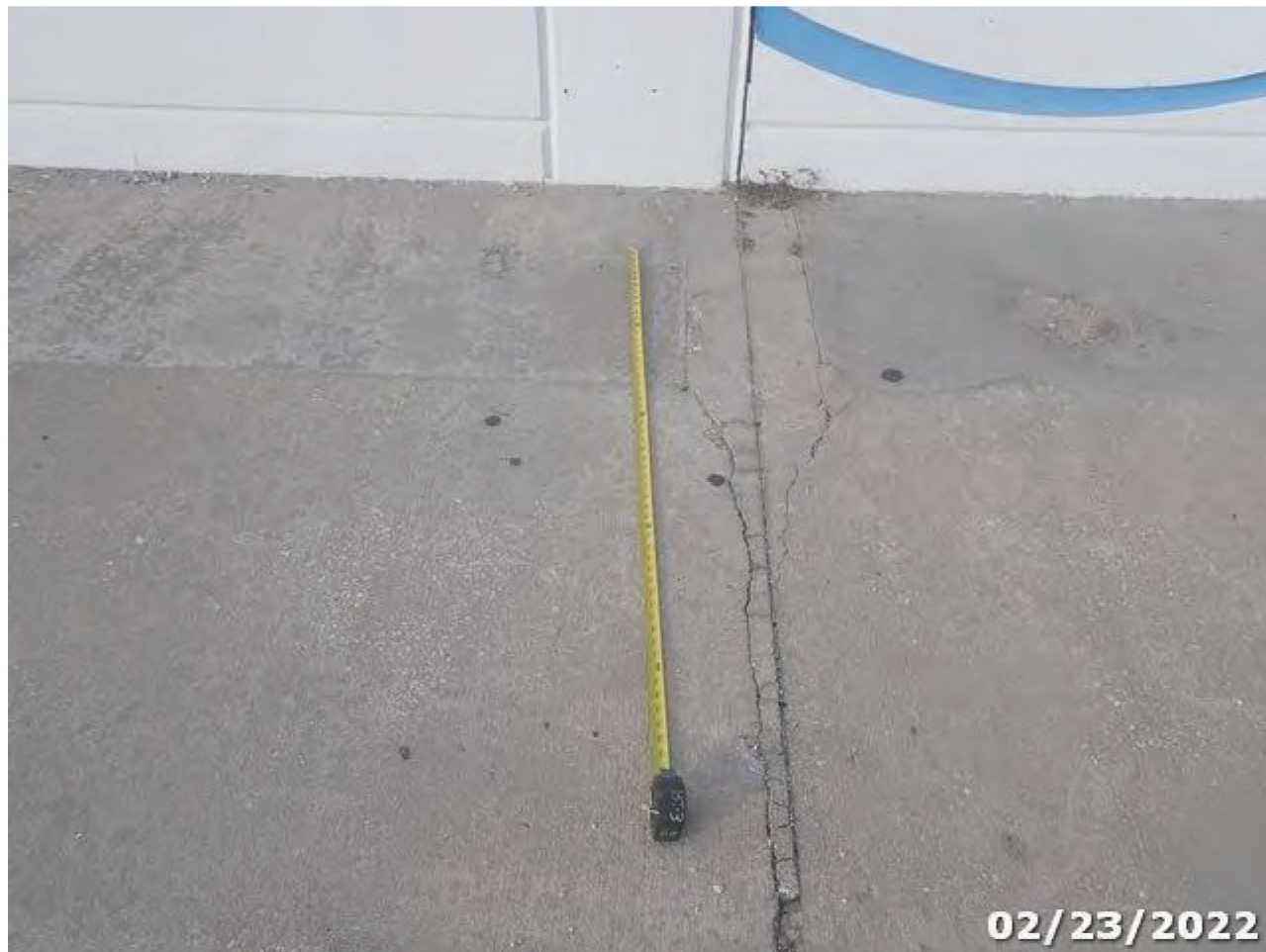
Photo 02 Element/Env 8099/4: PS Conc Slab (Sonovoid)
