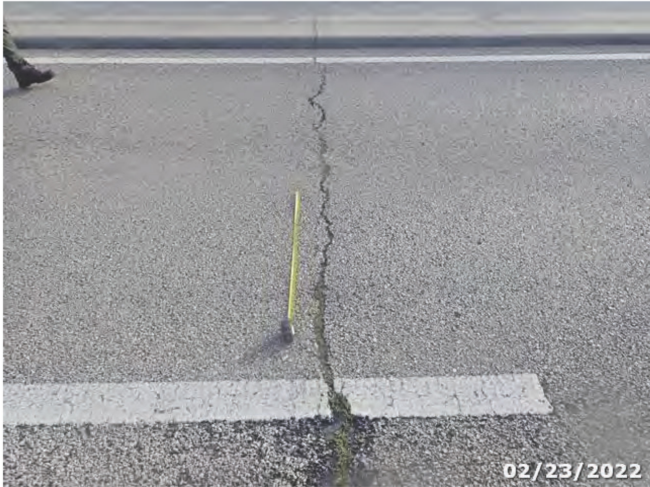
Photo 08 Element/Env 8099/510/4: PS Conc Slab (Sonovoid)/ Wearing Surfaces
