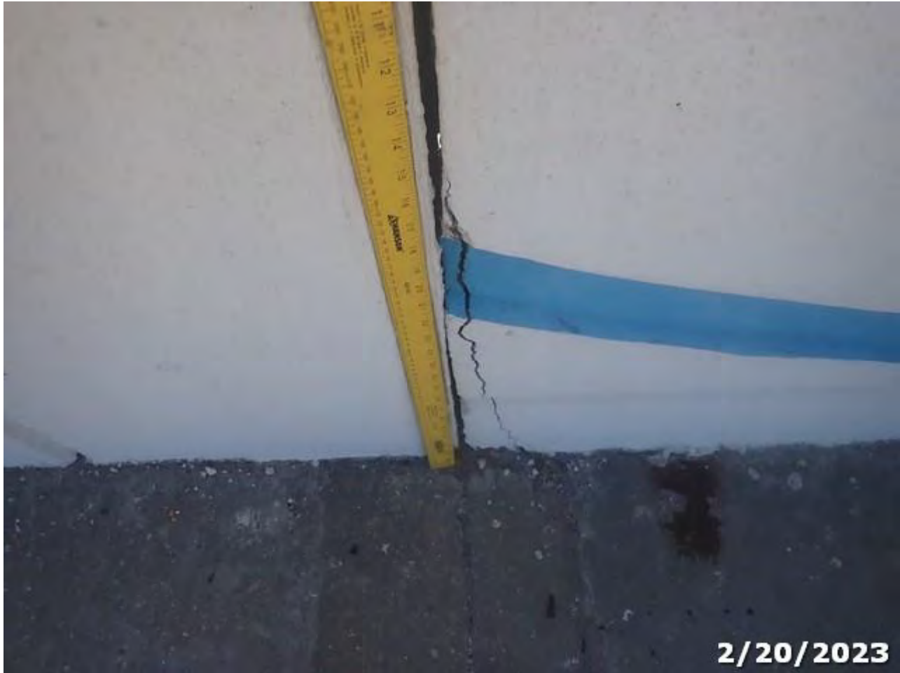
Photo 24 Element/Env 333/4: Other Bridge Railing
