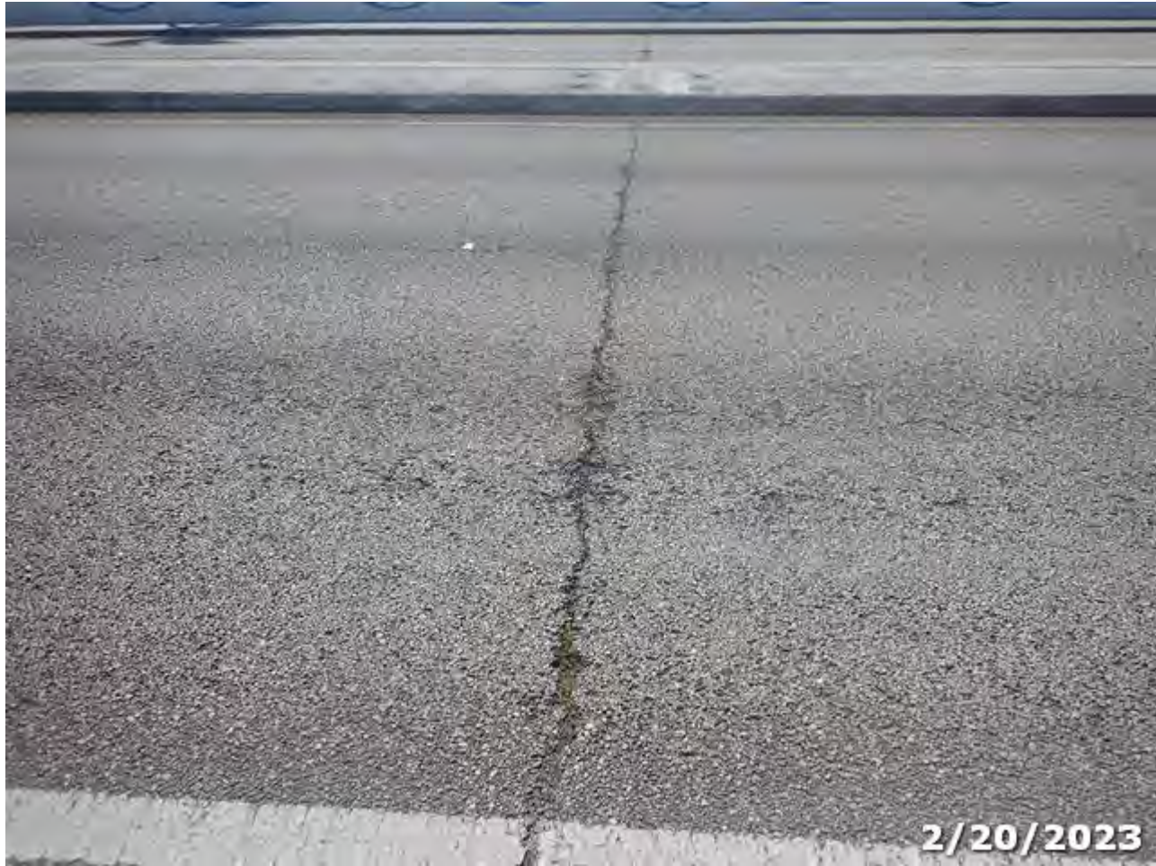
Photo 06 Element/Env 8099/510/4: PS Conc Slab (Sonovoid)/ Wearing Surfaces
