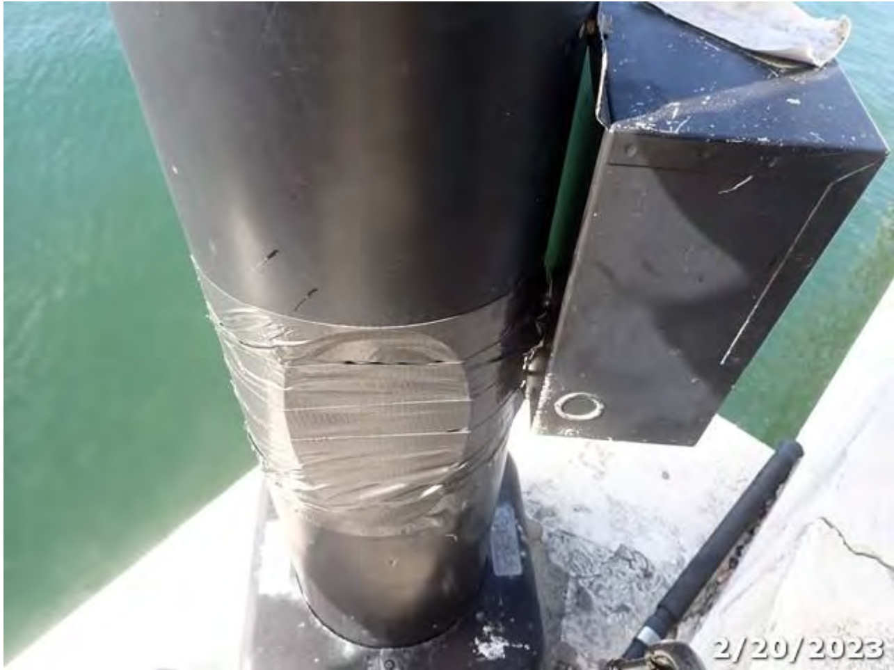
Photo 17 Element/Env 234/4: Re. Concrete Pier Cap
