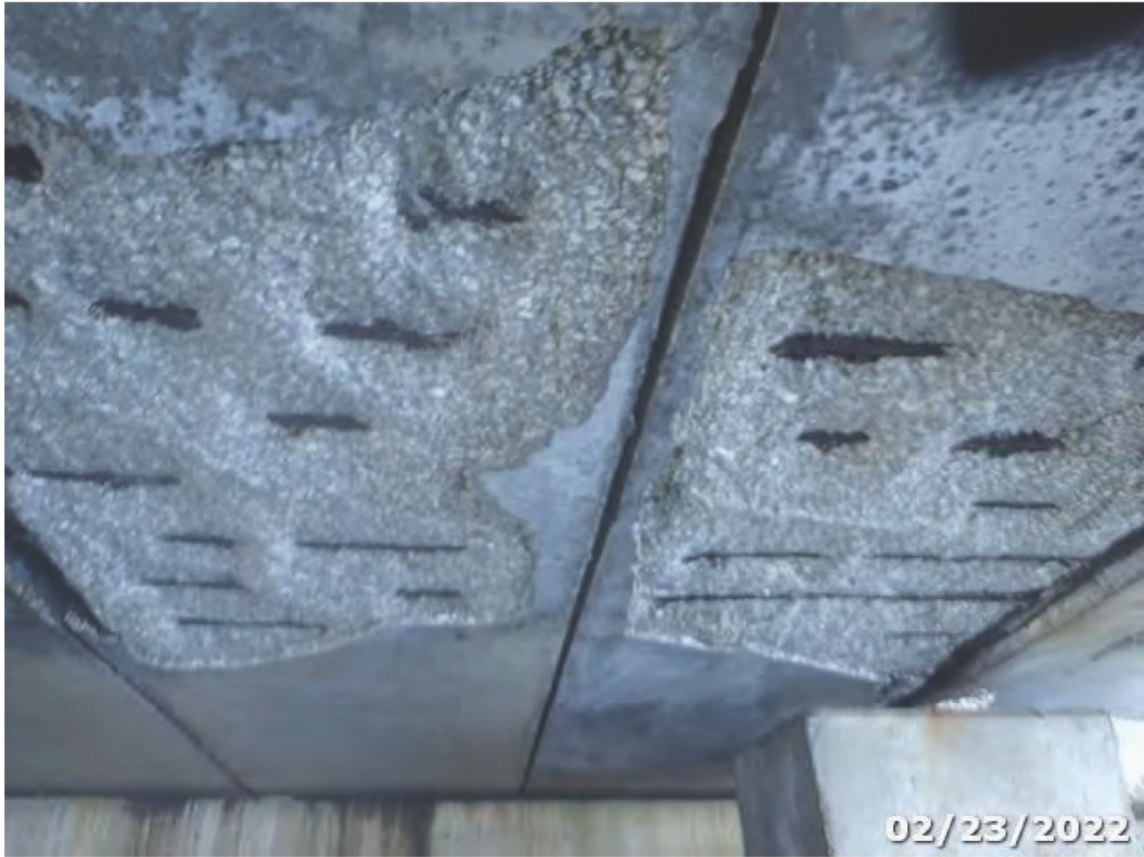
Photo 05 Element/Env 8099/4: PS Conc Slab (Sonovoid)
