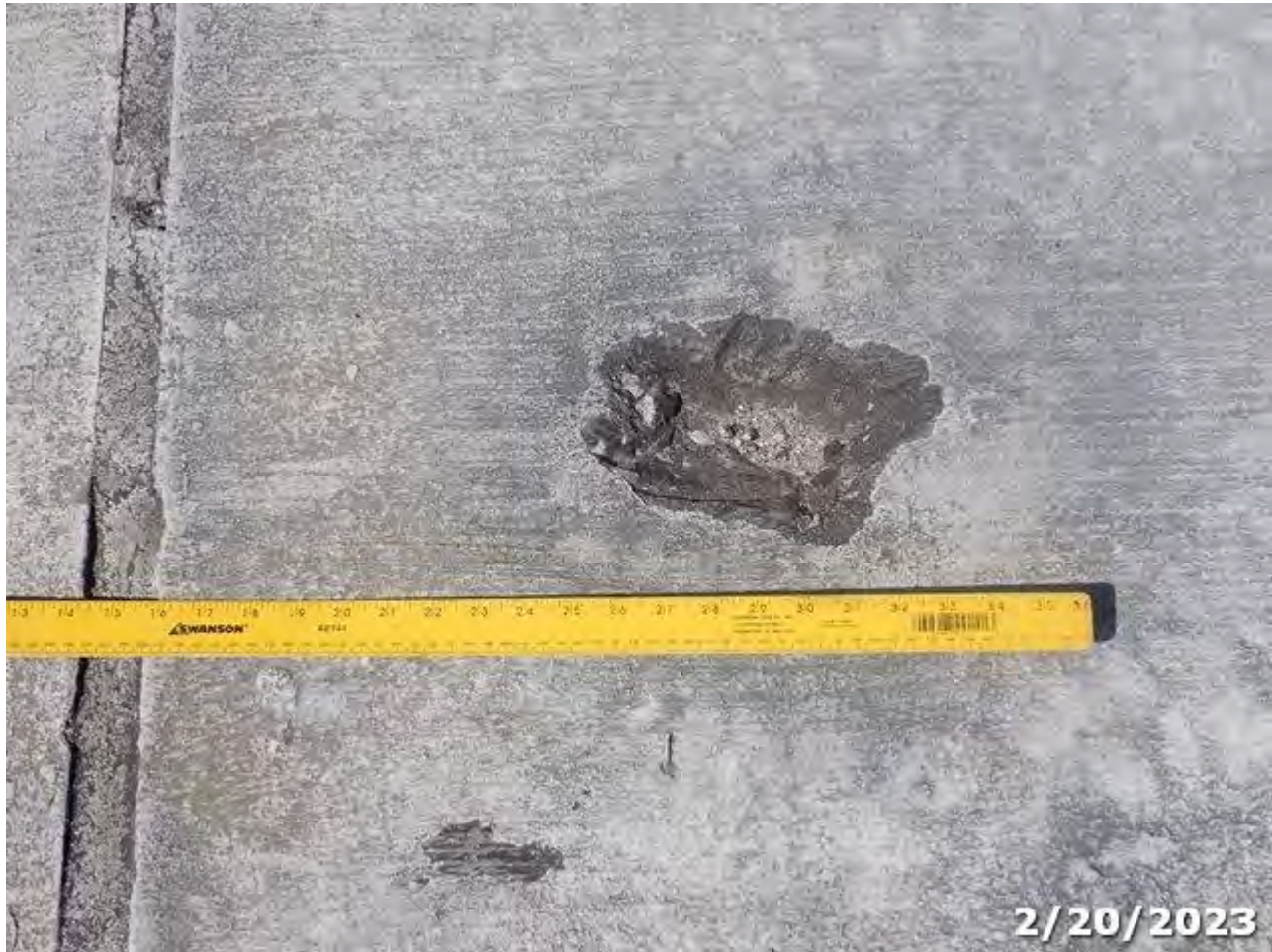
Photo 01 Element/Env 8099/4: PS Conc Slab (Sonovoid)
