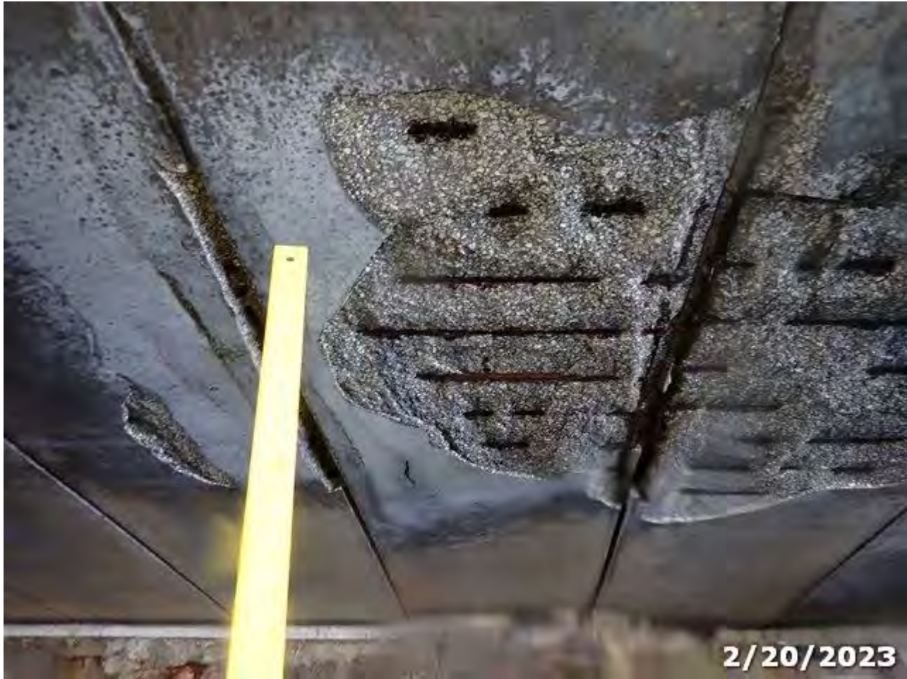
Photo 04 Element/Env 8099/4: PS Conc Slab (Sonovoid)
