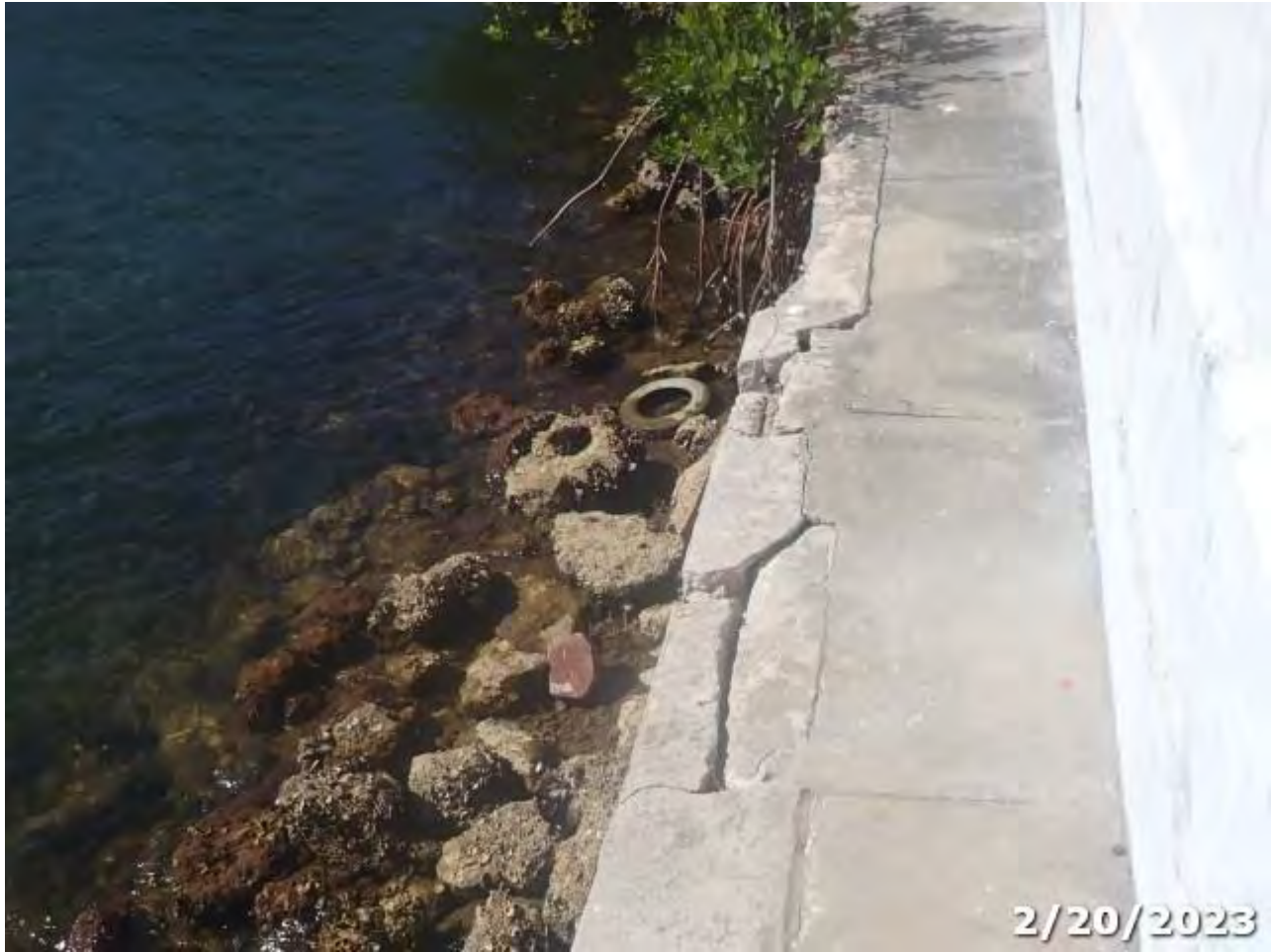
Photo 18 Element/Env 8393/4: Bulkhead Seawall Any Material
