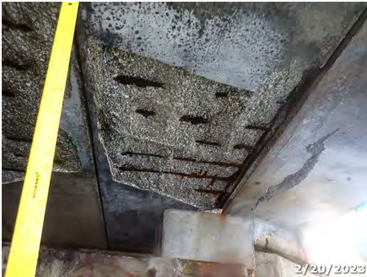
Photo 03 Element/Env 8099/4: PS Conc Slab (Sonovoid)
