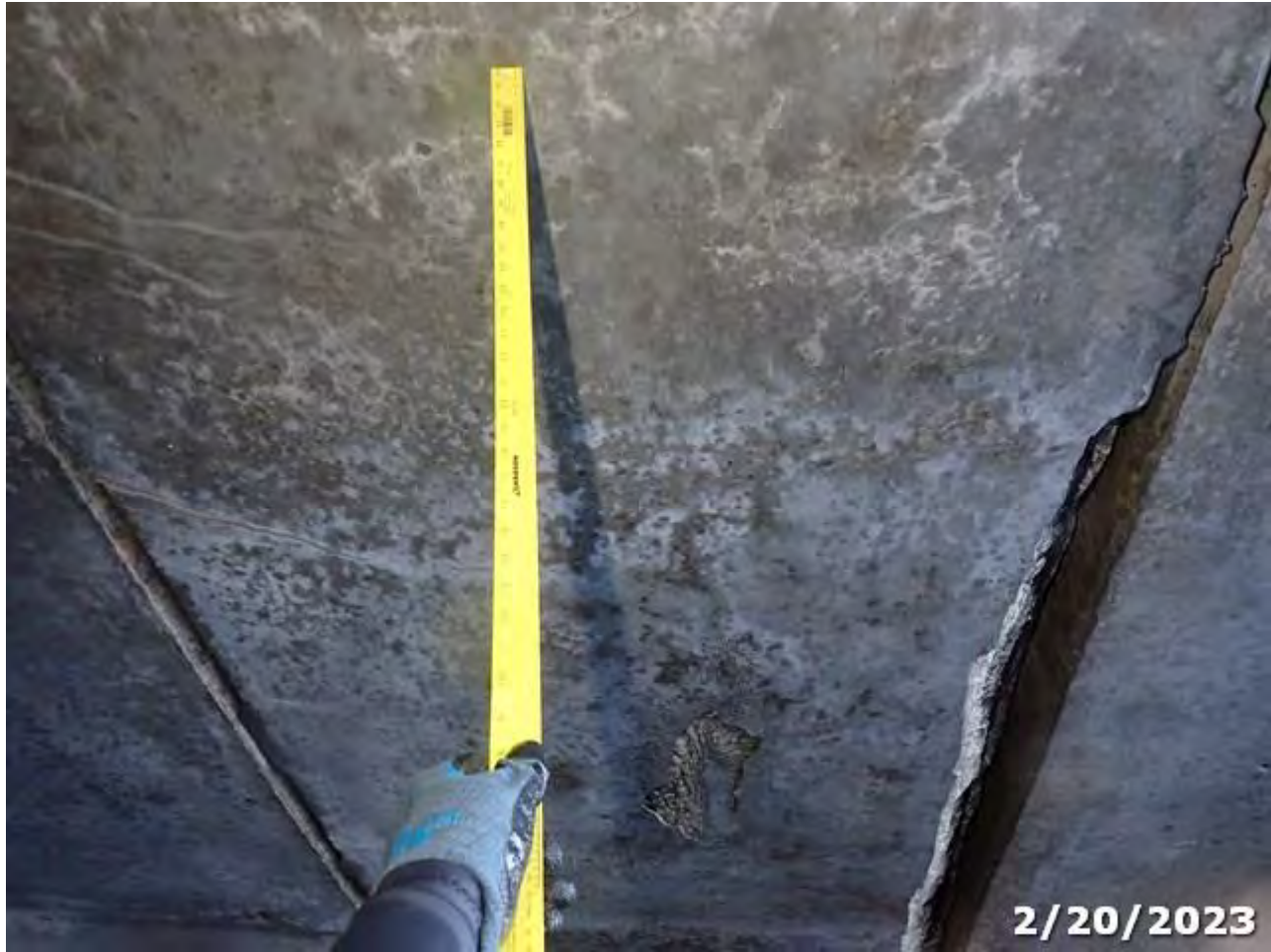
Photo 05 Element/Env 8099/4: PS Conc Slab (Sonovoid)
