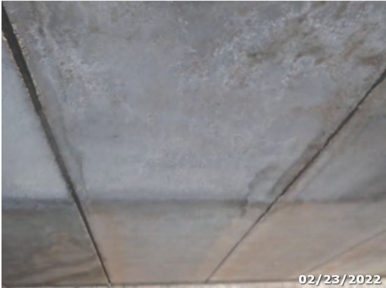
Photo 04 Element/Env 8099/4: PS Conc Slab (Sonovoid)
