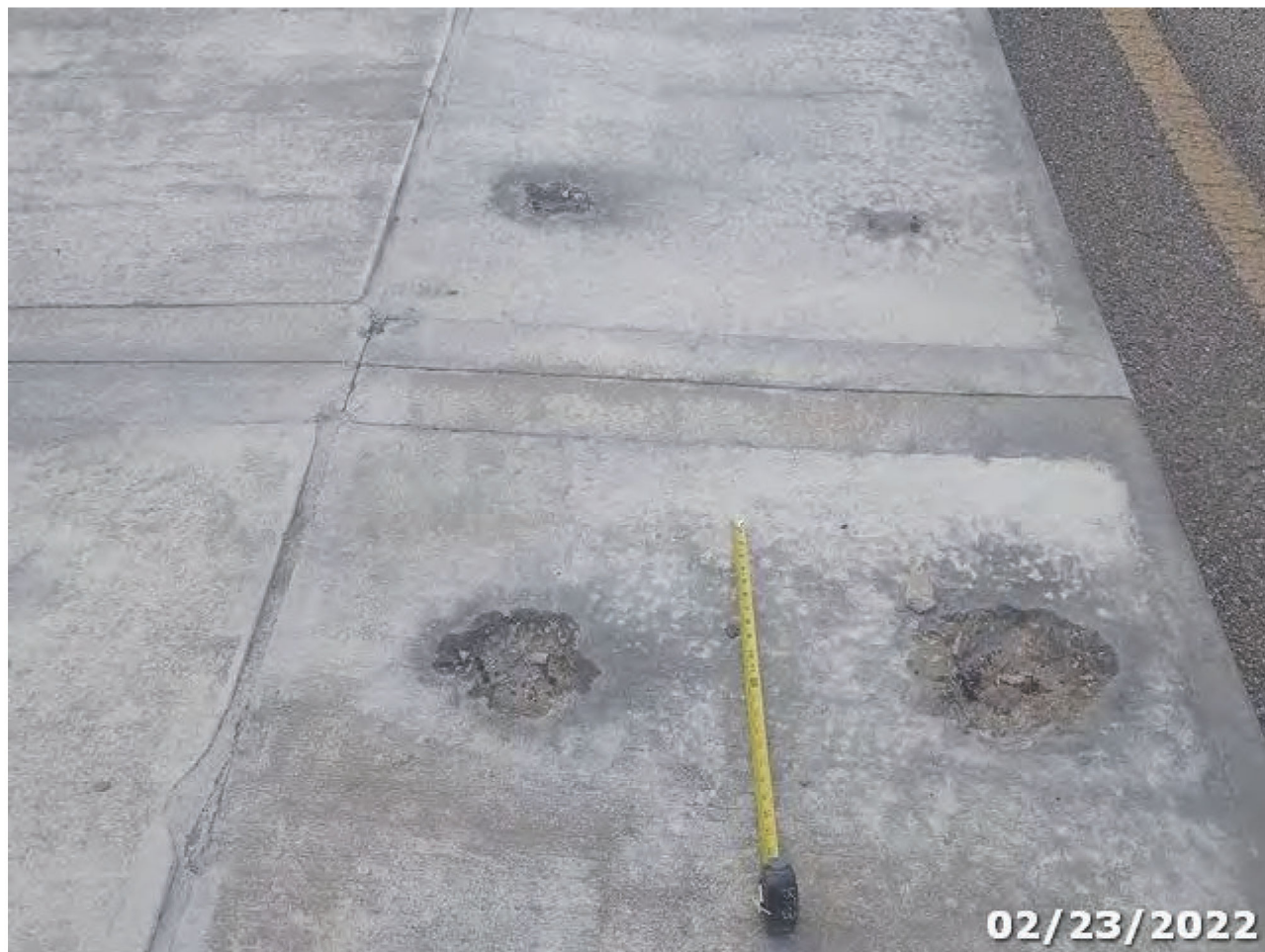
Photo 01 Element/Env 8099/4: PS Conc Slab (Sonovoid)
