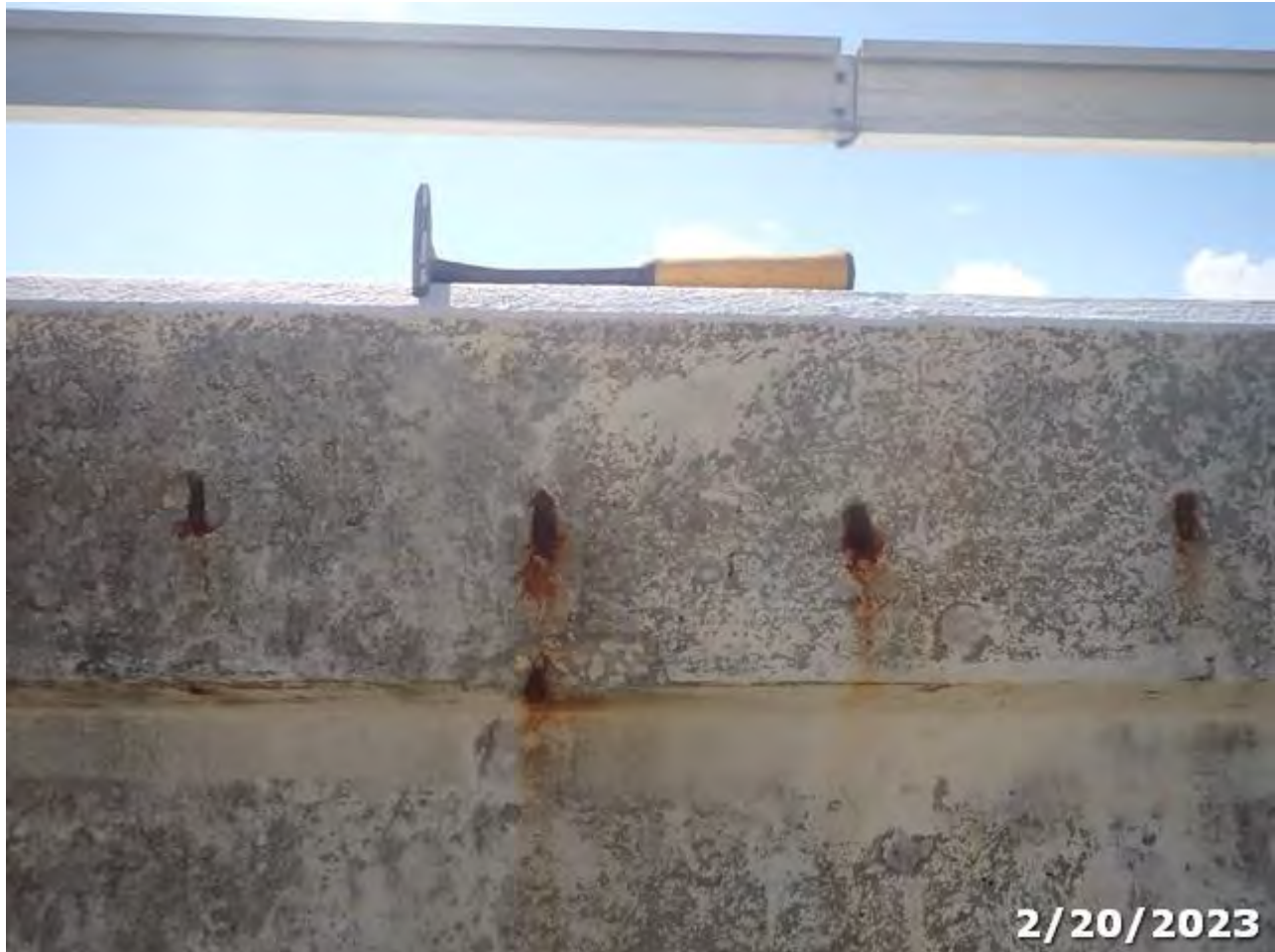
Photo 14 Element/Env 8475/4: R/Conc Walls
