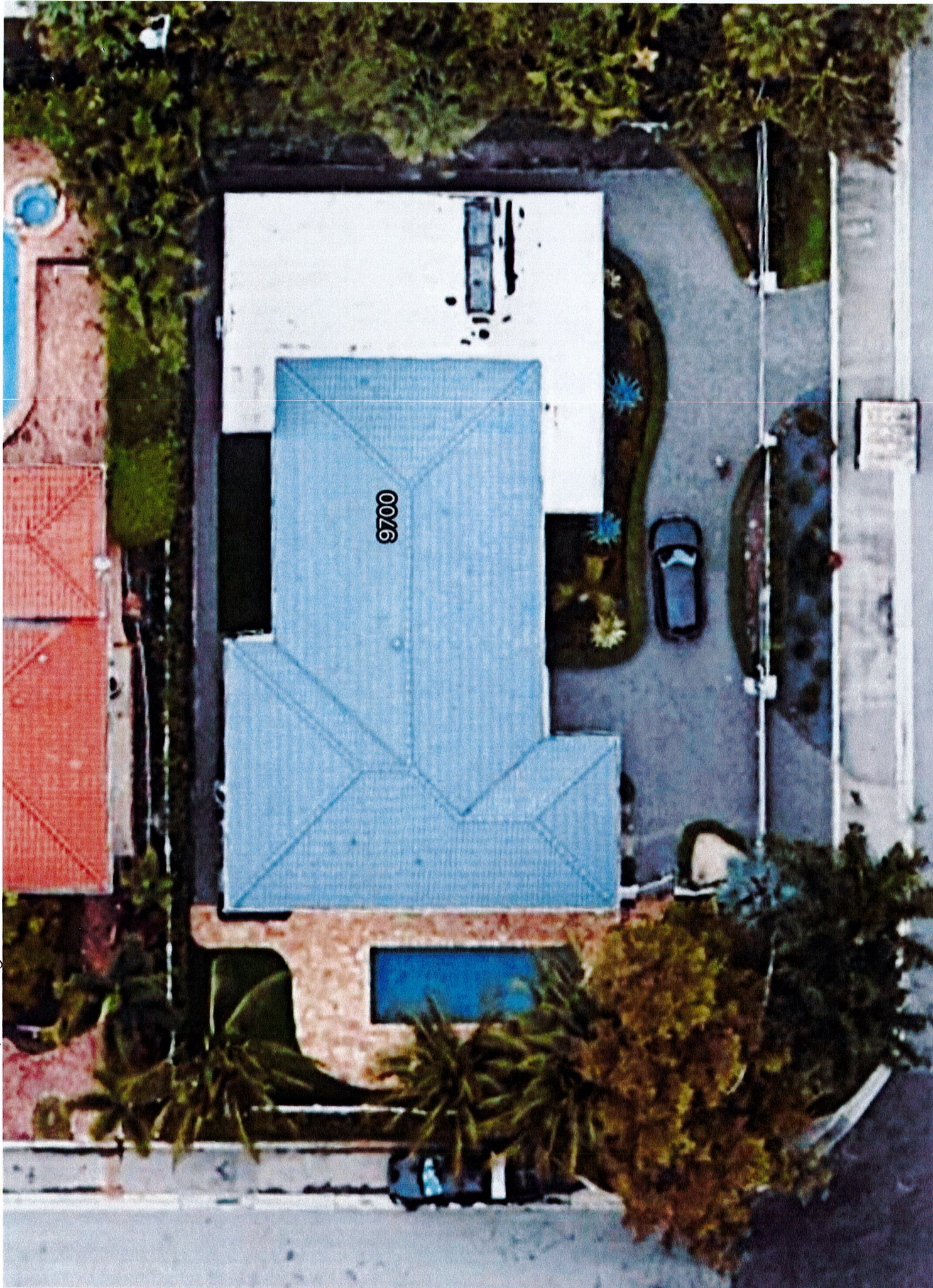
before (existing) 9700 E Broadview Dr, Bay Harbor Islands FL 33154
