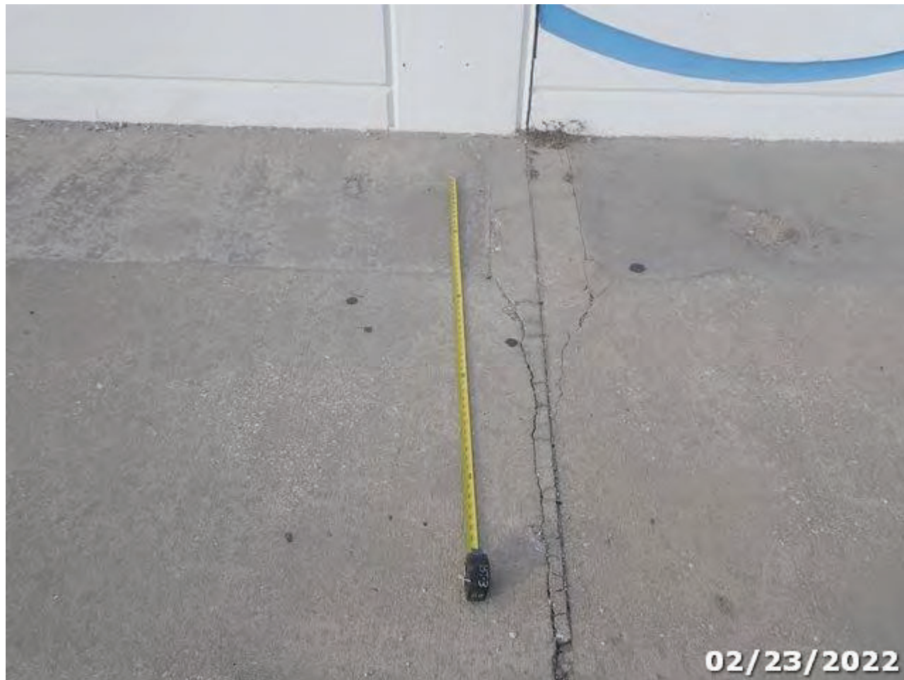
Photo 02 Element/Env 8099/4: PS Conc Slab (Sonovoid)
