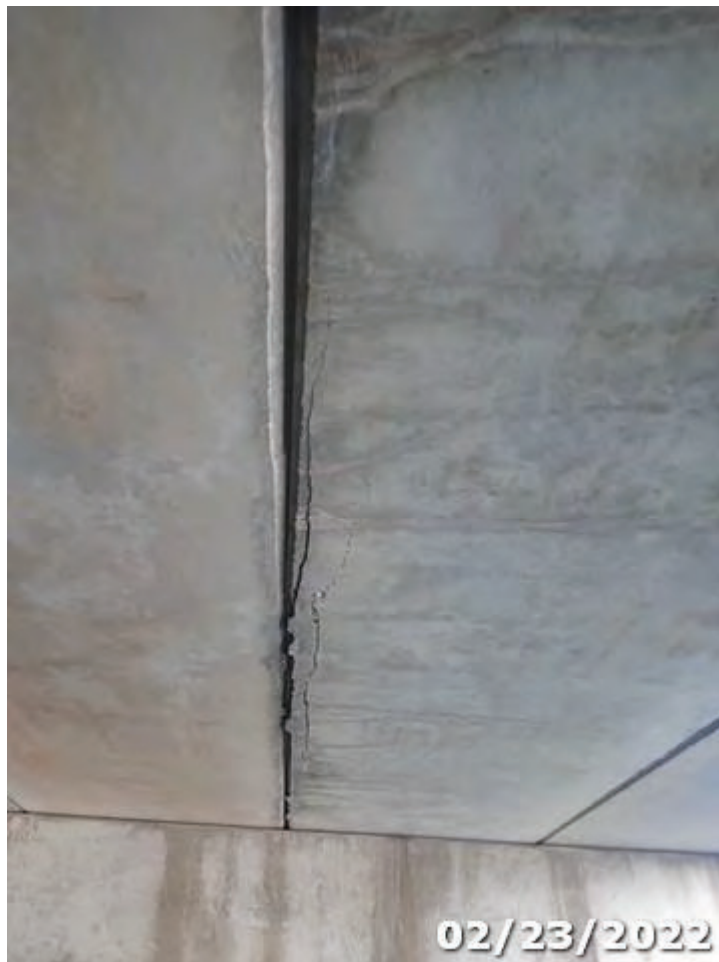
Photo 03 Element/Env 8099/4: PS Conc Slab (Sonovoid)
