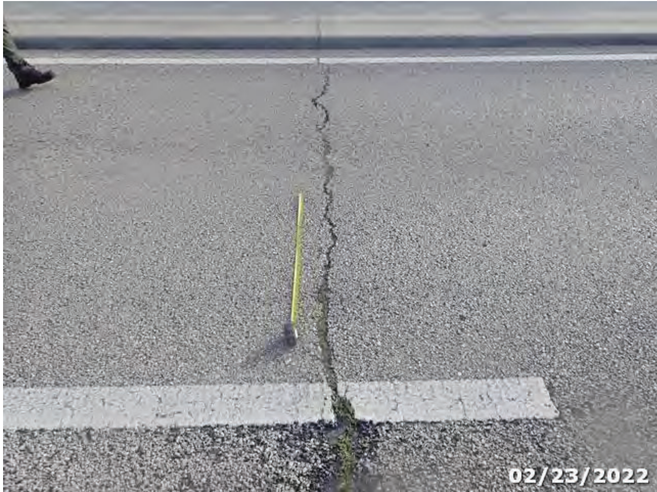
Photo 08 Element/Env 8099/510/4: PS Conc Slab (Sonovoid)/ Wearing Surfaces
