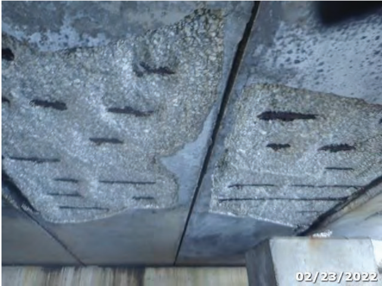
Photo 05 Element/Env 8099/4: PS Conc Slab (Sonovoid)
