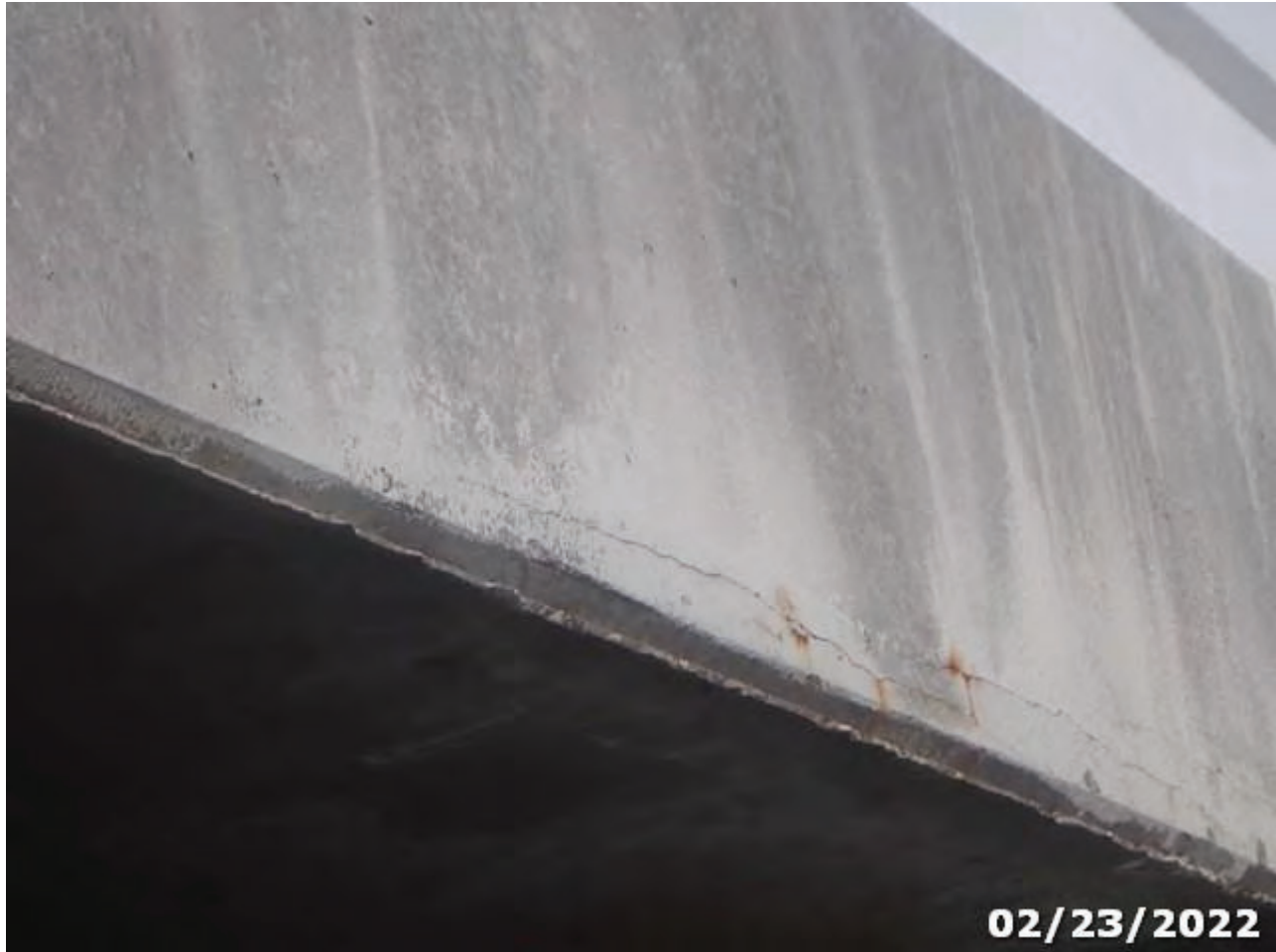
Photo 07 Element/Env 8099/4: PS Conc Slab (Sonovoid)
