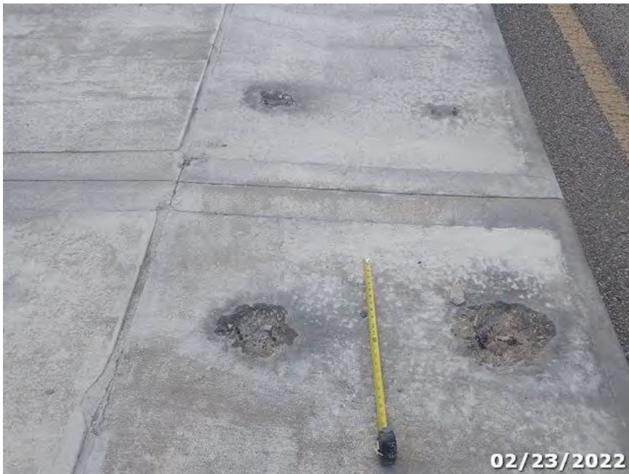
Photo 01 Element/Env 8099/4: PS Conc Slab (Sonovoid)
