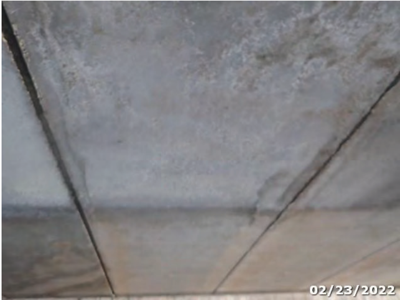
Photo 04 Element/Env 8099/4: PS Conc Slab (Sonovoid)
