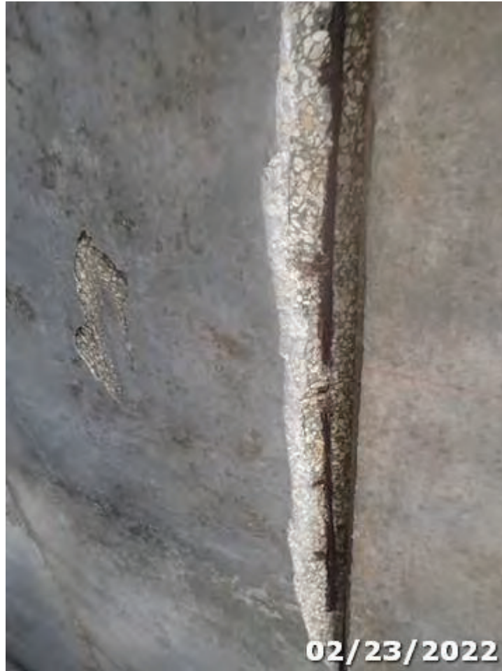
Photo 06 Element/Env 8099/4: PS Conc Slab (Sonovoid)
