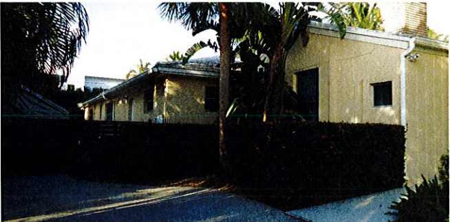
EXISTING PROPERTY WEST VIEW
