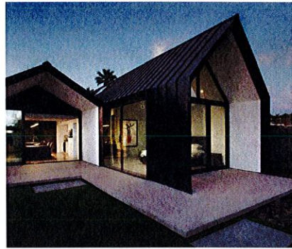
METAL ROOF AND CLADDING
