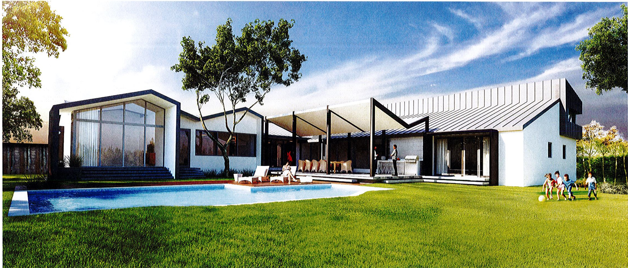
REAR VIEW - NORTH
