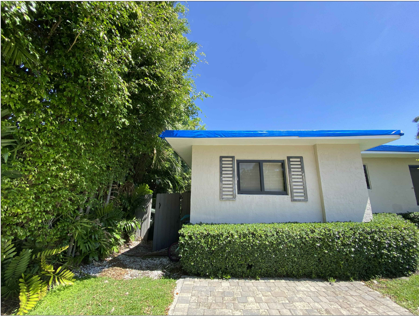
FRONT/SOUTH PARTIAL VIEW
