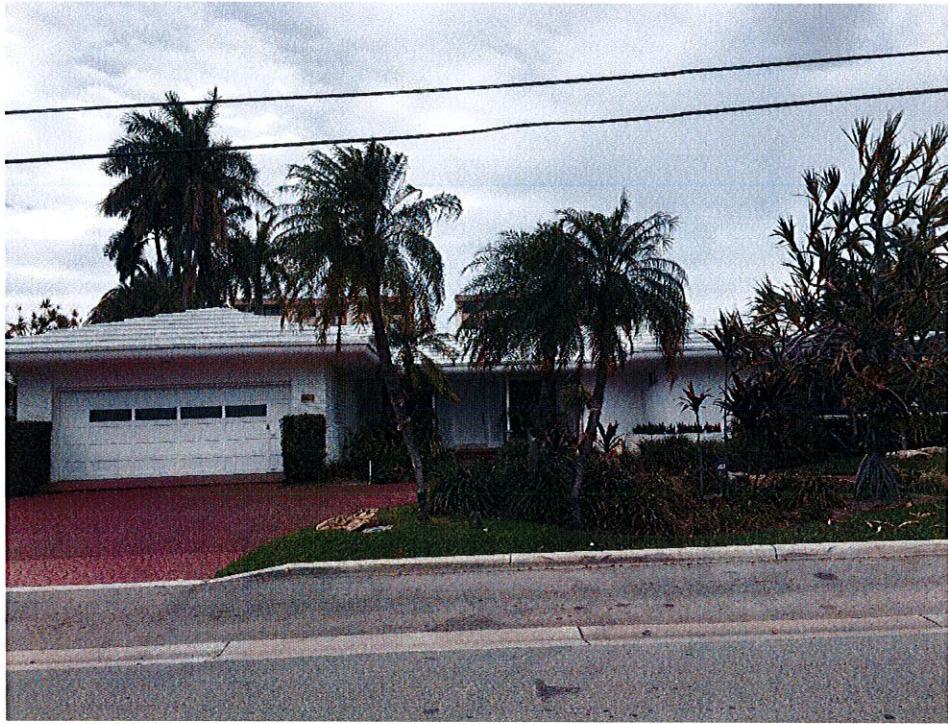
FRONT OF THE EXISTING SITE
