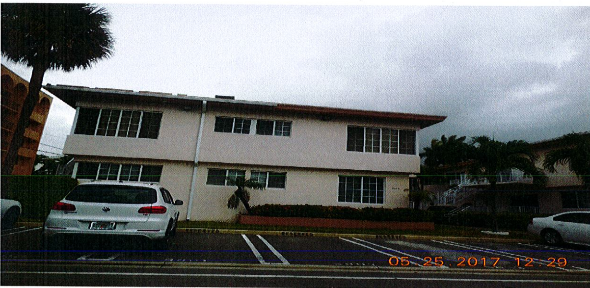
Building 9260- No violations observed.
