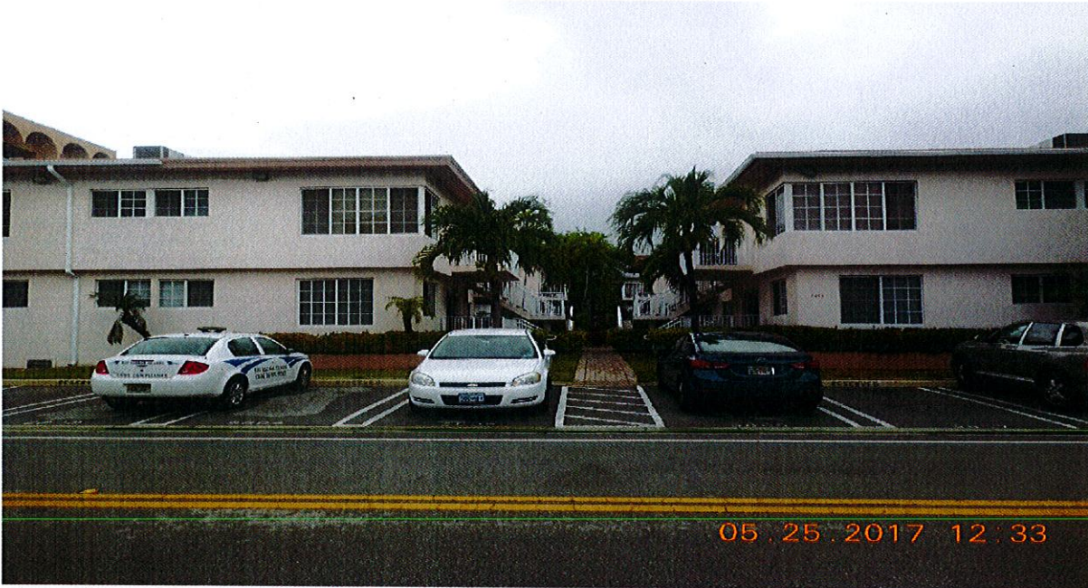
Front view of the property. No violations observed.
