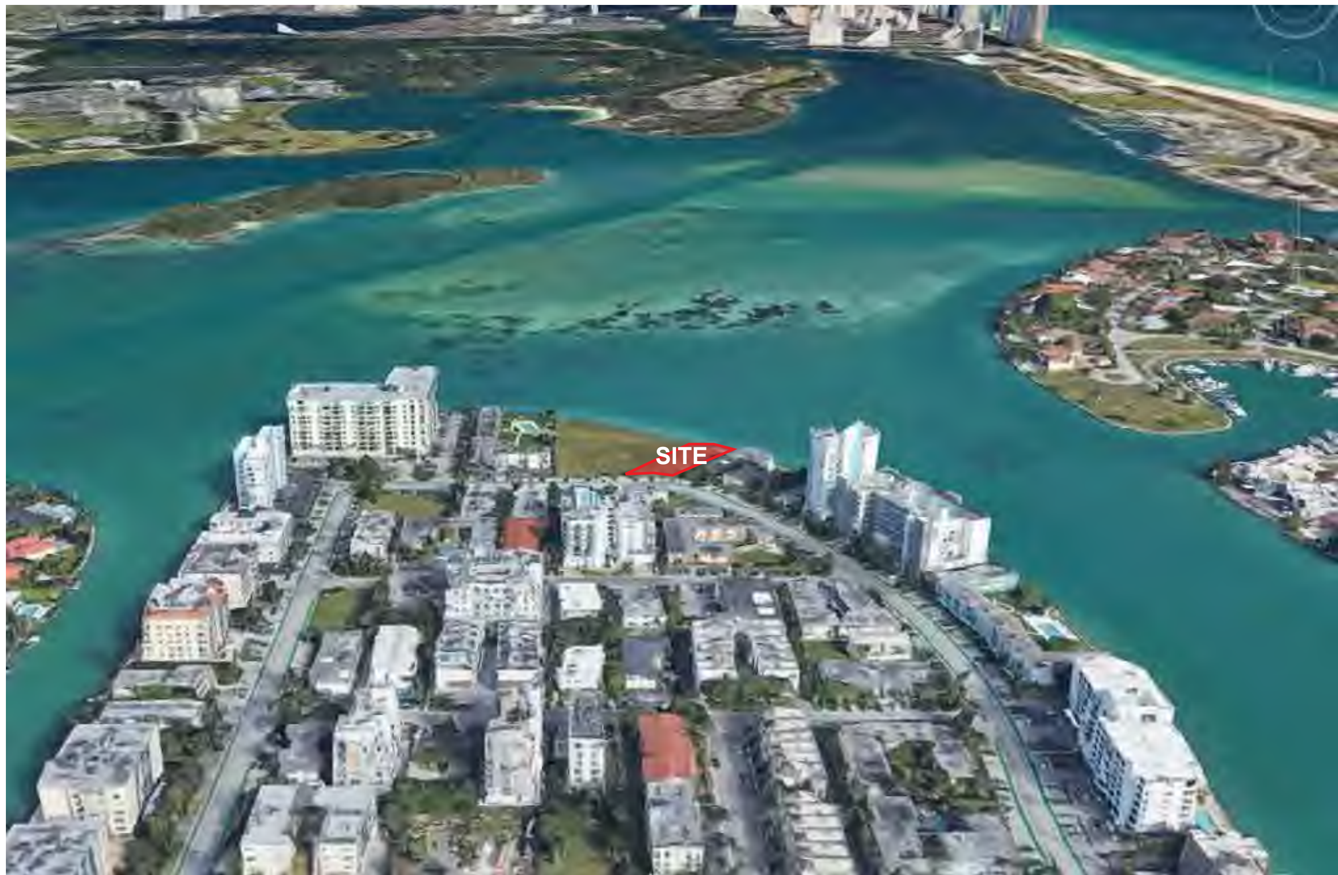
VIEW 02 - LOOKING NORTH
