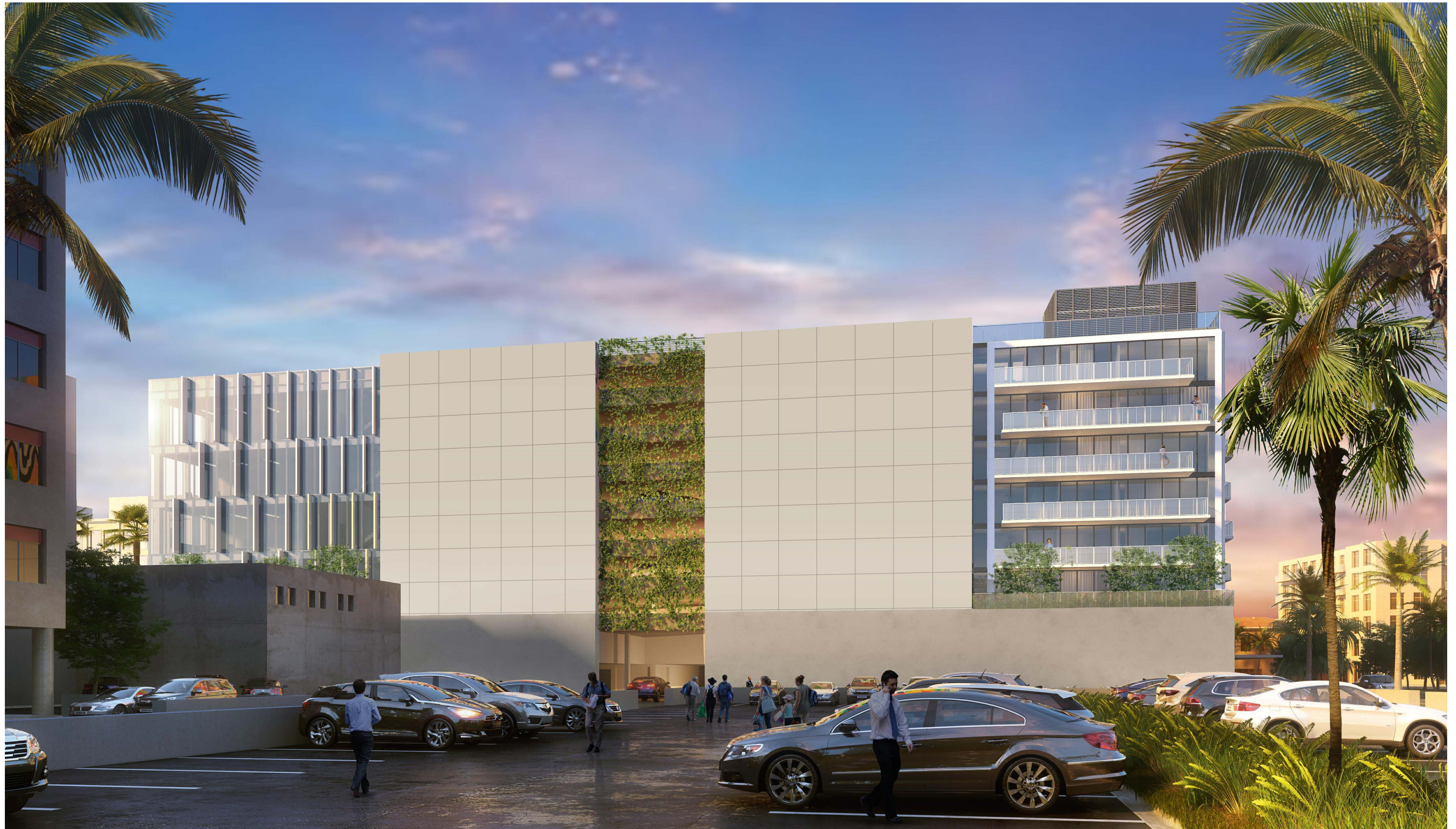
EAST FACADE FROM PARKING LOT
