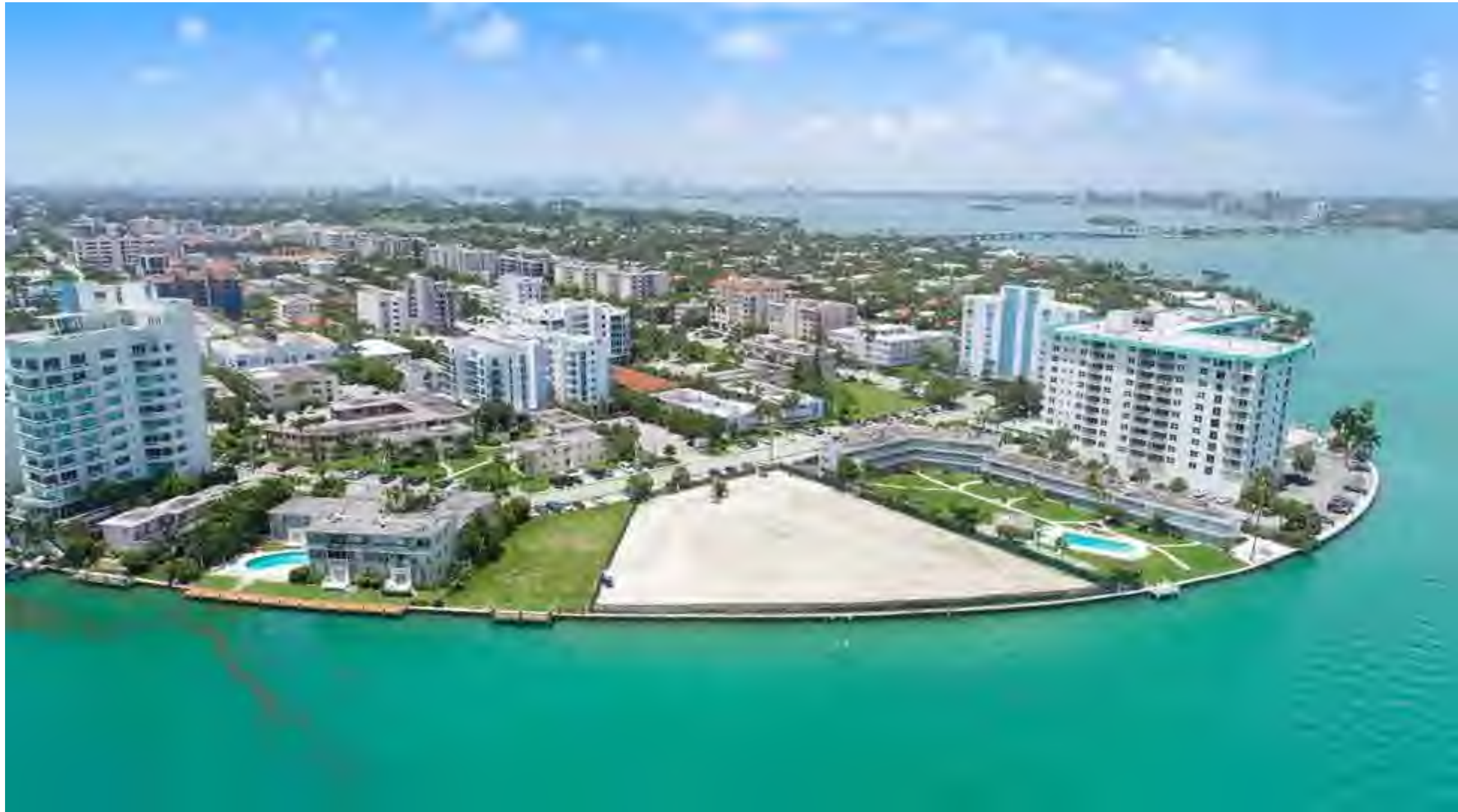
SITE VIEW 03 - FROM NORTHWEST (BISCAYNE BAY)
