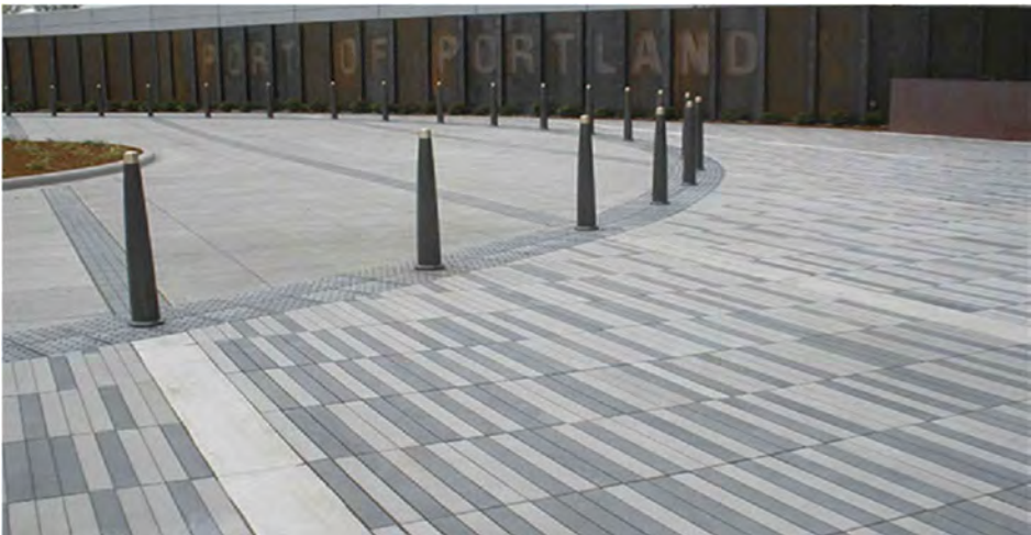
CONCRETE PAVER DRIVEWAYS
