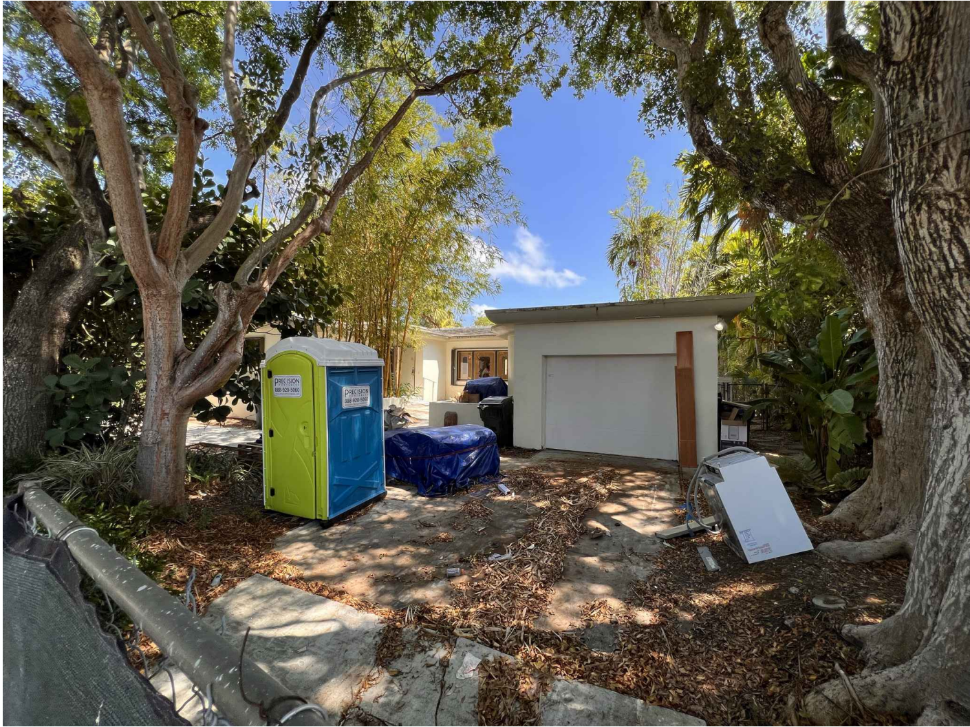
PIC: 3 VIEW: NEIGH- BOR EAST ADDRESS: 1260 99th ST.
