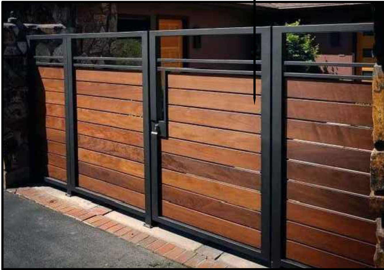
4'-0" HIGH SELF CLOSING BLACK ALUMINUM ENTRY GATE WITH IPE WD. SLAT INFILL. SHALL SWING OUTWARD AWAY FROM POOL W/ SELF LATCHING DEVICE MIN. 54" A.F.F.
