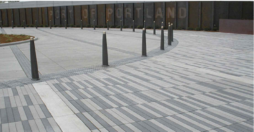
CONCRETE PAVER DRIVEWAYS
