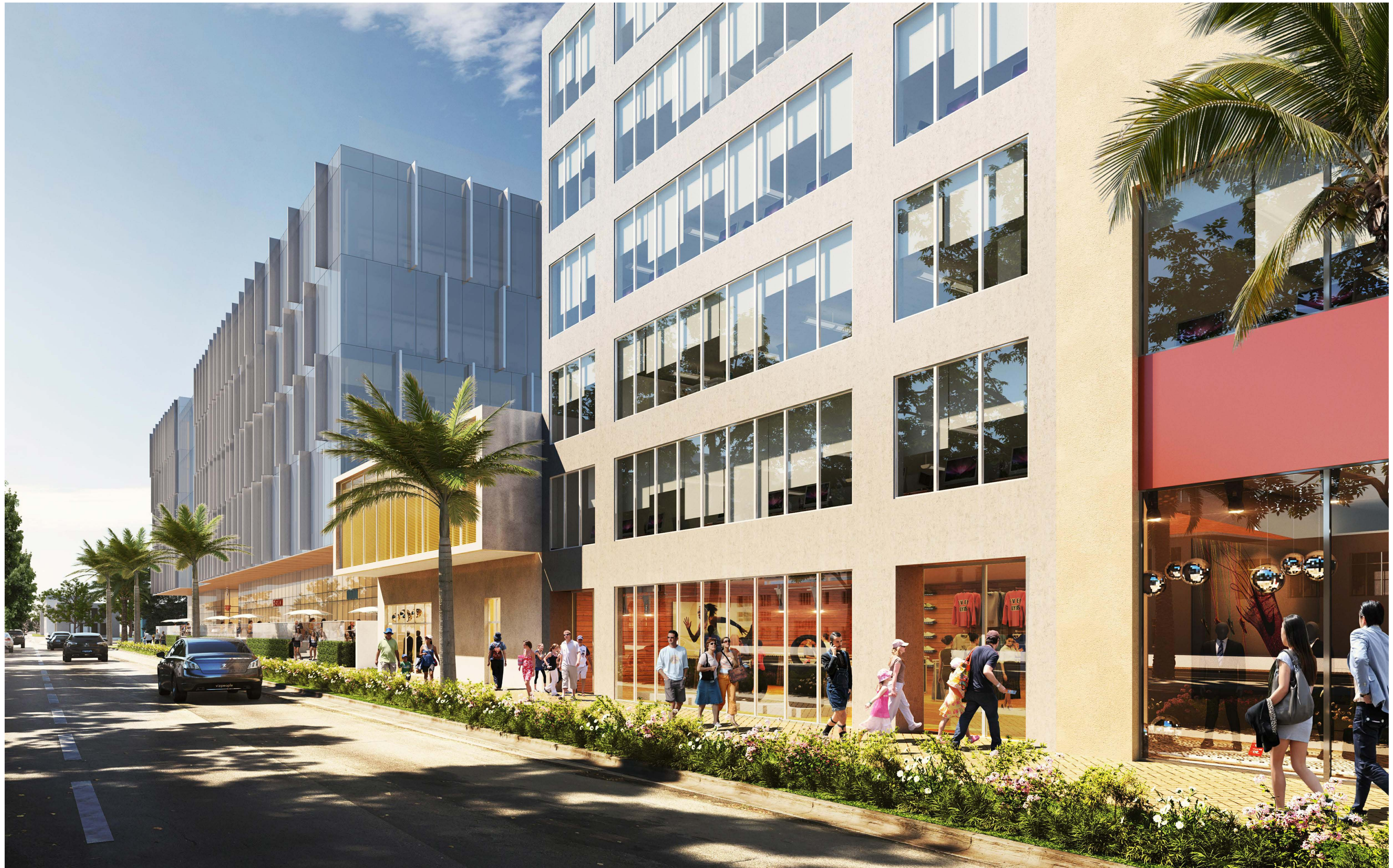
EAST FACADE FROM KANE CONCOURSE
