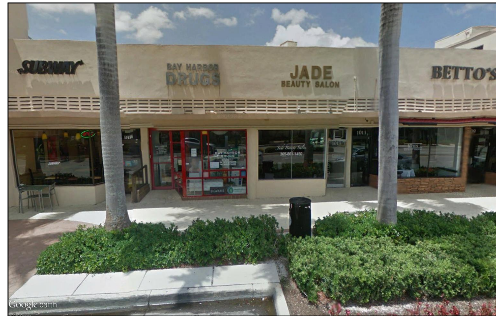
OFFICE, BUSINESS DISTRICT FLUM: COMMERCIAL 1 STORY
