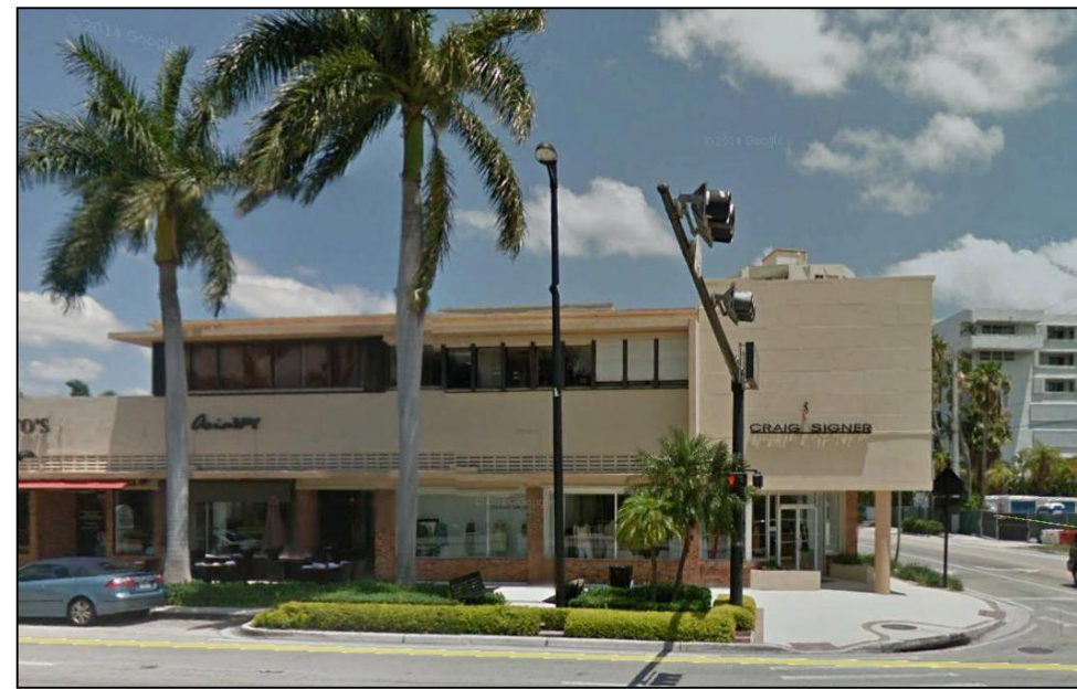
OFFICE, BUSINESS DISTRICT FLUM: COMMERCIAL 1 STORY
