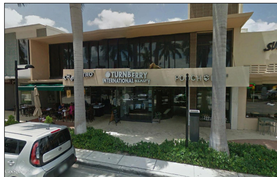
OFFICE, BUSINESS DISTRICT FLUM: COMMERCIAL 1 STORY
