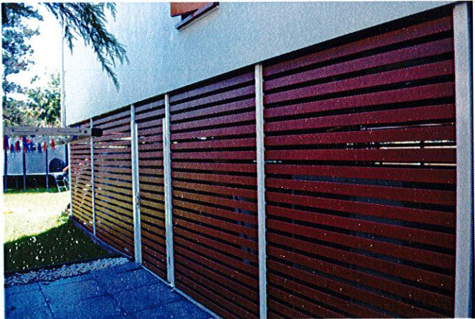
MECHANICAL SCREENING (AT GENERATOR & GARAGE GATES & AT GARAGE)
