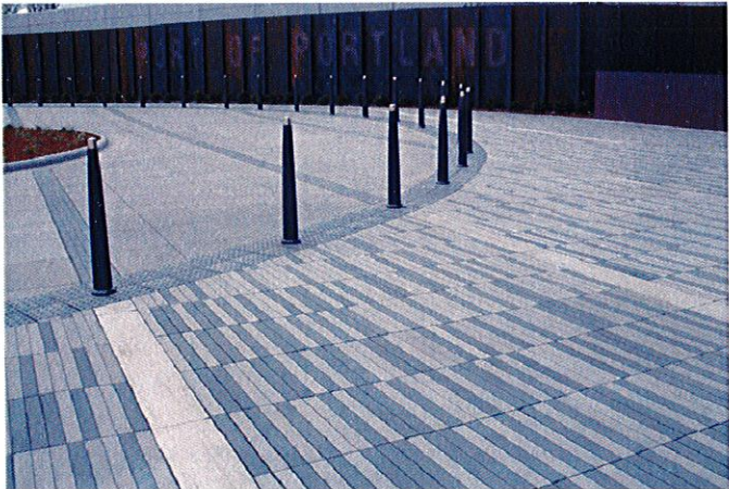
CONCRETE PAVER DRIVEWAYS
