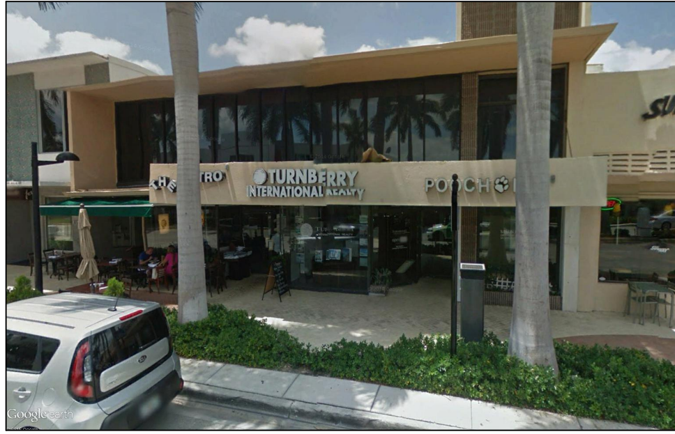
OFFICE, BUSINESS DISTRICT FLUM: COMMERCIAL 1 STORY
