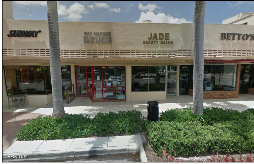
OFFICE, BUSINESS DISTRICT FLUM: COMMERCIAL 1 STORY
