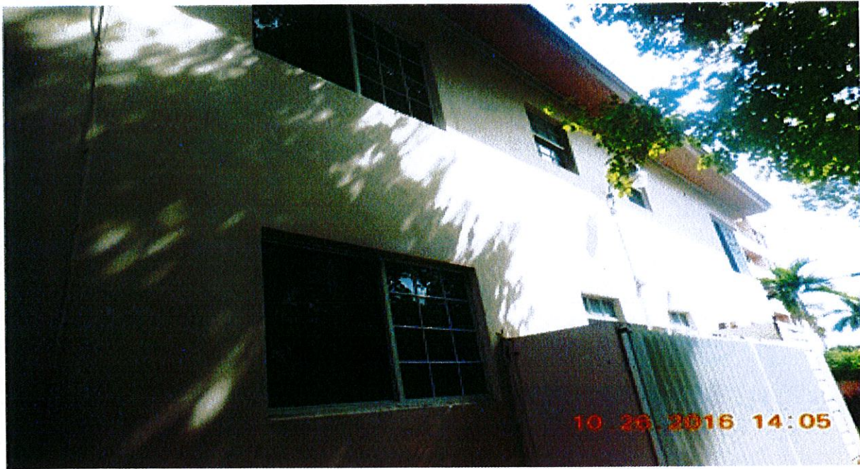
9260 rear view- No violations observed.
