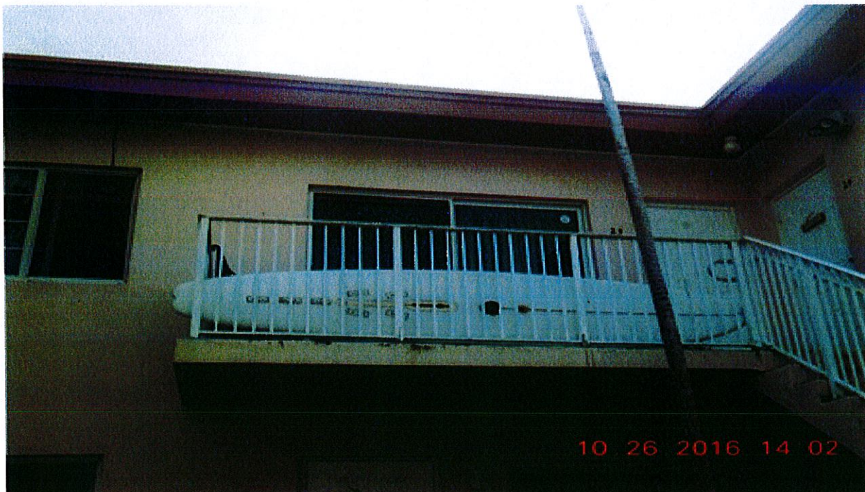
Unit # 23- No violations observed. (6 of 16 units)
