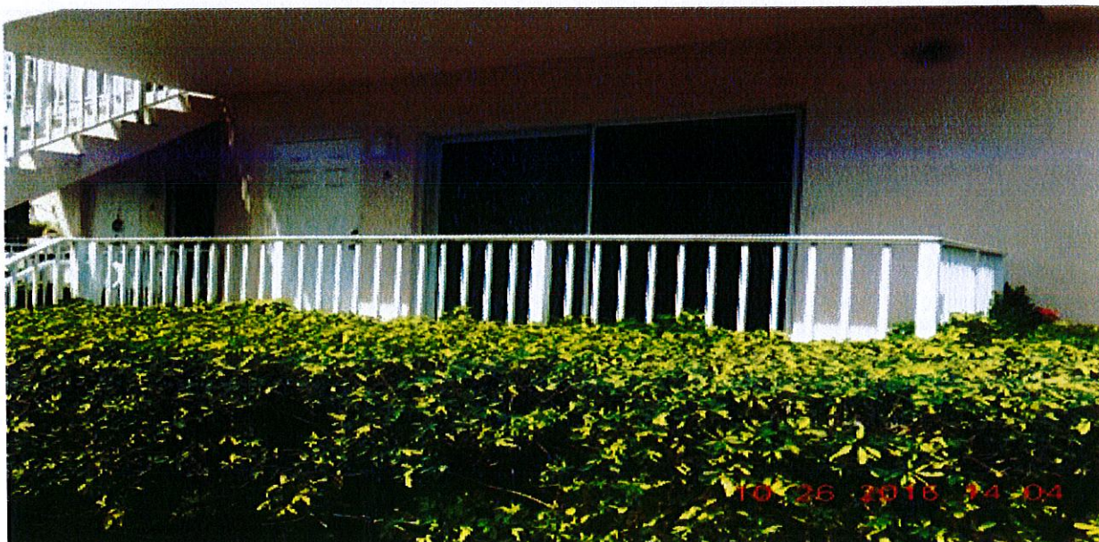
Unit # 5- No violations observed. (9 of 16 units)
