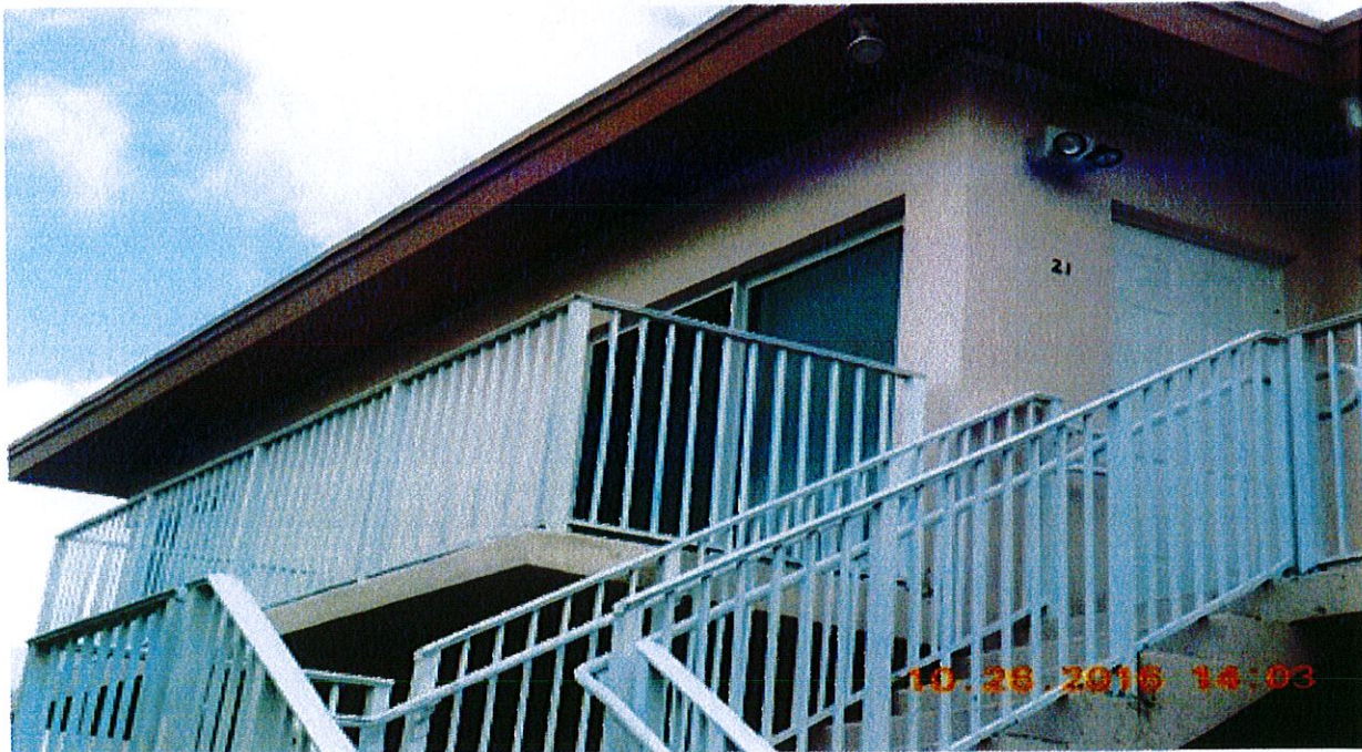
Unit # 21- No violations observed. (8 of 16 units)
