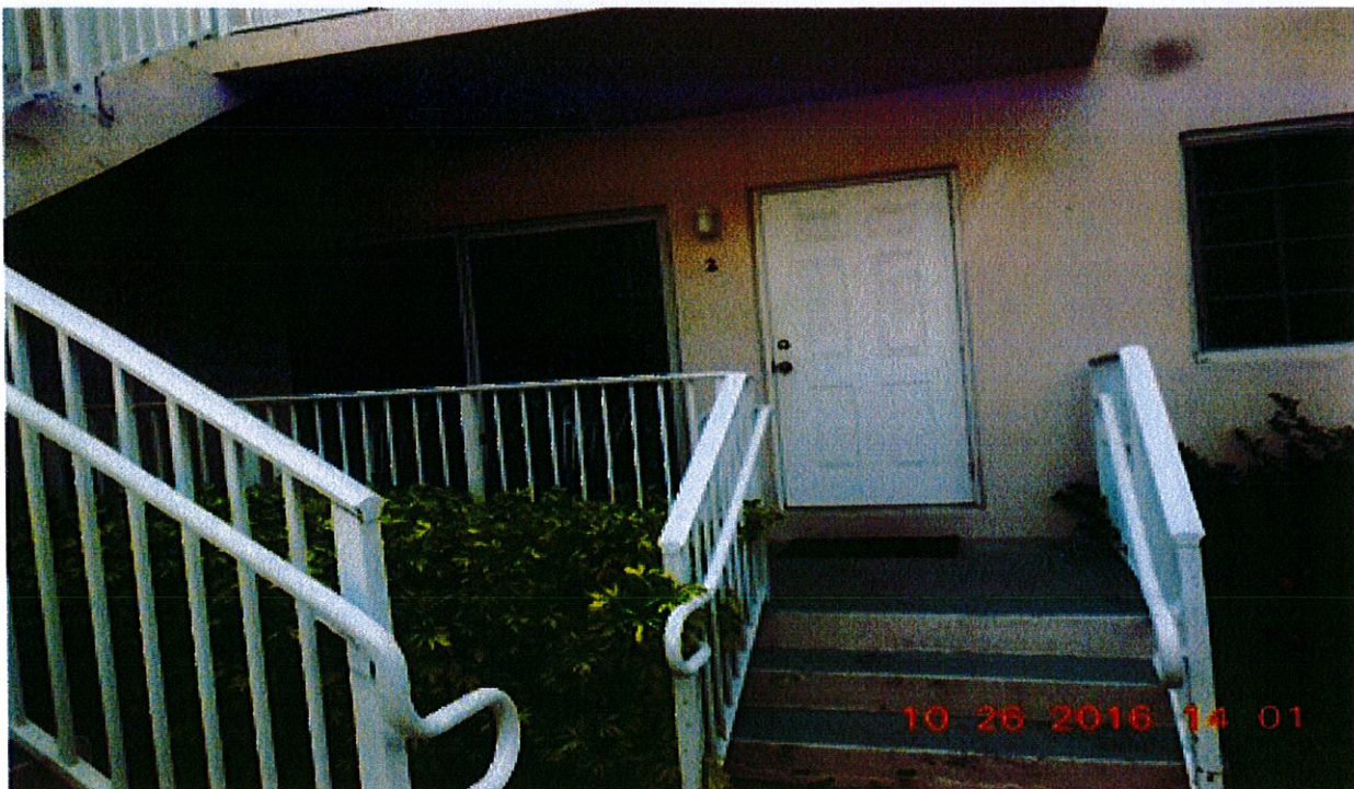
Unit # 2- No violations observed. (2 of 16 units)
