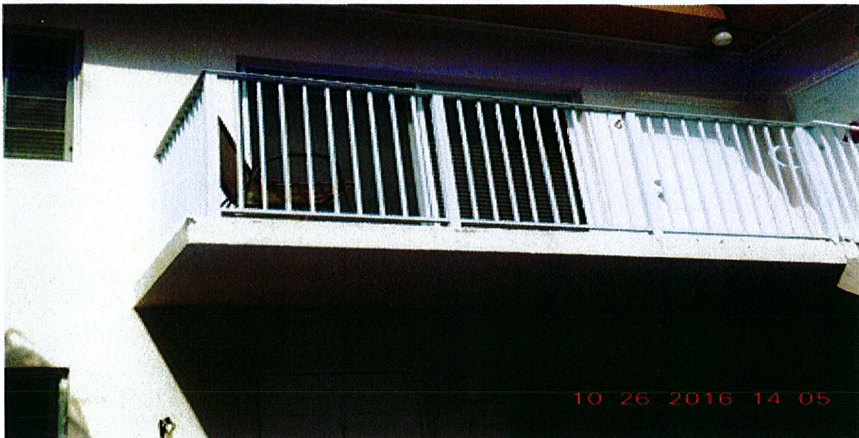
Unit # 26- No violations observed. (15 of 16 units)
