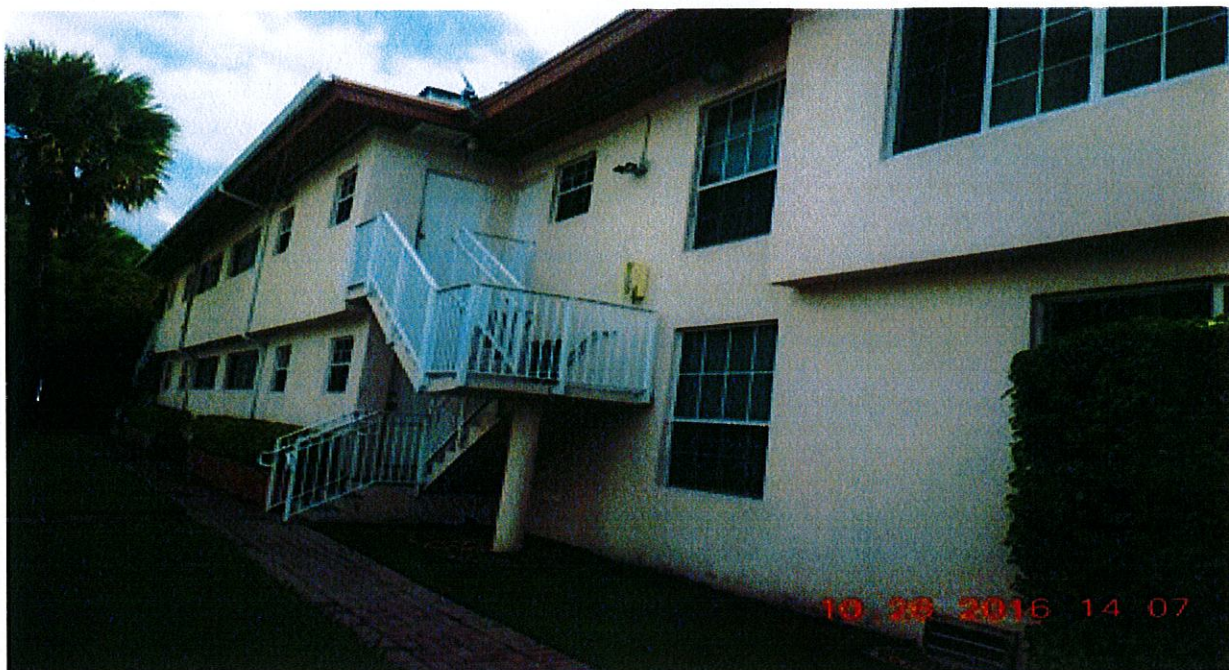
9280 North side- No violations observed.
