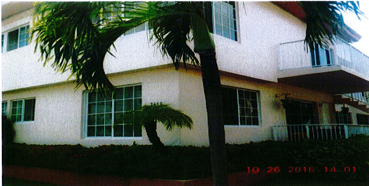
Building 9260- No violations observed.
