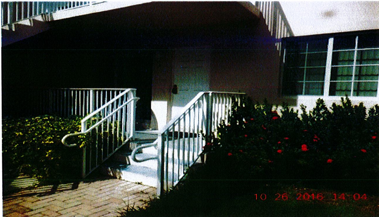
Unit # 7- No violations observed. (11 of 16 units)
