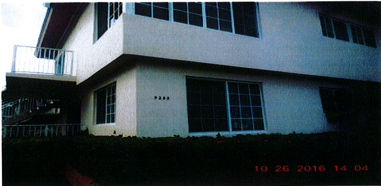
Building 9280- No violations observed.
