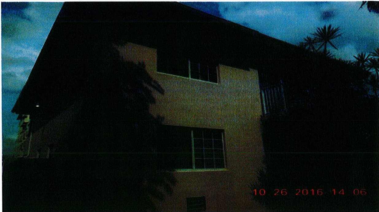
9280 Rear view- No violations observed.
