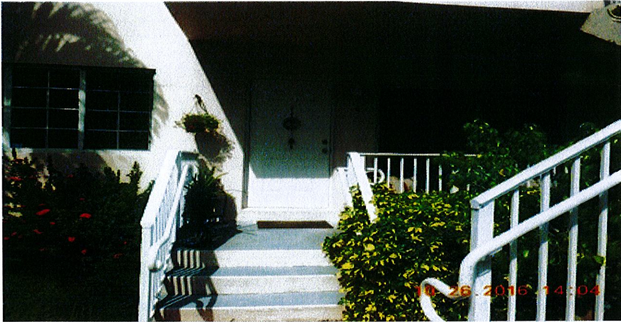
Unit #6- No violations observed. (10 of 16 units)
