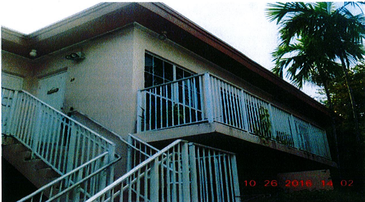
Unit # 24- No violation observed. (5 of 16 units)
