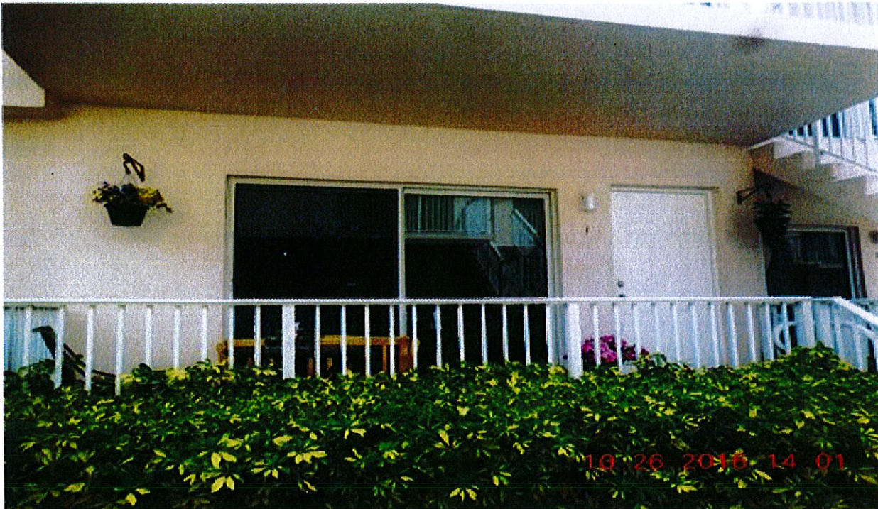
Unit # 1- No violations observed. (1 of 16 units)
