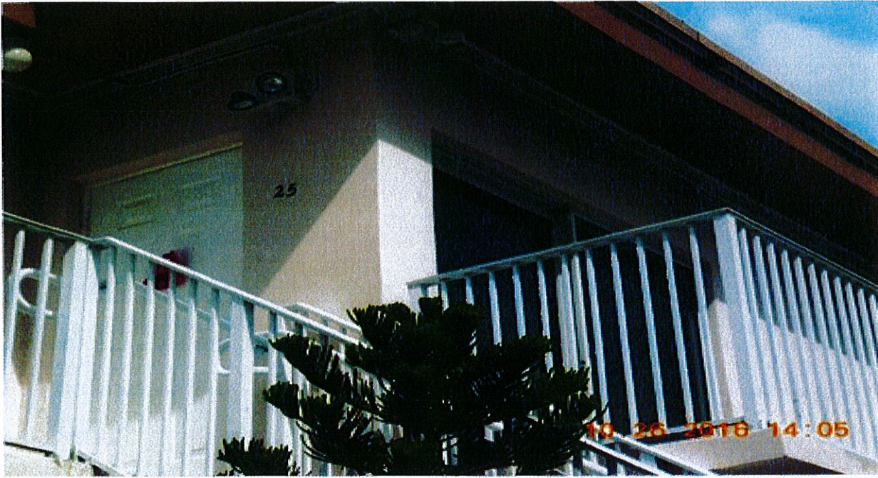
Unit #27- No violations observed. (16 of 16 units)
