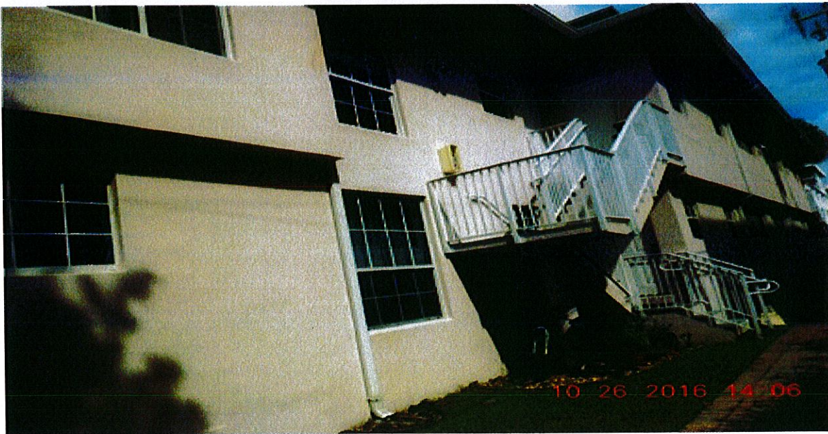
9260 South side- No violations observed.
