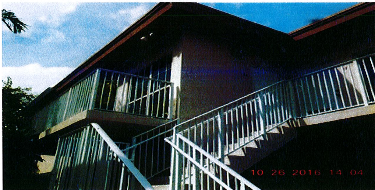
Unit #28- No violations observed. (13 of 16 units)
