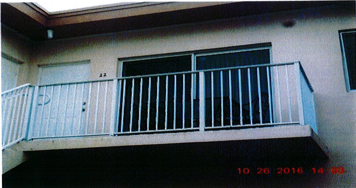
Unit # 22- No violations observed. (7 of 16 units)
