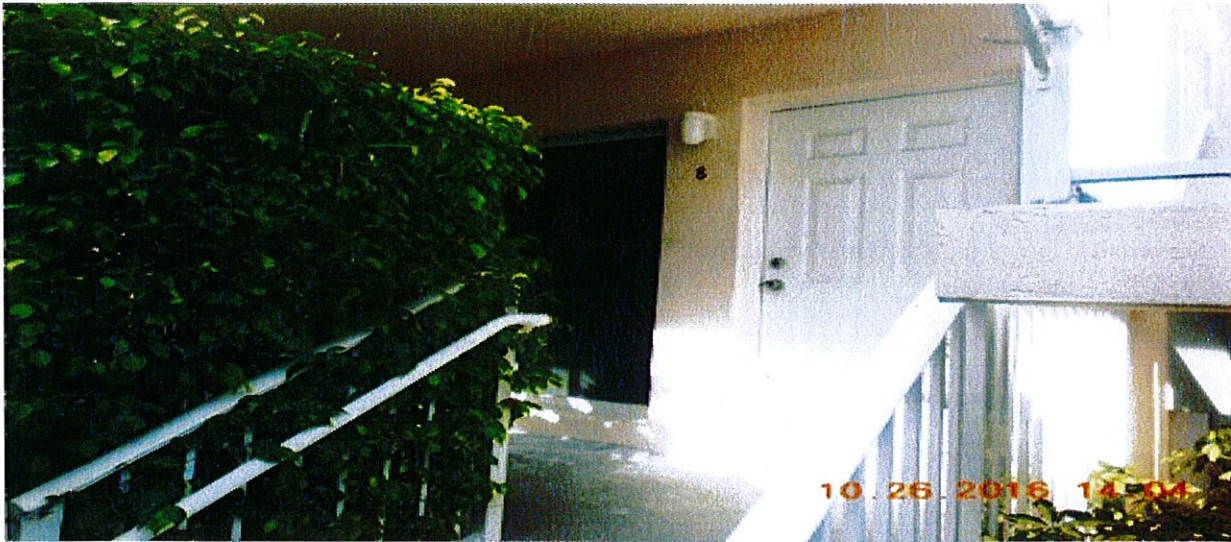
Unit #8 – No violations observed. (12 of 16 units)
