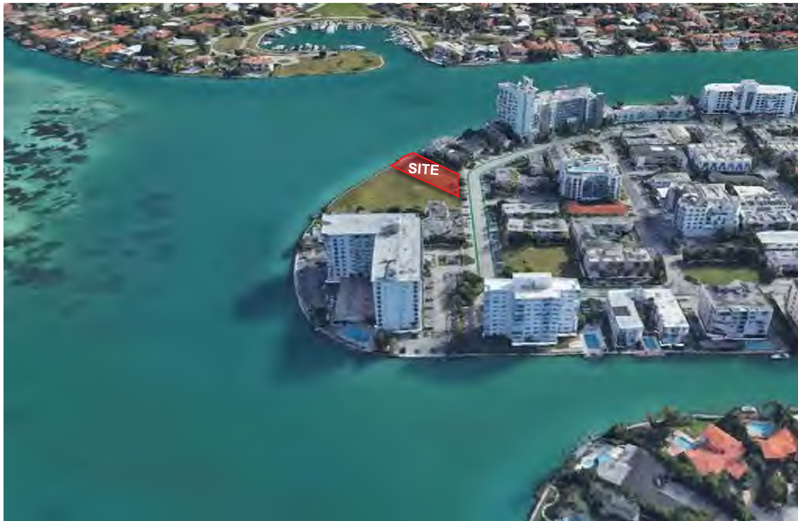
VIEW 03 - LOOKING EAST
