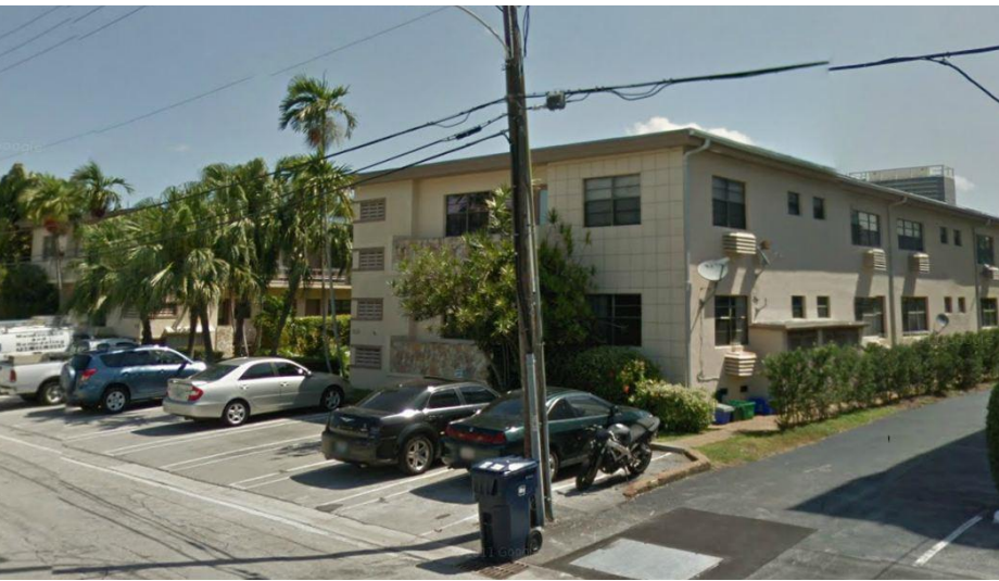
OFFICE, BUSINESS DISTRICT FLUM: COMMERCIAL 1 STORY
