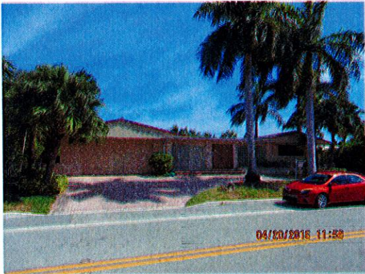
1351 99 STREET (ADJACENT ON EAST SIDE)
