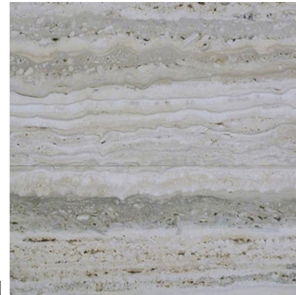
07 STONE CLADDING TRAVERTINE ACCENT WALLS
