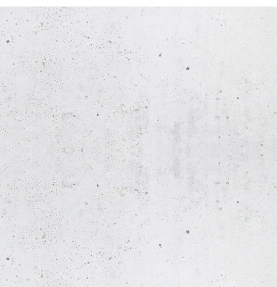
05 SMOOTH EXPOSED ARCHITECTURAL CONCRETE ROUND COLUMNS
