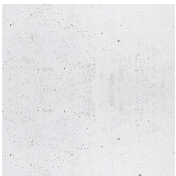
05 SMOOTH EXPOSED ARCHITECTURAL CONCRETE ROUND COLUMNS
