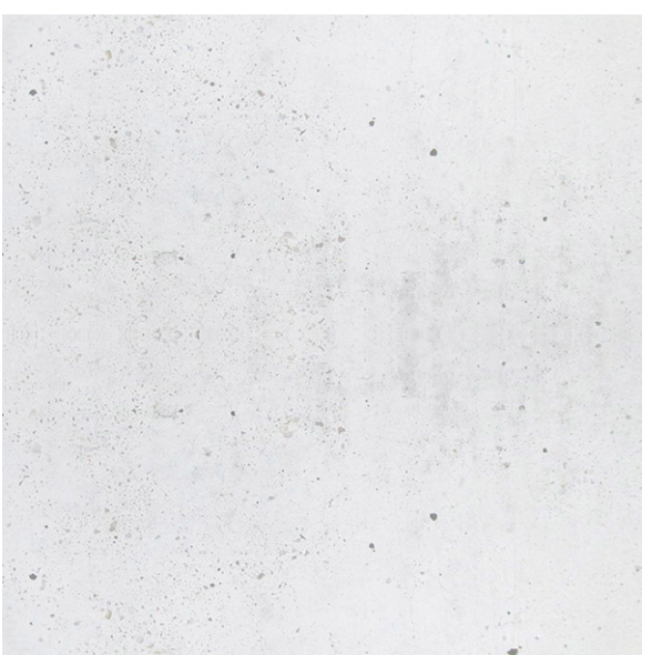
05 SMOOTH EXPOSED ARCHITECTURAL CONCRETE ROUND COLUMNS
