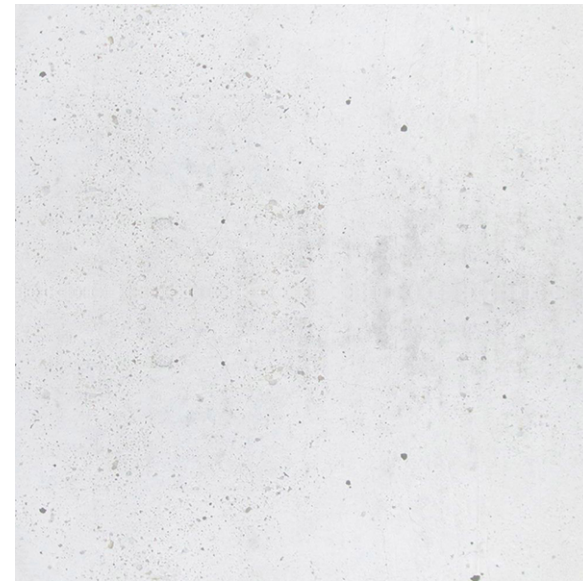
05 SMOOTH EXPOSED ARCHITECTURAL CONCRETE ROUND COLUMNS
