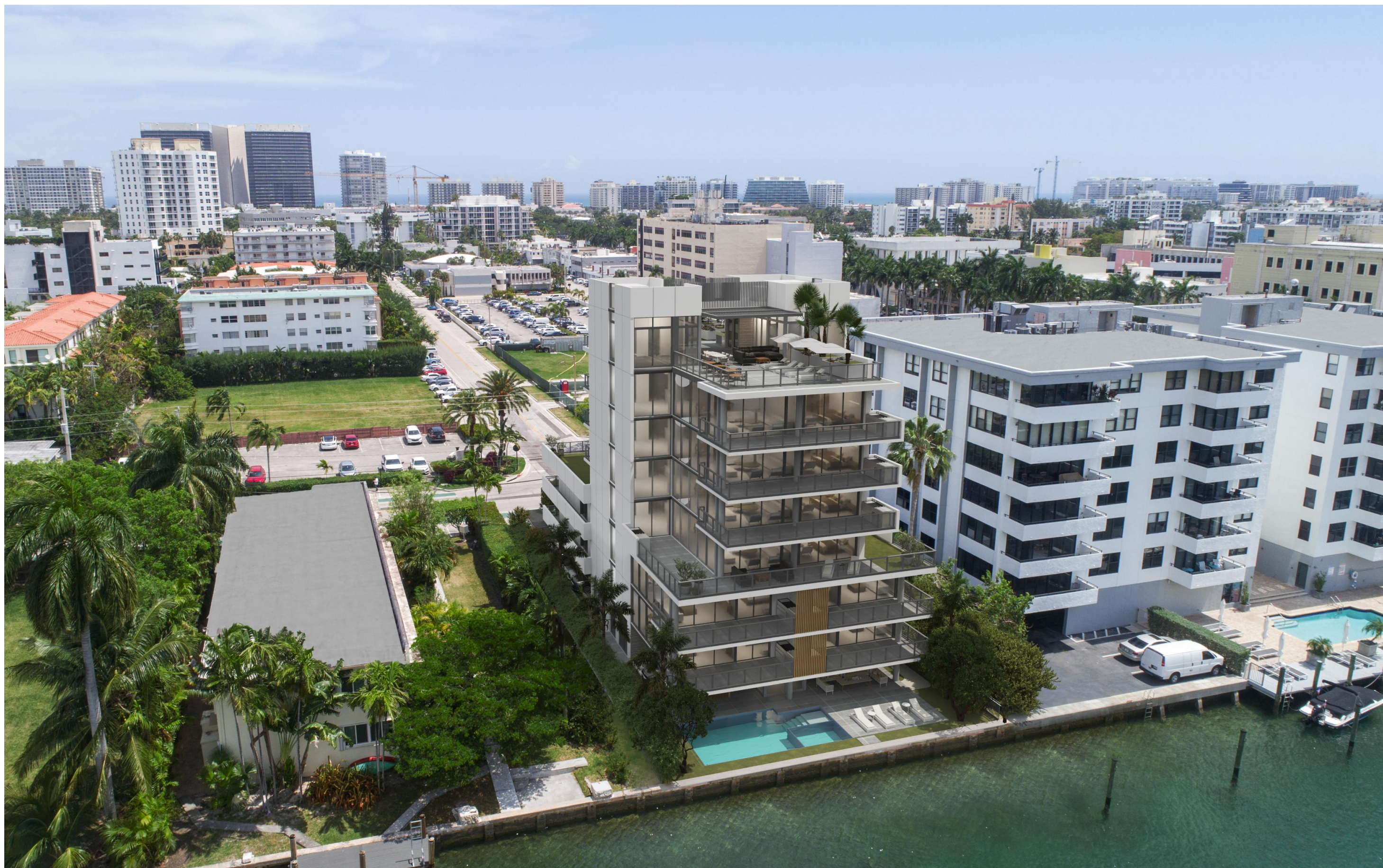
4 A-102 AERIAL VIEW - LOOKING S.W. NOT TO SCALE
