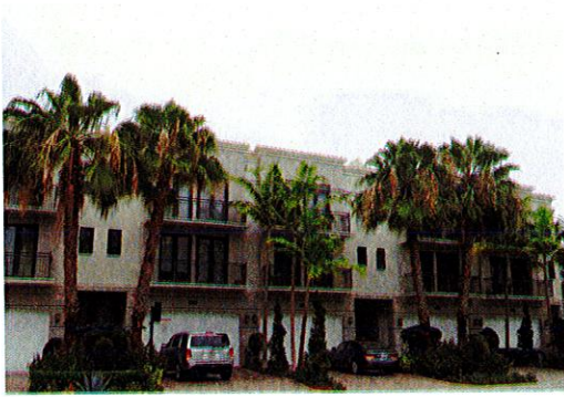
WEST SIDE ADJOINING BUILDING
