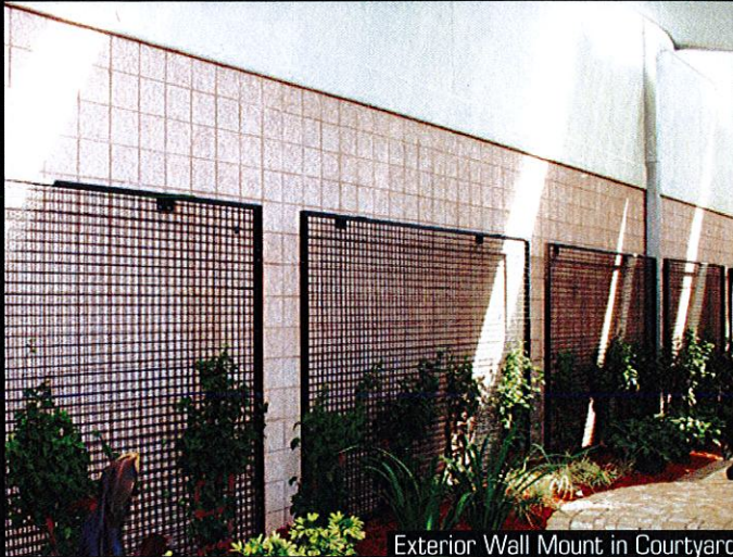
Exterior Wall Mount in Courtyard
