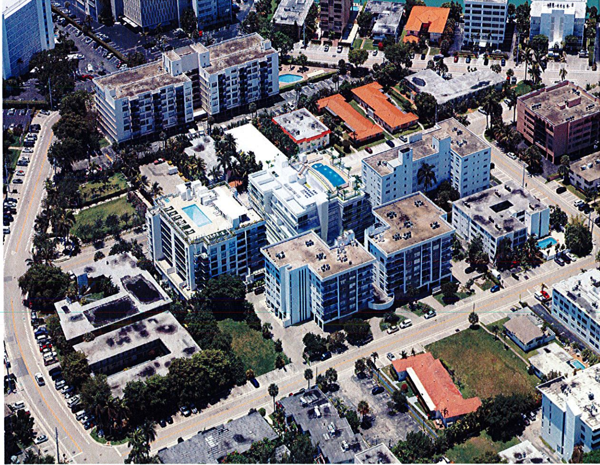
AERIAL VIEW FROM NORTHEAST
