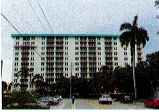
WEST SIDE VIEW TO THE NORTH
