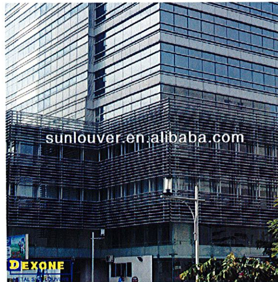
HORIZONTAL SCREENING IN FRONT OF GLAZING
