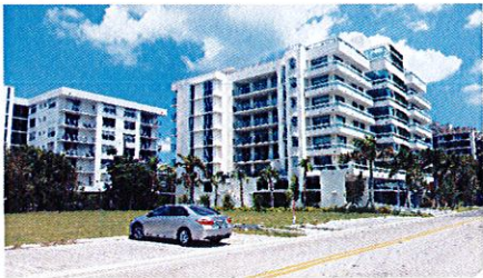
NE STREET VIEW
