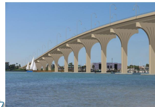
Bayway Structure E (SR 679) PD&E
