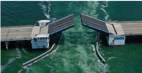
MAINTAIN BASCULE SPAN BRIDGE OPERATION
