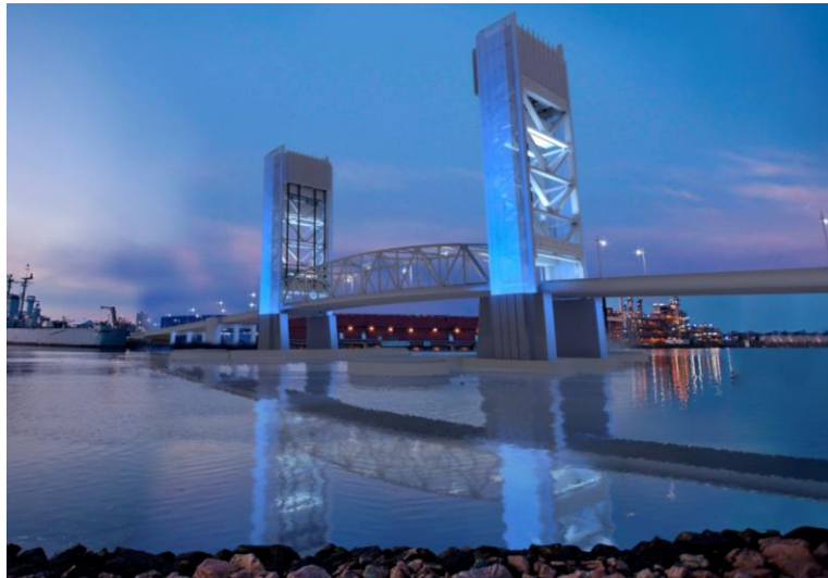
Fore River Bridge Replacement | Boston, MA
