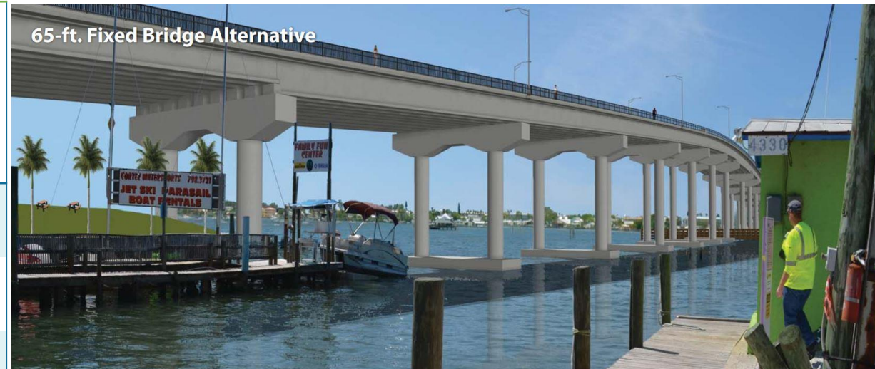
Cortez Boulevard Bridge PD&E
