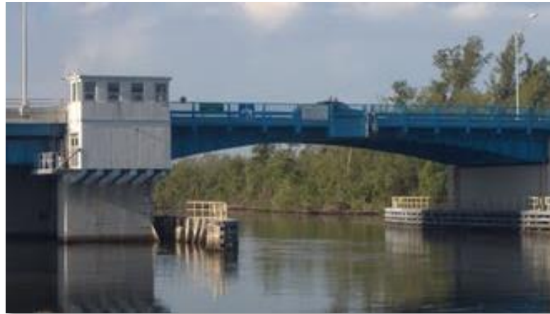
Dania Bascule Bridge, Ft. Lauderdale | FDOT – District 4
