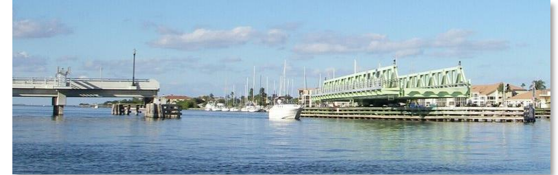
Mathers Swing Bridge, Merritt Island | FDOT – District 5
