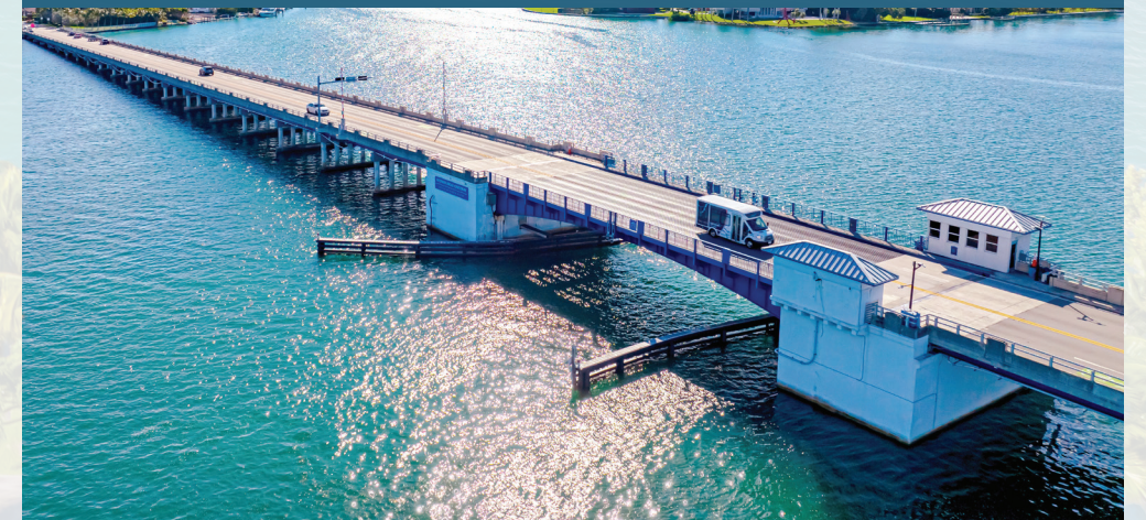
BROAD CAUSEWAY BRIDGE REHABILITATION
