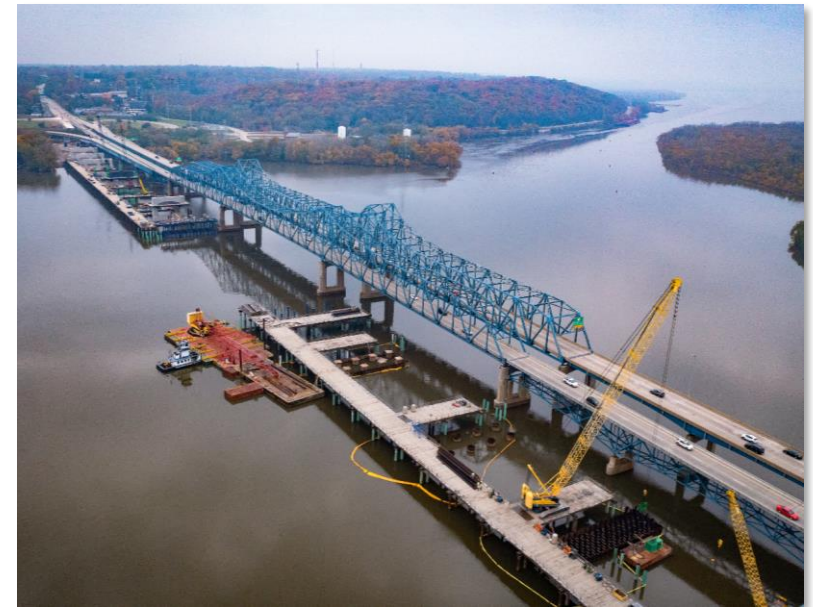
McCluggage Bridge over the Illinois River Illinois DOT
