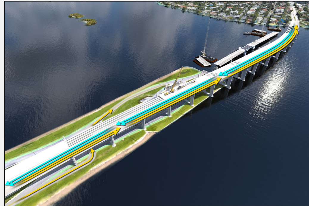
PHASE 3 – EXISTING BRIDGE NO LONGER USED
