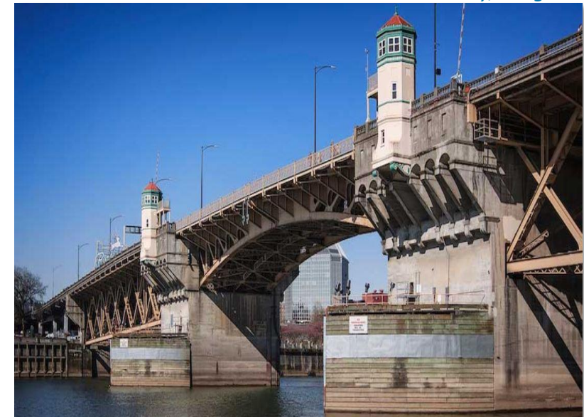
DPW Burnside Bridge Replacement Multnomah County, Oregon
