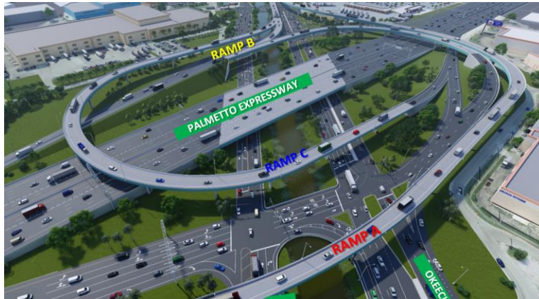
SR 826 at US 27/Okeechobee Road PD&E & Design Services | FDOT – District 6
