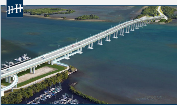
NORTH CAUSEWAY BRIDGE, FT PIERCE
