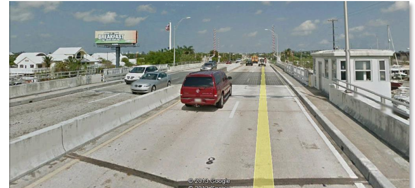
SR 84 Bascule Bridge, Ft. Lauderdale | FDOT – District 4
