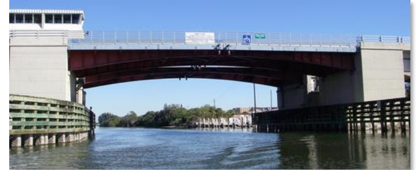
Christa McAuliffe Bridge, Merritt Island | FDOT – District 5
