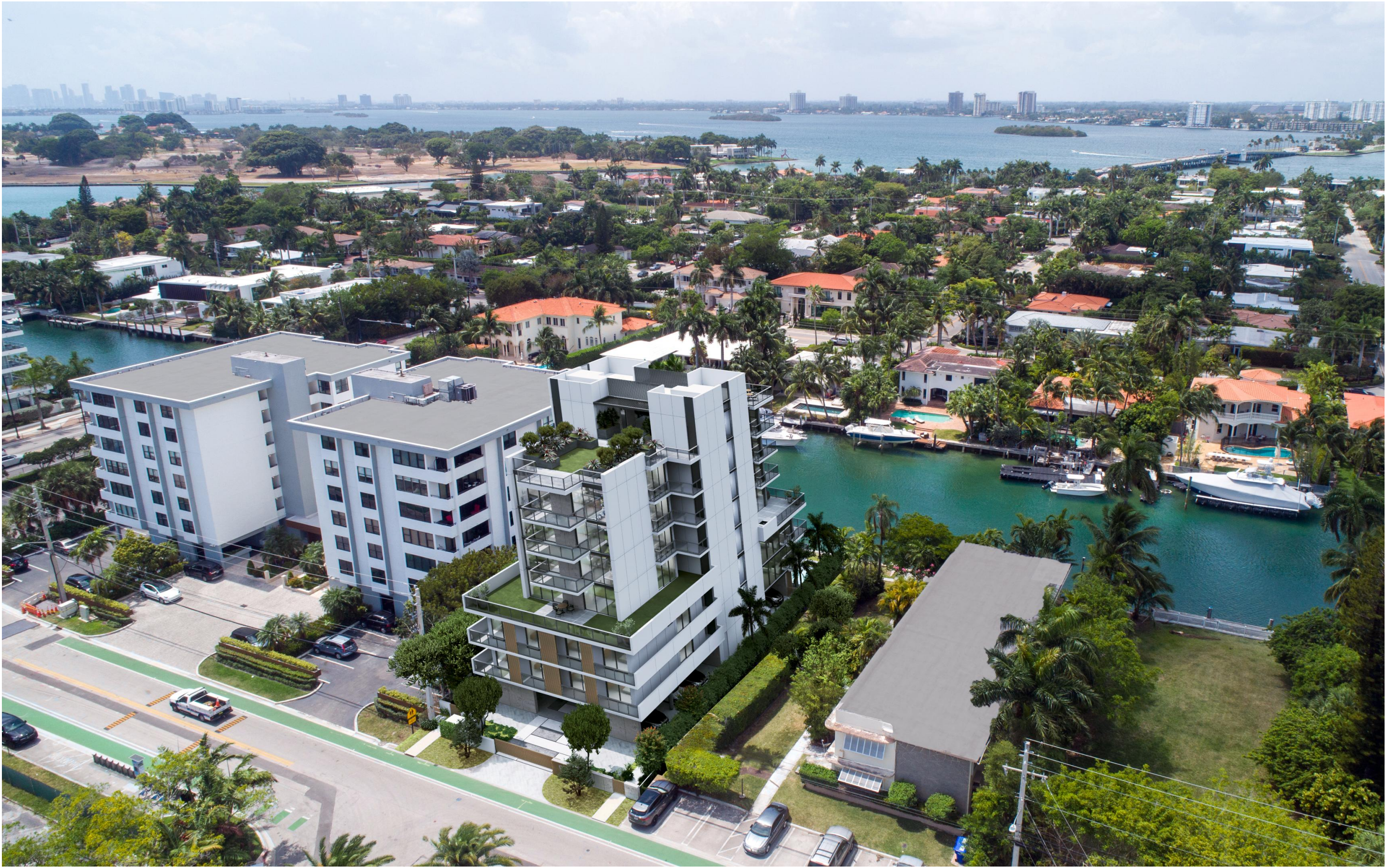
1 A-102 AERIAL VIEW - LOOKING S.W. NOT TO SCALE
