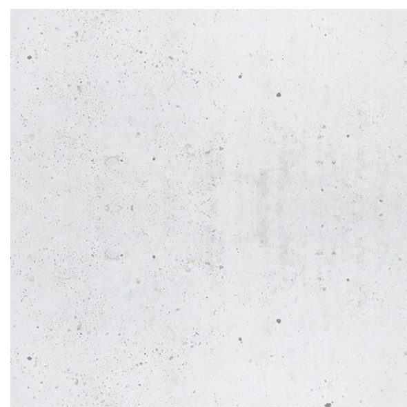
05 SMOOTH EXPOSED ARCHITECTURAL CONCRETE ROUND COLUMNS
