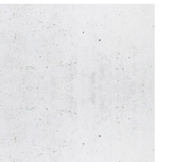
05 SMOOTH EXPOSED ARCHITECTURAL CONCRETE ROUND COLUMNS
