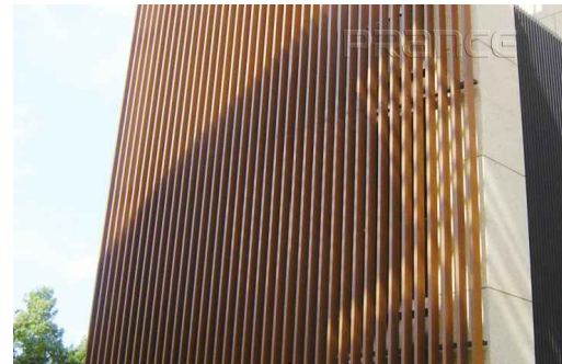
BRONZE, SILVER, GOLD ALUMINUM TUBES ON FRONT FACADE,
