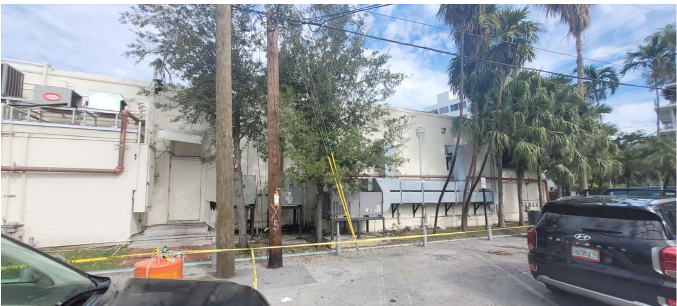
10. VIEW OF SITE WEST (SIDE)
