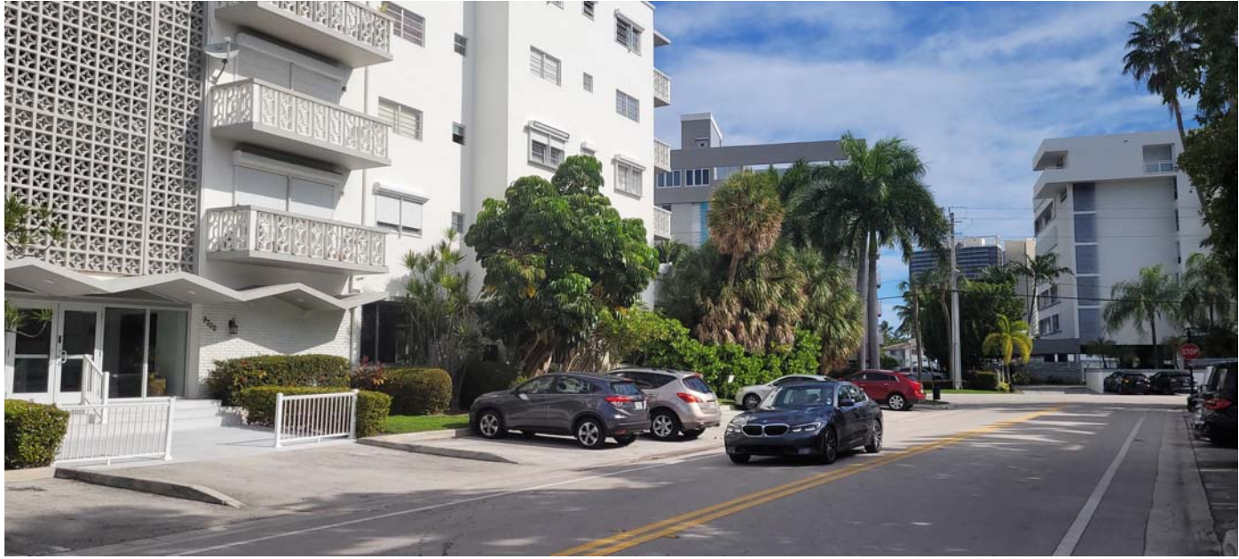
8. VIEW OF BUILDINGS ON NORTH (SIDE)
