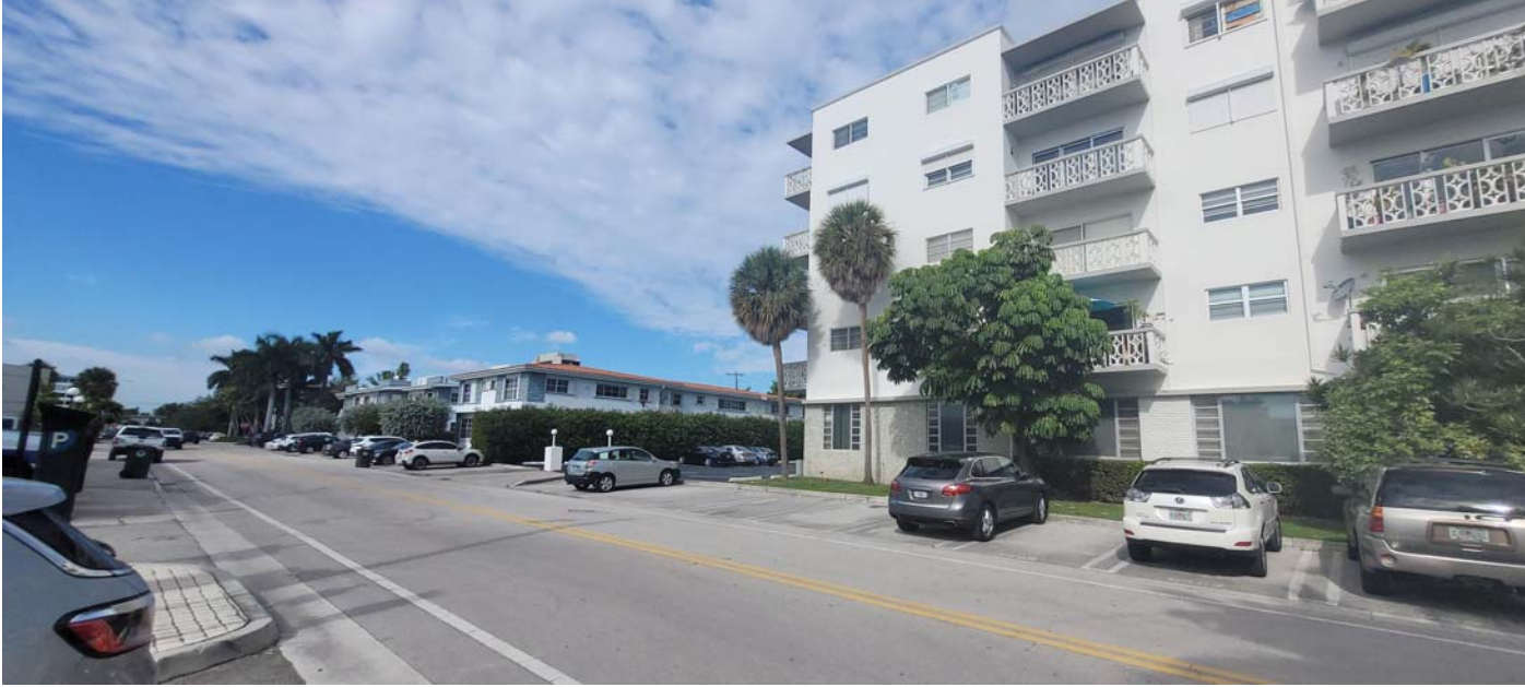
9. VIEW OF BUILDINGS ON NORTH (SIDE)
