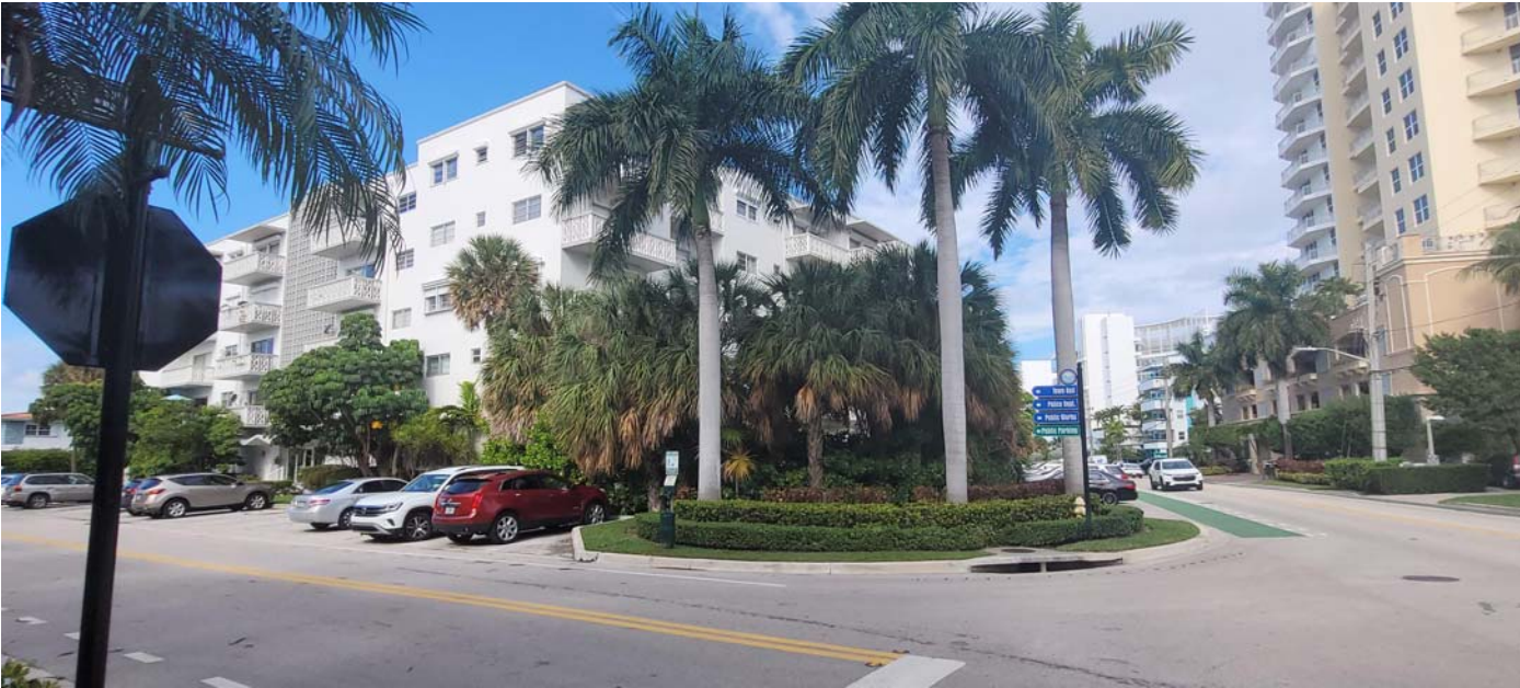
7. VIEW OF BUILDINGS ON NORTH (SIDE)
