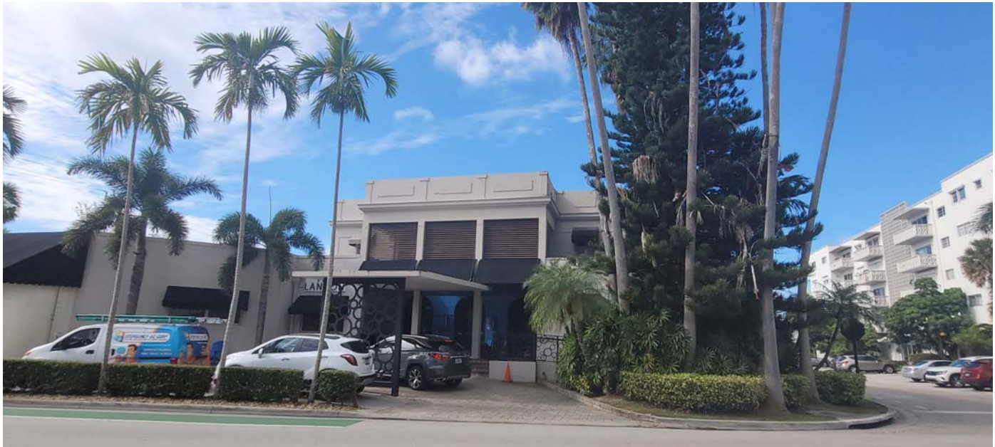
3. VIEW OF SITE FACING EAST (ENTRANCE)
