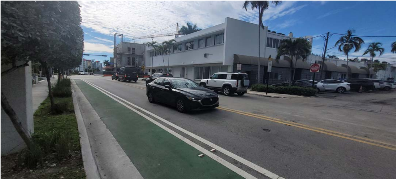
1. VIEW OF BUILDINGS ON THE SOUTH SIDE
