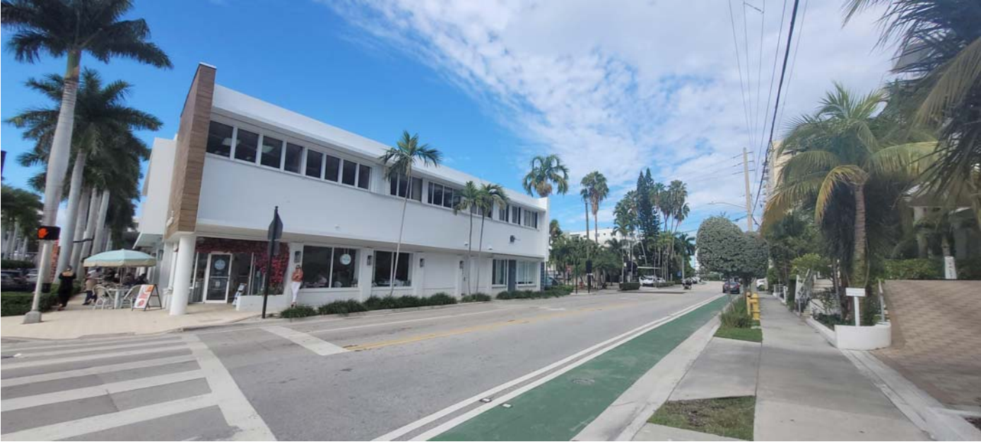
2. VIEW OF SITE FROM 96TH STREET
