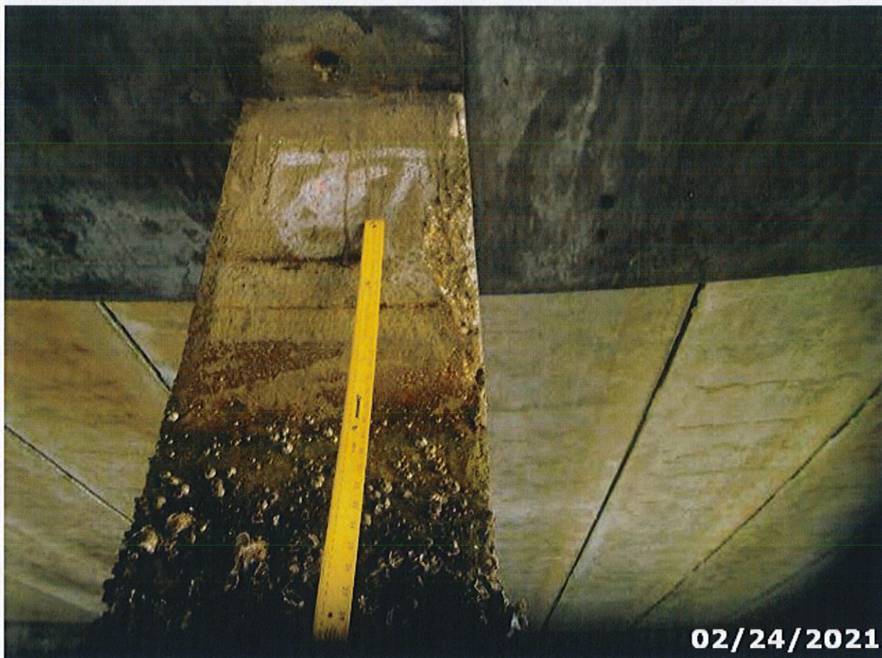
Photo 13 Element/Env 226/4: Pre. Concrete Pile
