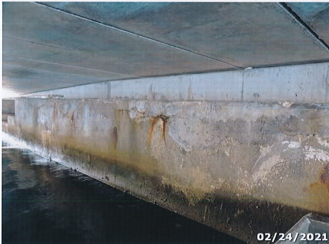
Photo 17 Element/Env 8393/4: Bulkhead Seawall Any Material
