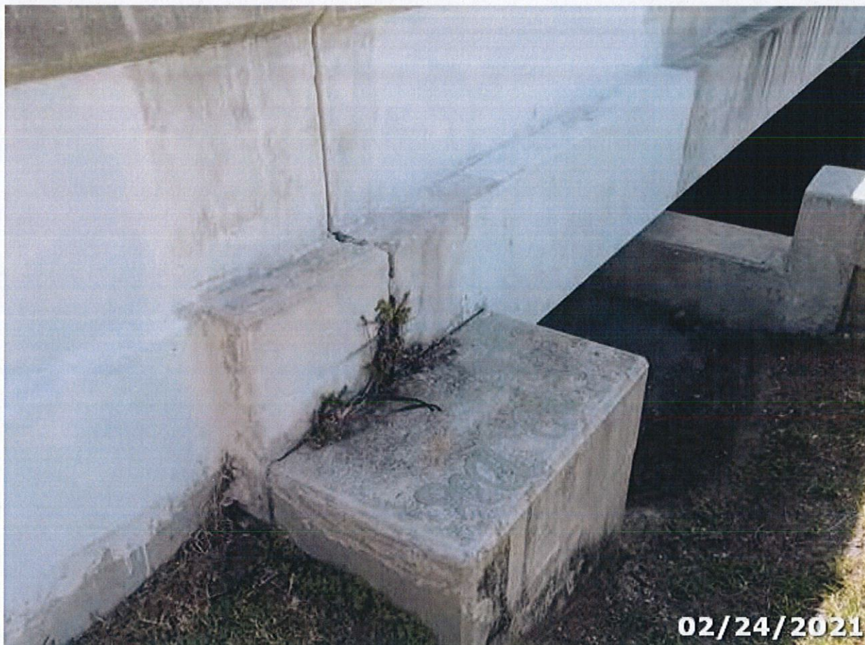
Photo 12 Element/Env 215/4: Re Conc Abutment
