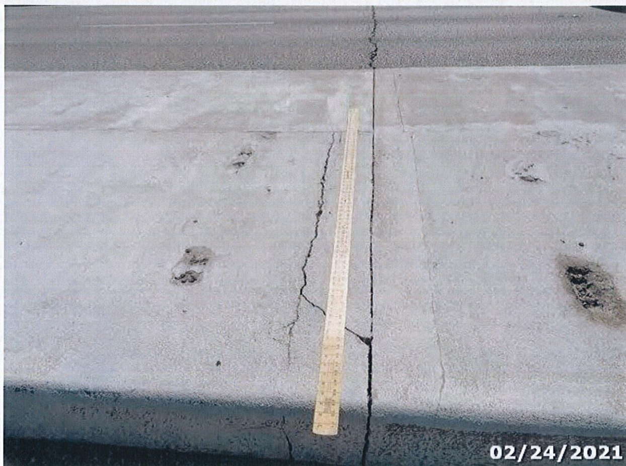
Photo 01 Element/Env 8099/4: PS Conc Slab (Sonovoid)
