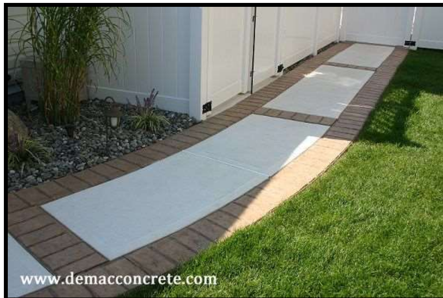
Figure 8: Colored Stamped Concrete Sidewalk
