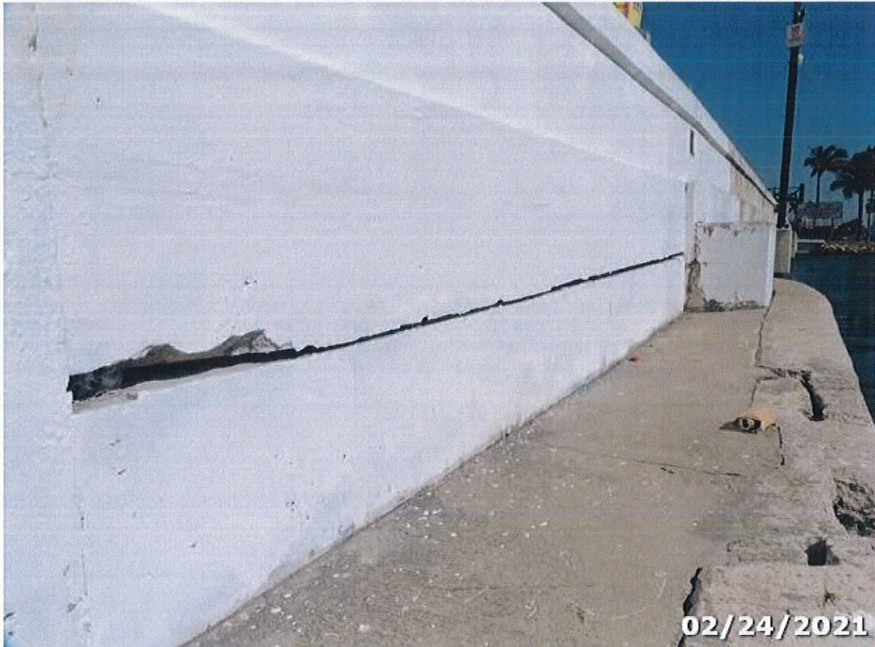
Photo 10 Element/Env 8475/4: R/Conc Walls
