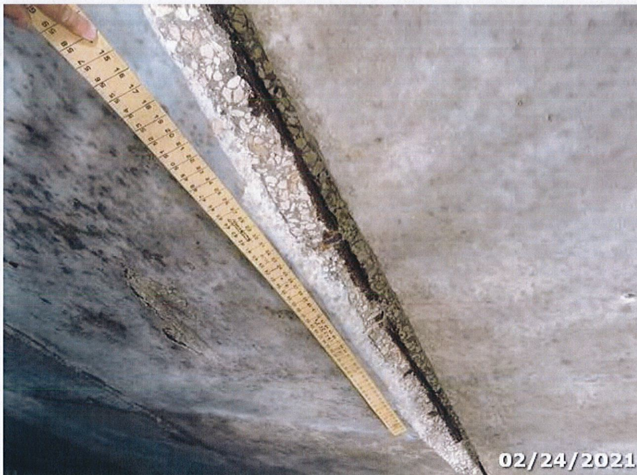
Photo 03 Element/Env 8099/4: PS Conc Slab (Sonovoid)
