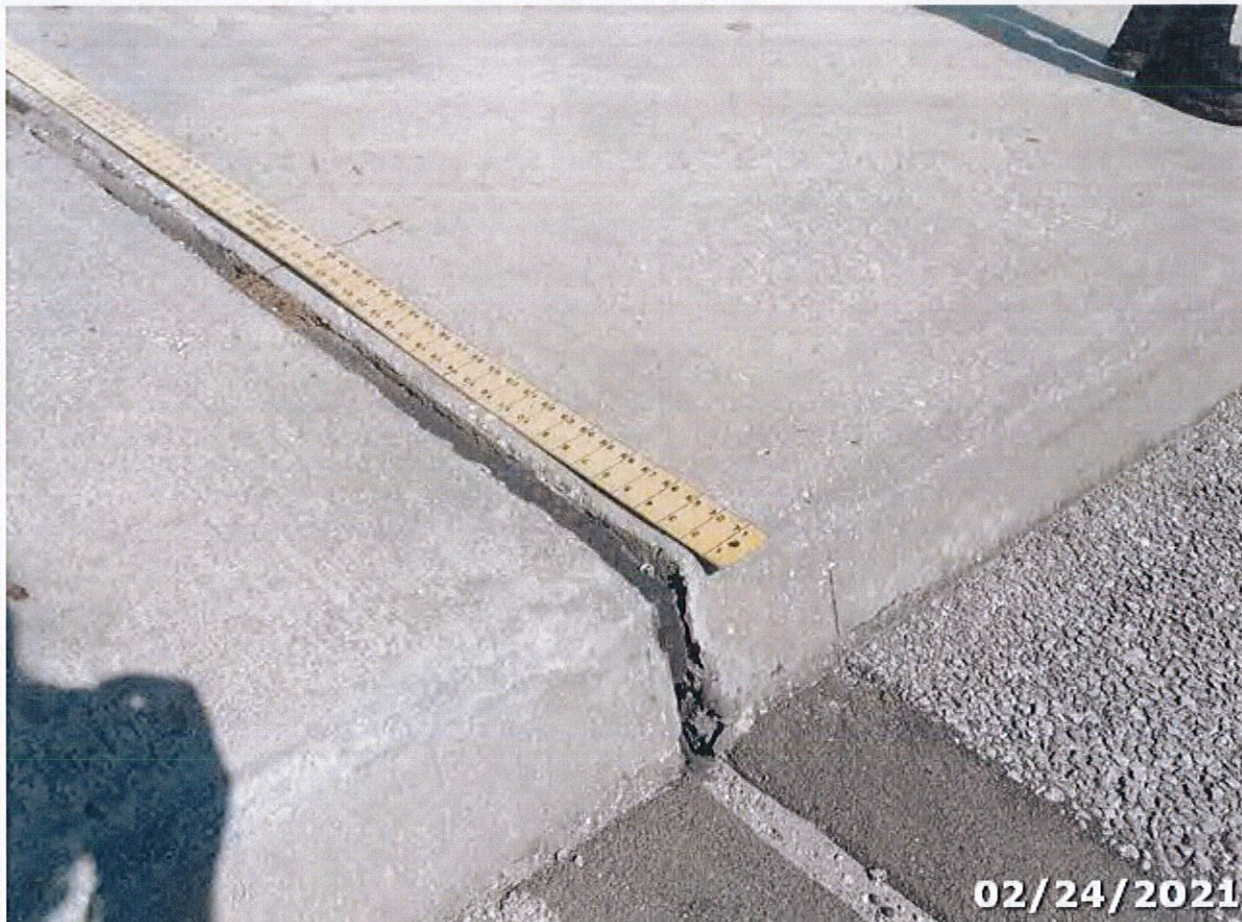
Photo 06 Element/Env 301/4: Pourable Joint Seal
