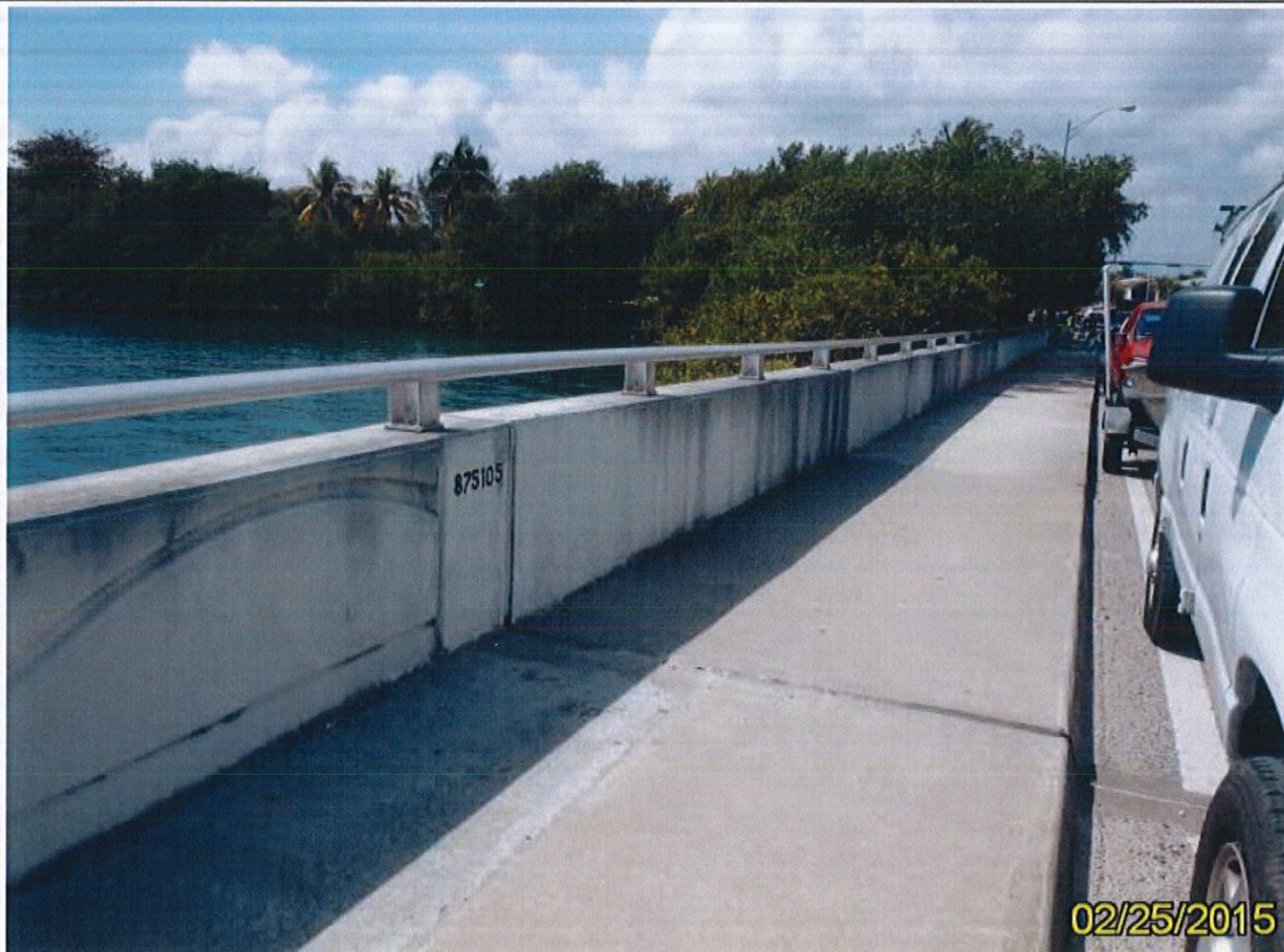
Southwest Oncoming Transition - 02/25/2015
