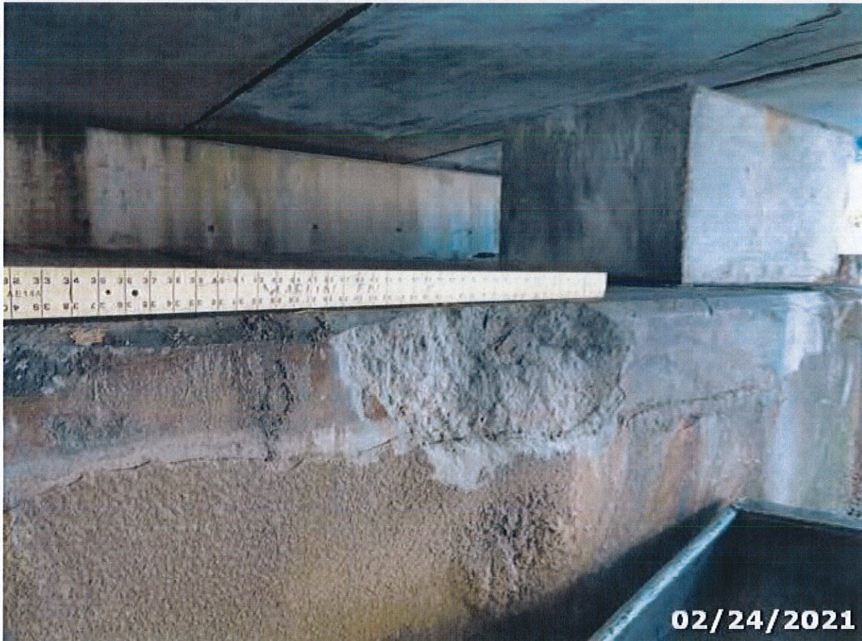
Photo 19 Element/Env 8393/4: Bulkhead Seawall Any Material
