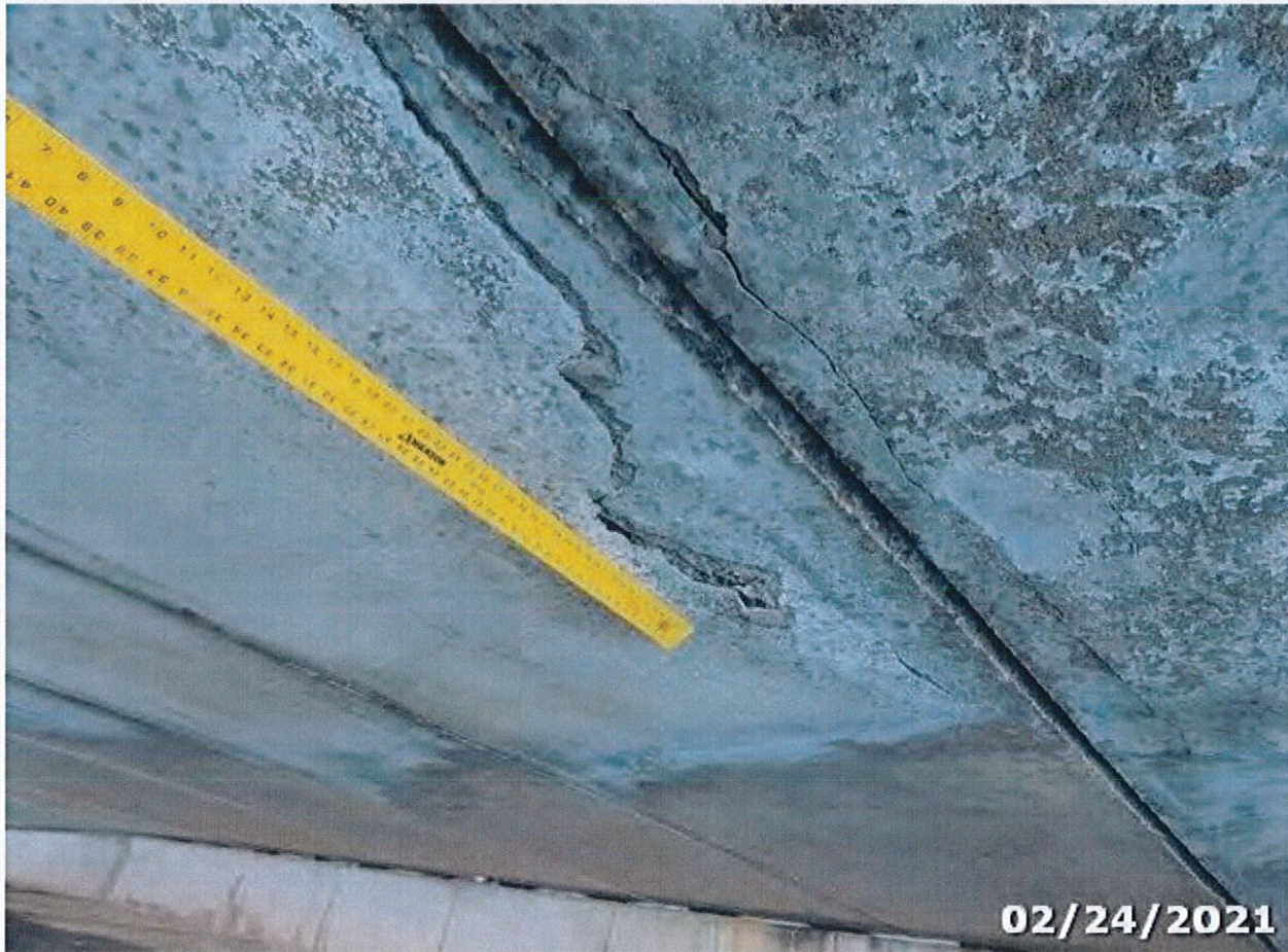
Photo 02 Element/Env 8099/4: PS Conc Slab (Sonovoid)
