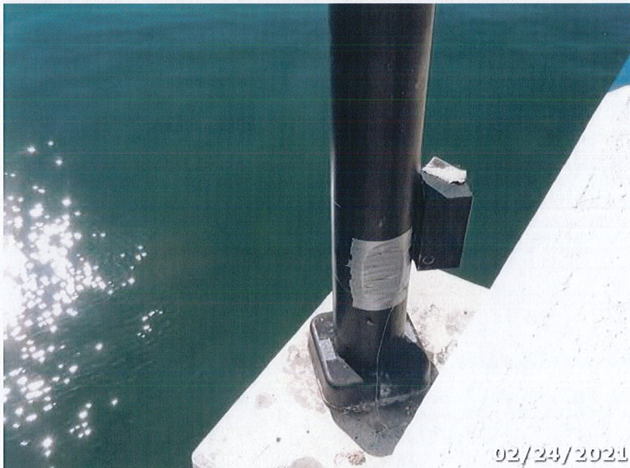
Photo 14 Element/Env 234/4: Re. Concrete Pier Cap
