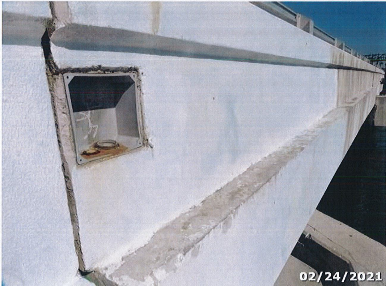
Photo 21 Element/Env 333/4: Other Bridge Railing
