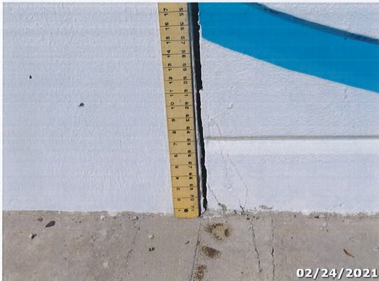
Photo 23 Element/Env 333/4: Other Bridge Railing
