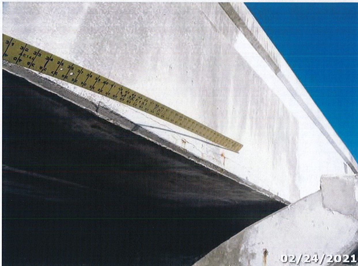
Photo 04 Element/Env 8099/4: PS Conc Slab (Sonovoid)
