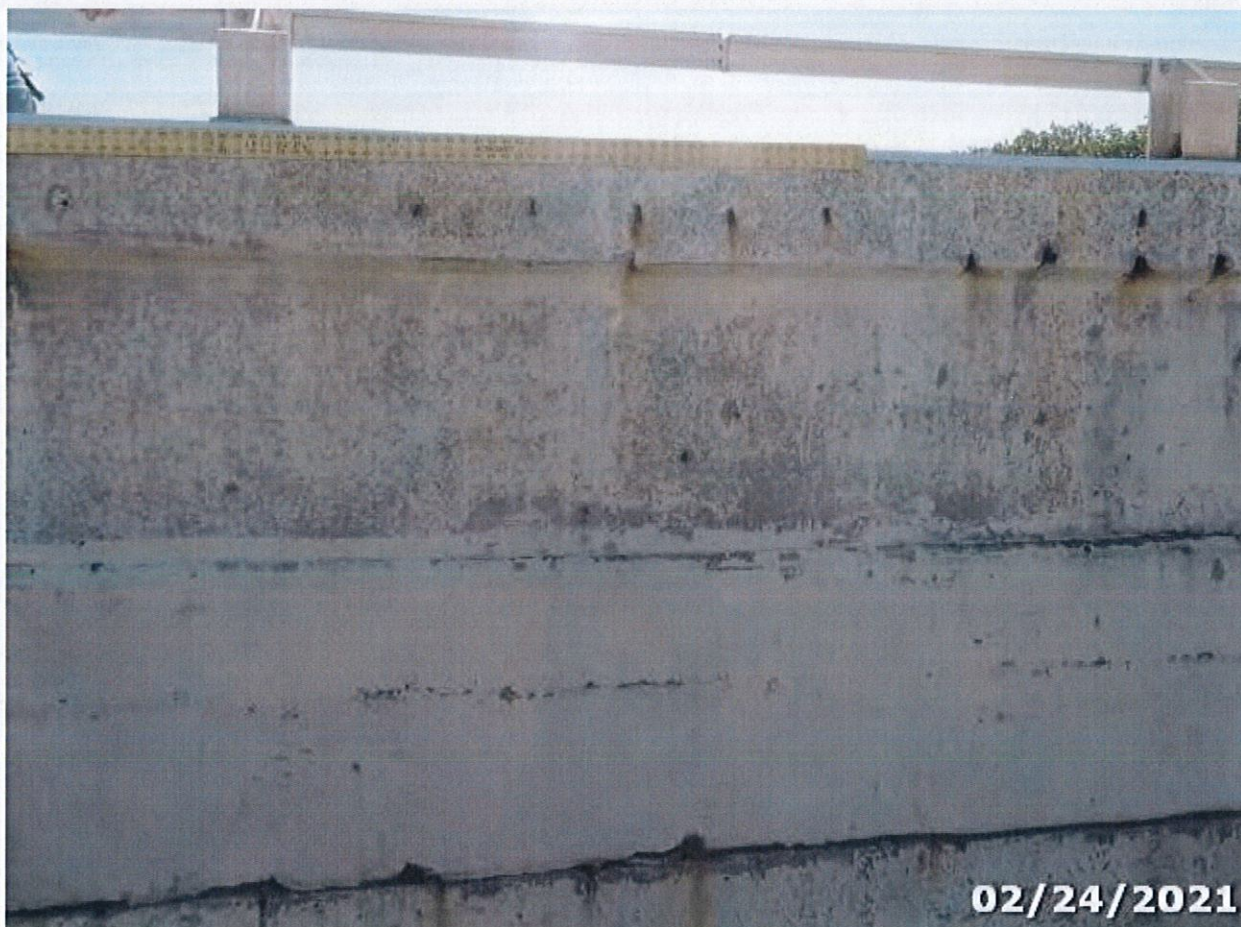
Photo 11 Element/Env 8475/4: R/Conc Walls
