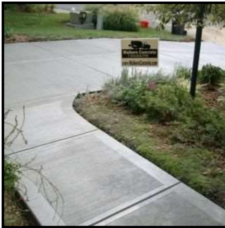
Figure 6: Plain Concrete with Broom Finish
