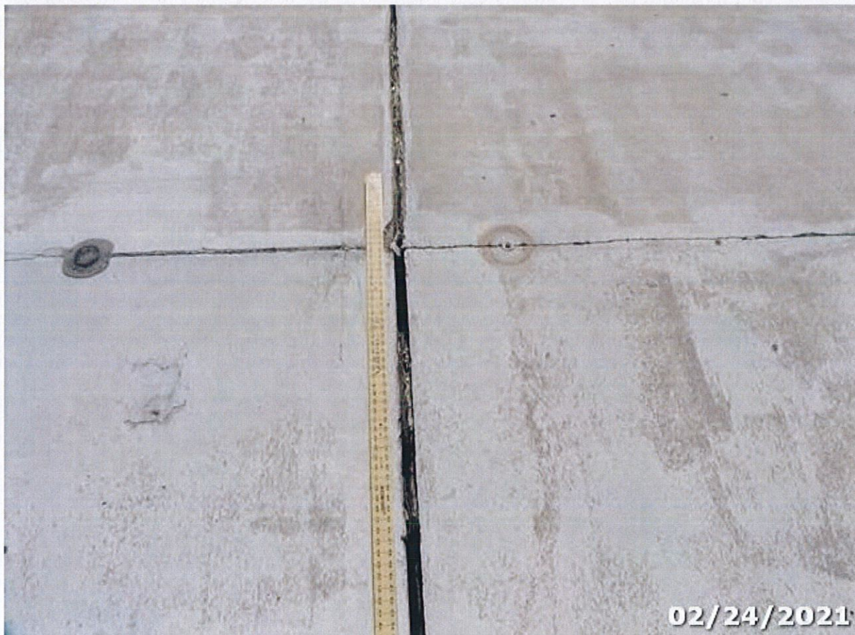
Photo 07 Element/Env 301/4: Pourable Joint Seal
