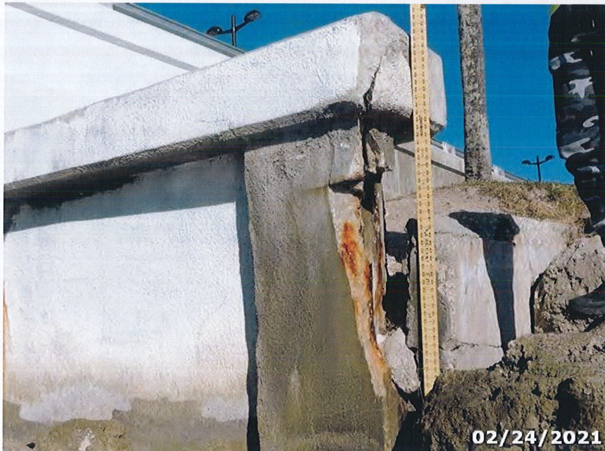
Photo 16 Element/Env 8393/4: Bulkhead Seawall Any Material
