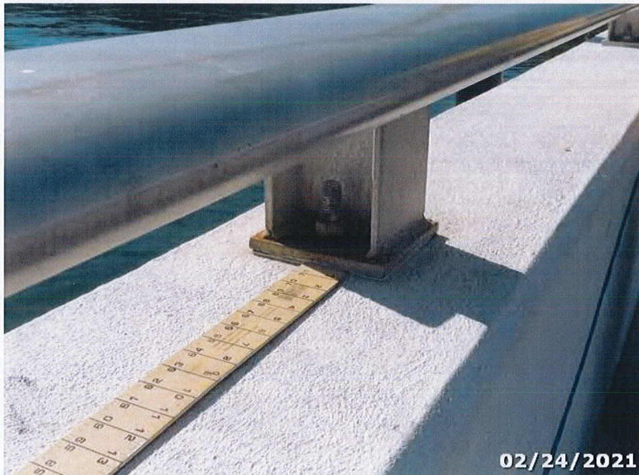
Photo 22 Element/Env 333/4: Other Bridge Railing
