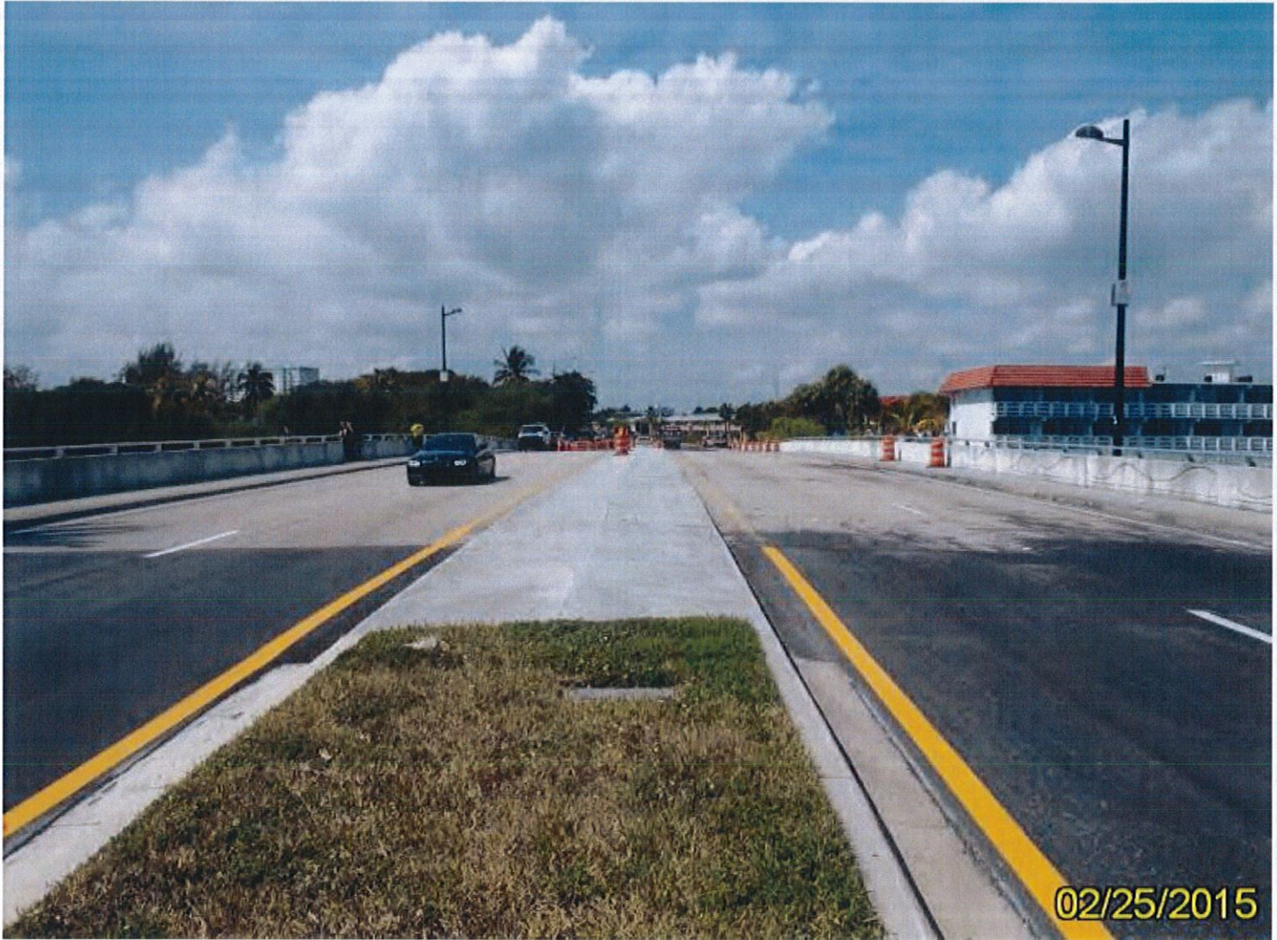
East Approach Looking West - 02/25/2015
