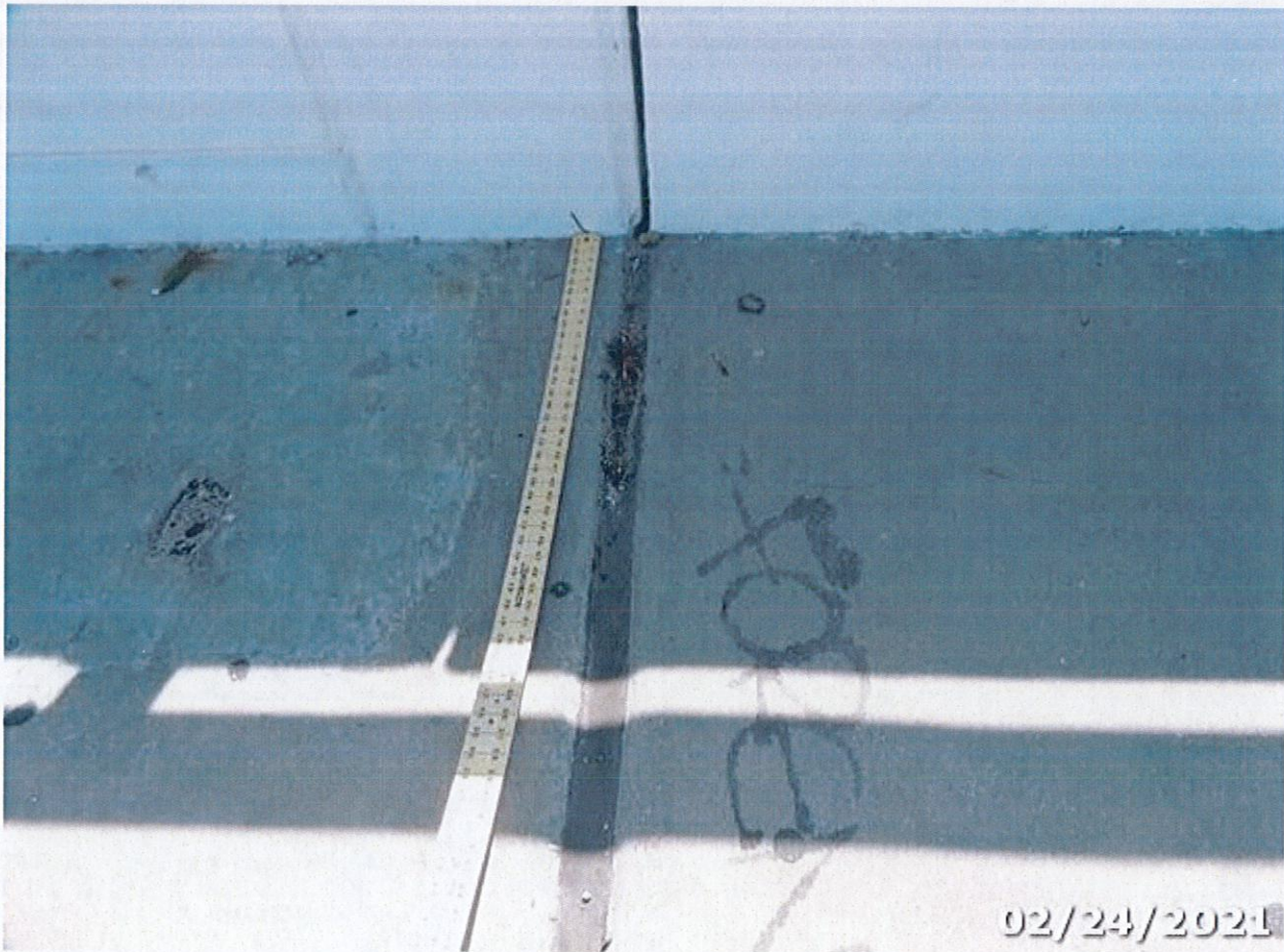
Photo 08 Element/Env 301/4: Pourable Joint Seal
