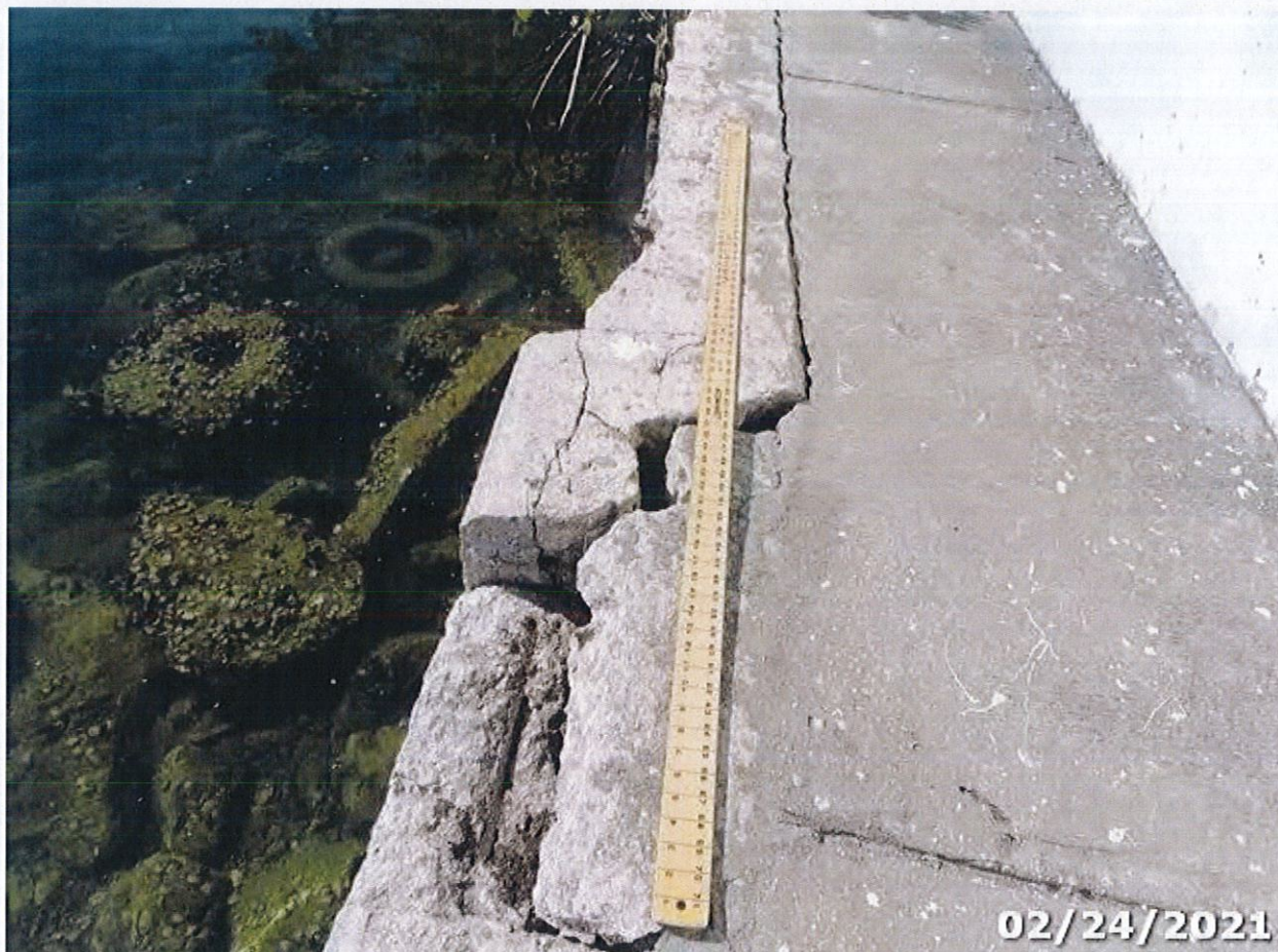
Photo 15 Element/Env 8393/4: Bulkhead Seawall Any Material
