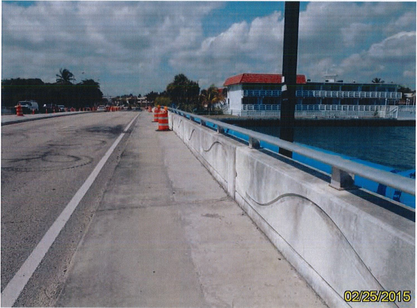
Typical Bridge Rail - 02/25/2015
