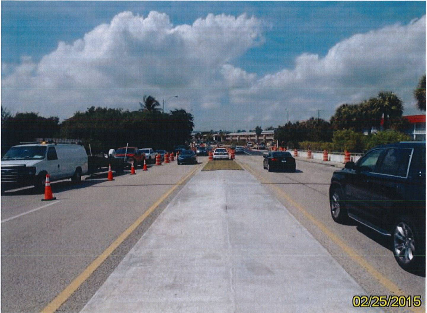
West Approach Looking West - 02/25/2015
