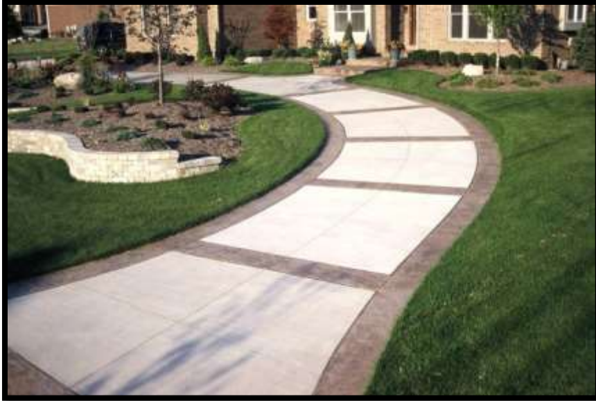
Figure 7: Colored Stamped Concrete Sidewalk
