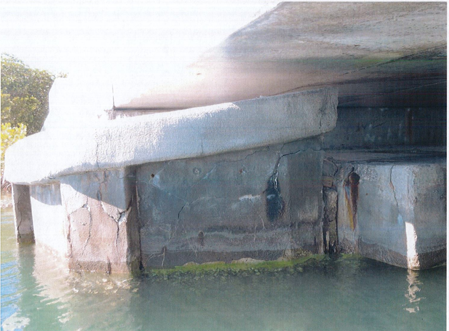
Photo 18 Element/Env 8393/4: Bulkhead Seawall Any Material
