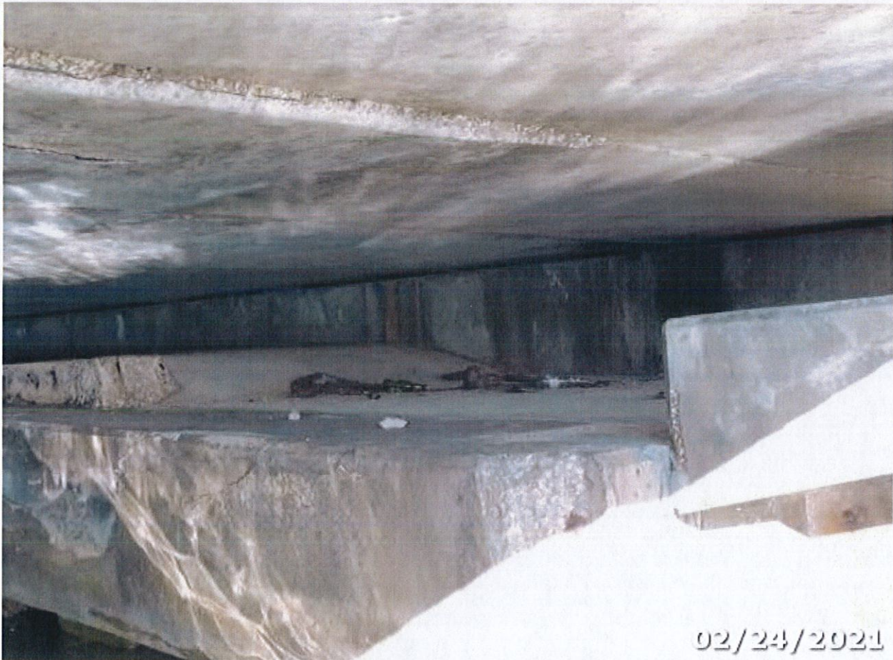
Photo 20 Element/Env 8394/4: R/Conc Abut Slope Protection
