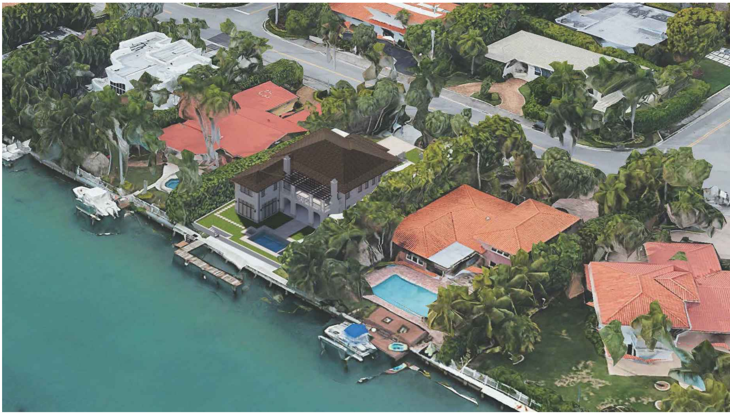
SOUTH (LEFT) AERIAL VIEW
