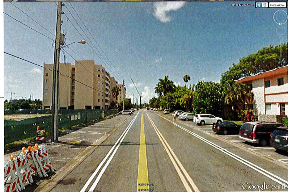
East Bay Harbor looking South
