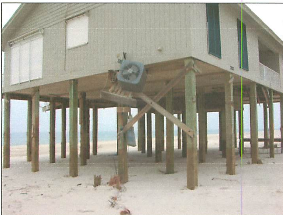
Figure 12-3. Small piles supporting a platform broken by floodborne debris
