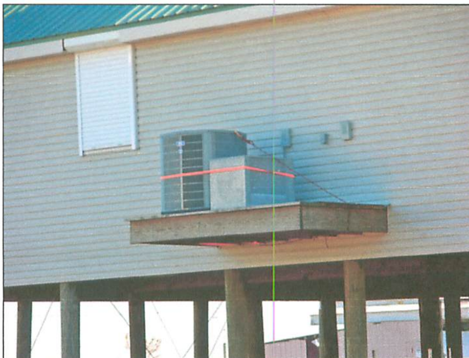
Figure 12-2. Proper elevation of an air-conditioning condenser in a floodprone area; additional anchorage is recommended
