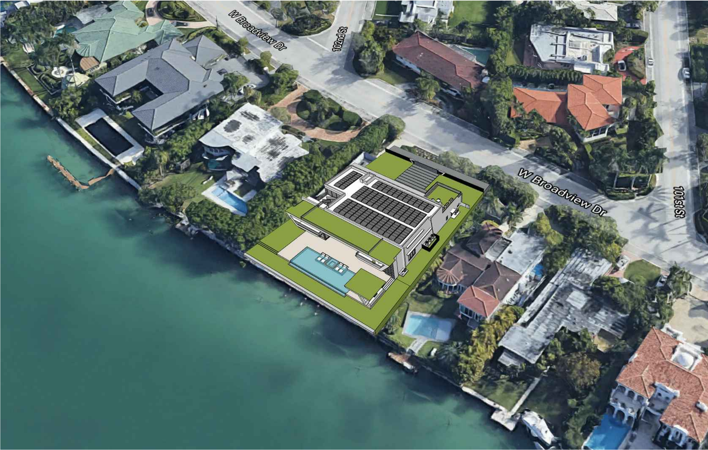
SOUTH WEST VIEW
