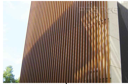
BRONZE, SILVER, GOLD ALUMINUM TUBES ON FRONT FACADE,
