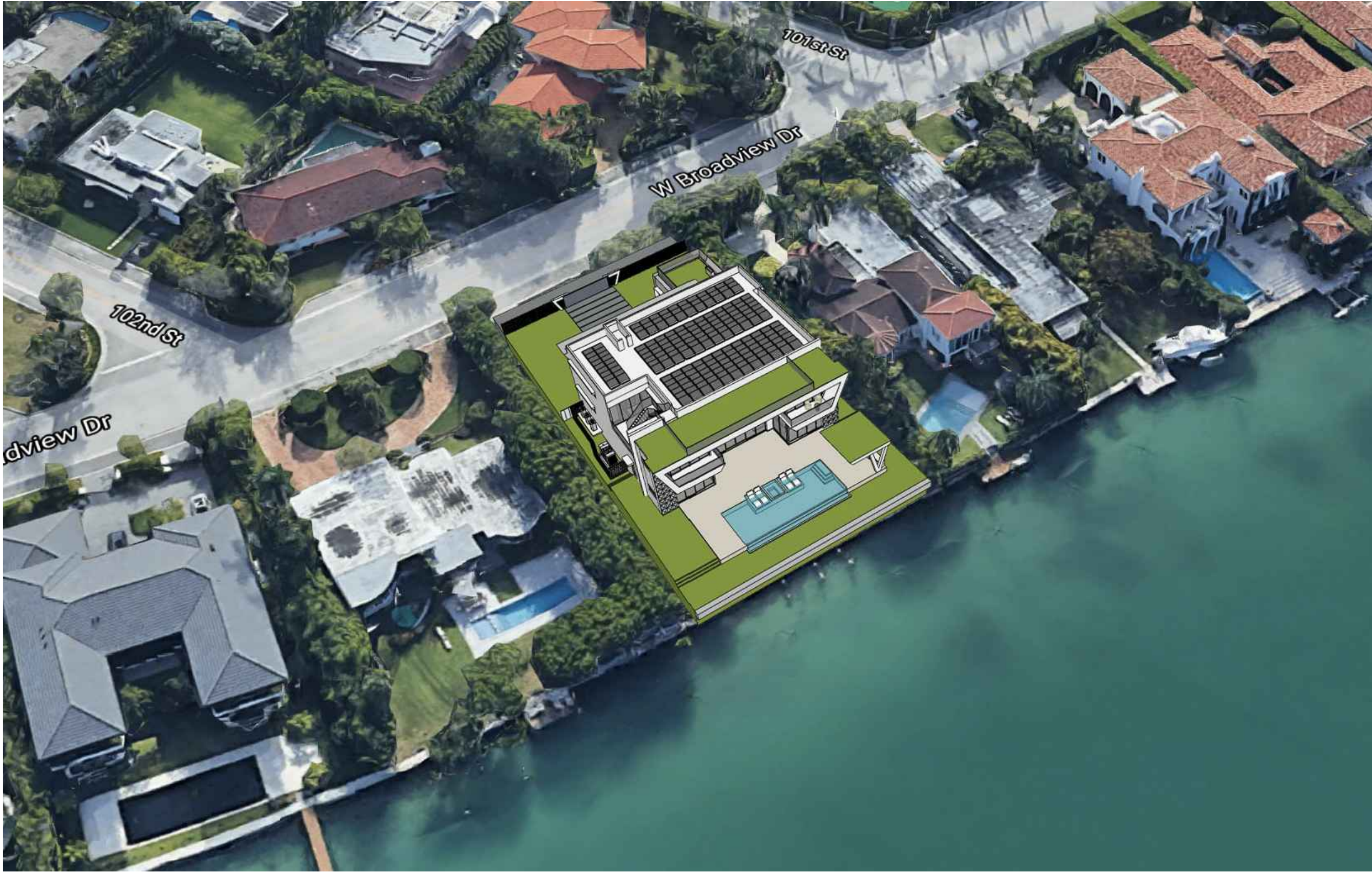
NORTH WEST VIEW
