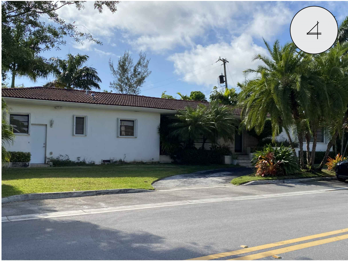
PROPERTY ACROSS THE STREET FROM SUBJECT PROPERTY.
