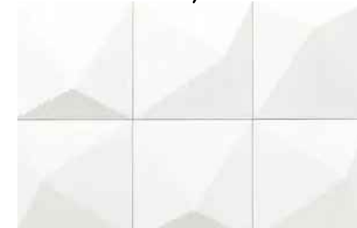
2'-6" X 2'-6" CONCRETE PANELS OVER WALL (PAINTED WHITE)
