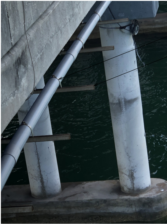
EXAMPLE: U-CLAMP CONNECTION TO CONDUIT
