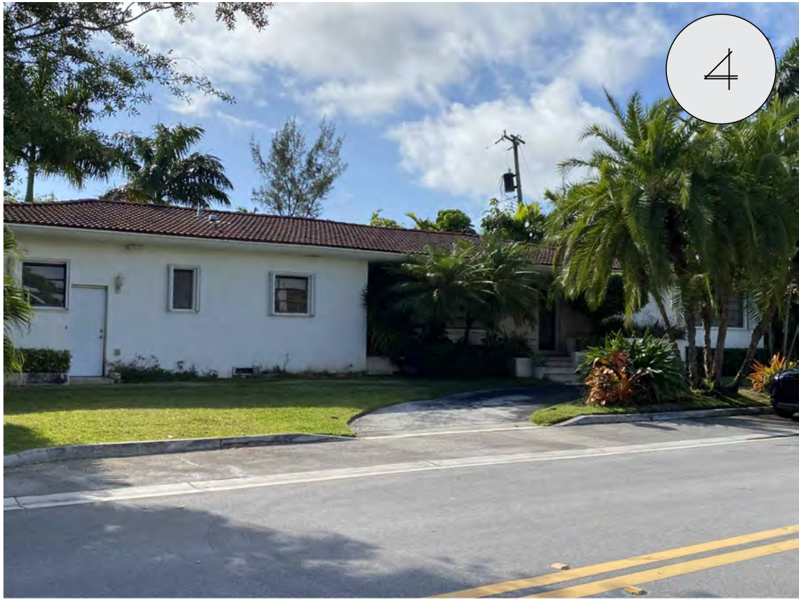
PROPERTY ACROSS THE STREET FROM SUBJECT PROPERTY.
