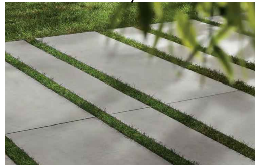
AGREGATE CONCRETE DRIVEWAY WITH GRASS STRIPS
