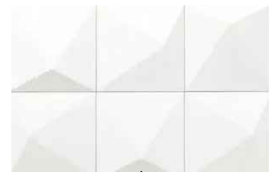
2'-6" X 2'-6" CONCRETE PANELS OVER WALL (PAINTED WHITE)
