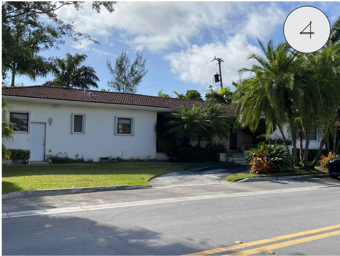
PROPERTY ACROSS THE STREET FROM SUBJECT PROPERTY.
