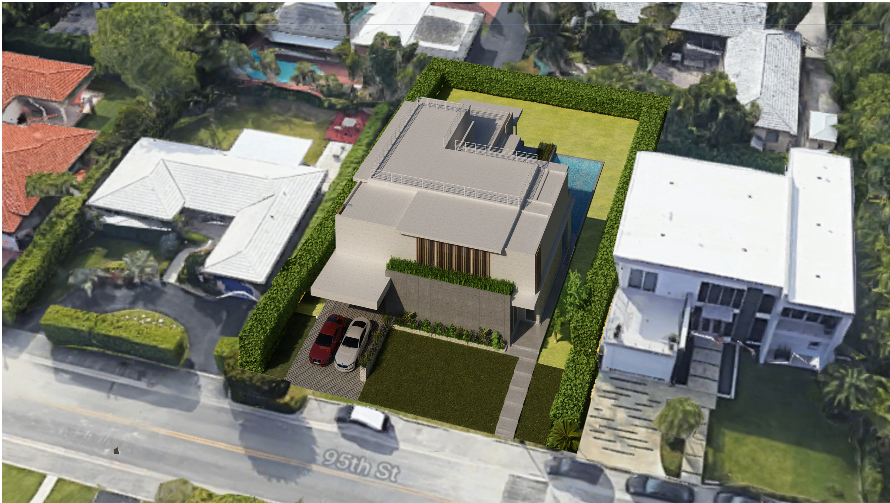
NORTH AERIAL VIEW
