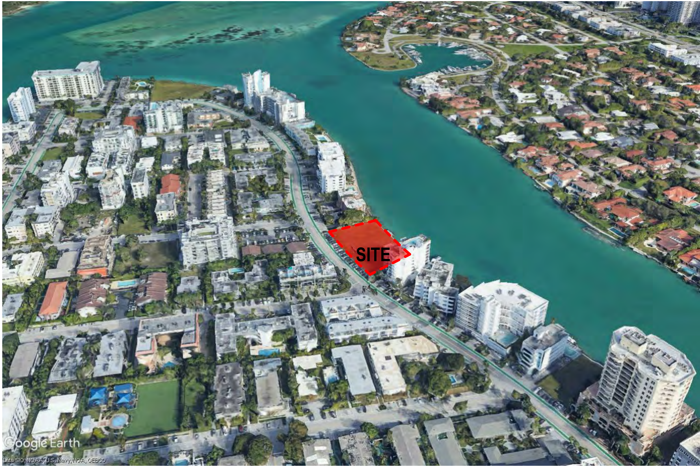
AERIAL VIEW- SOUTH
