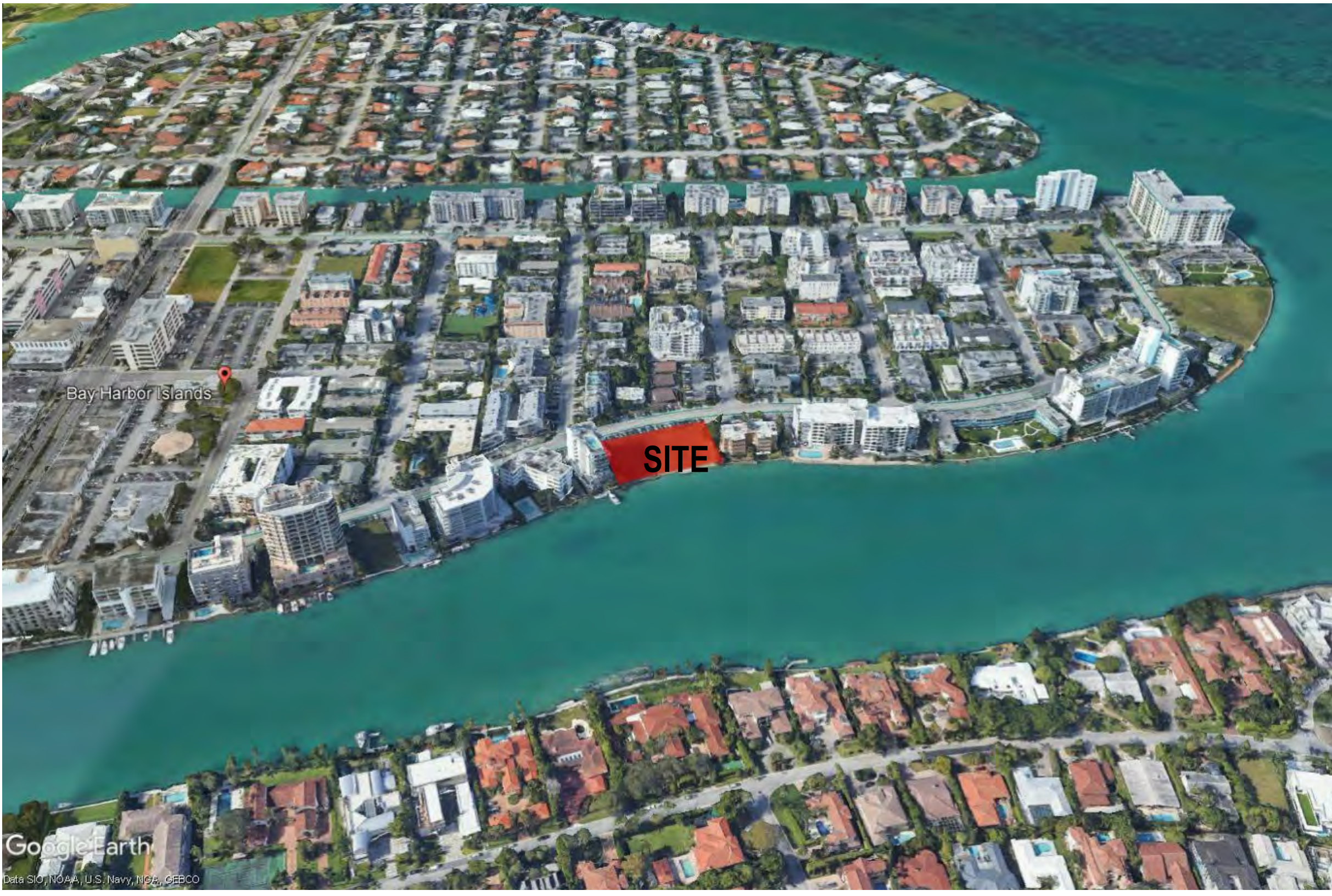
AERIAL VIEW- EAST
