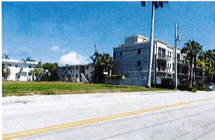
WEST SIDE LOOKING SOUTH
