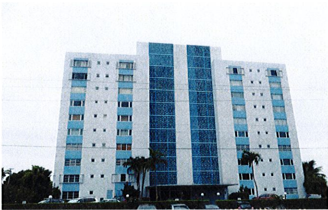
VIEW ACROSS WEST SIDE
