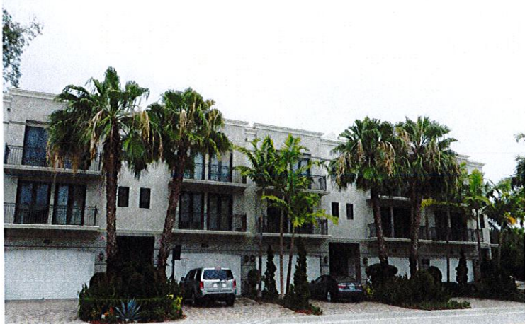
WEST SIDE ADJOINING BUILDING
