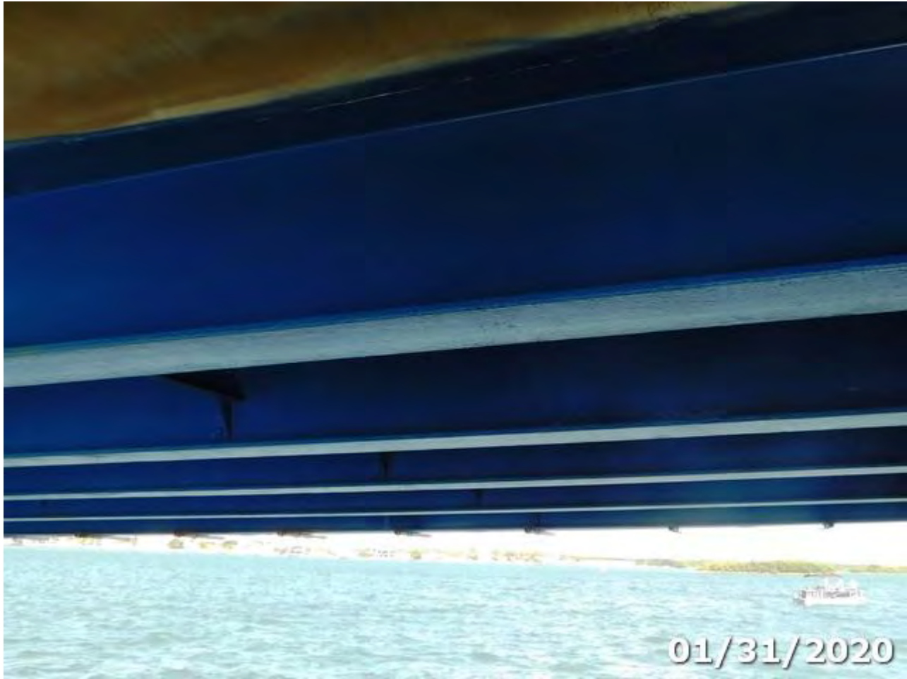
Photo 107-08 (Str Unit Element/Env 107/4: Steel Opn Girder/Beam)
