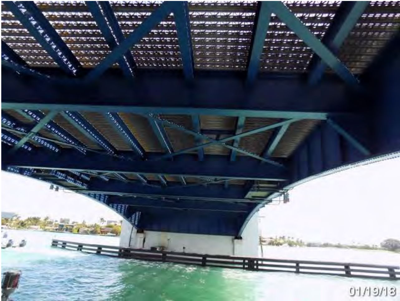
Typical Underside at Main Span - 1/19/2018
