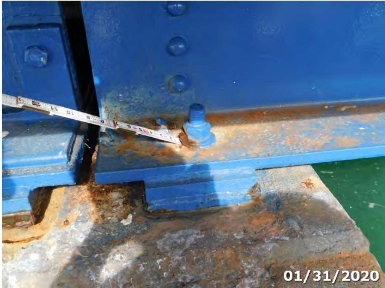
Photo 313-01 (Element/Env 313/4: Fixed Bearing)
