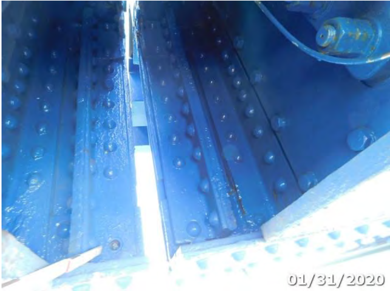
Photo 107-03 (Str Unit 0 Element/Env 107/4: Steel Opn Girder/Beam)
