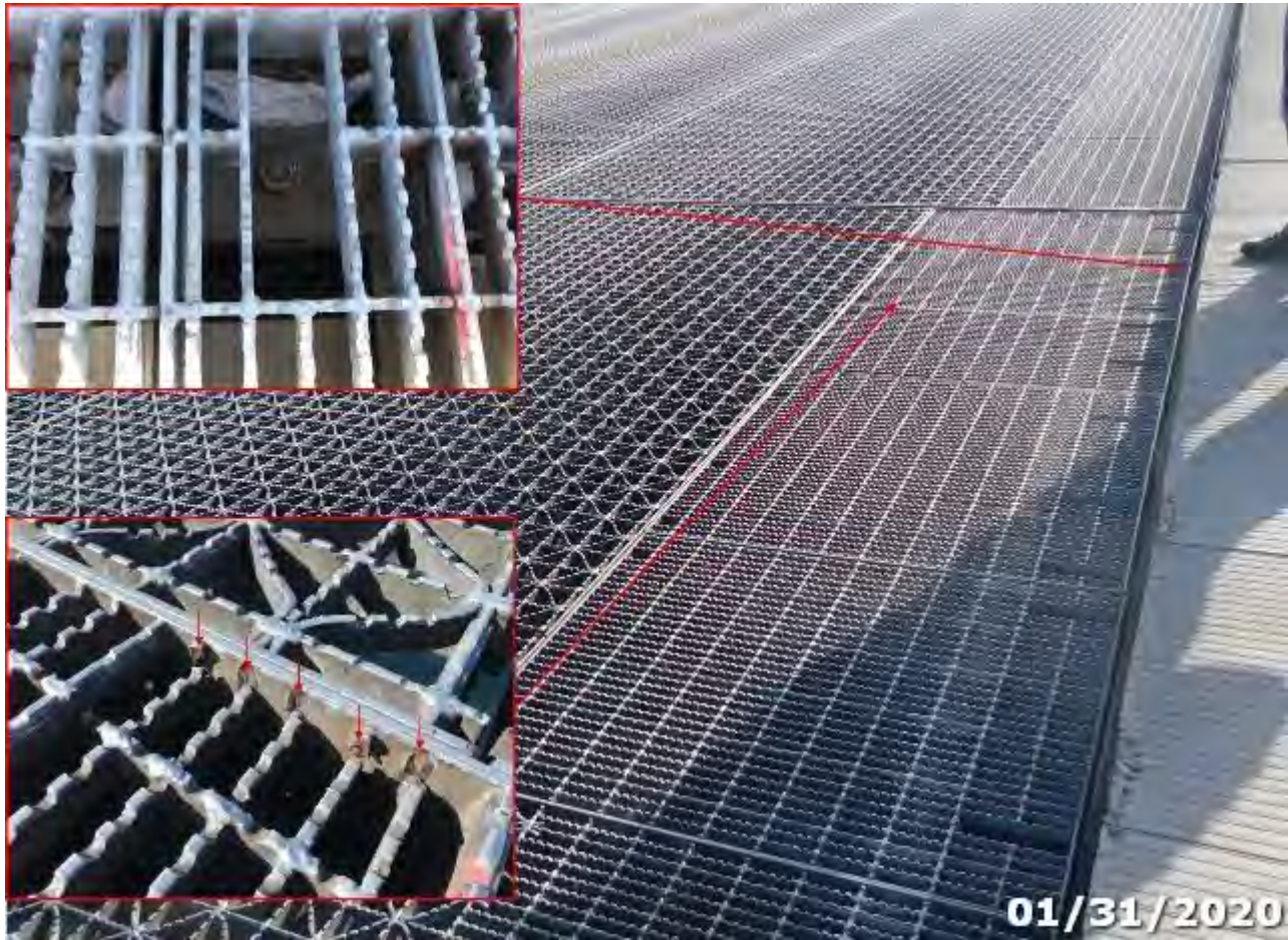
Photo 28-01 Element/Env 28/4: Steel Deck - Open Grid
