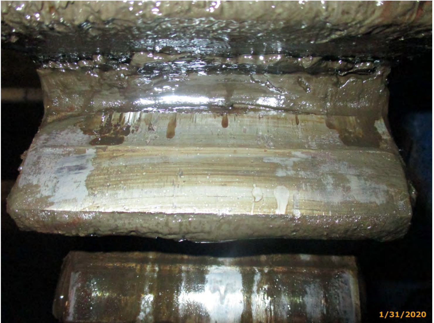
Photo 8540-M04 (Element/Env 8540/4: Open Gearing)
