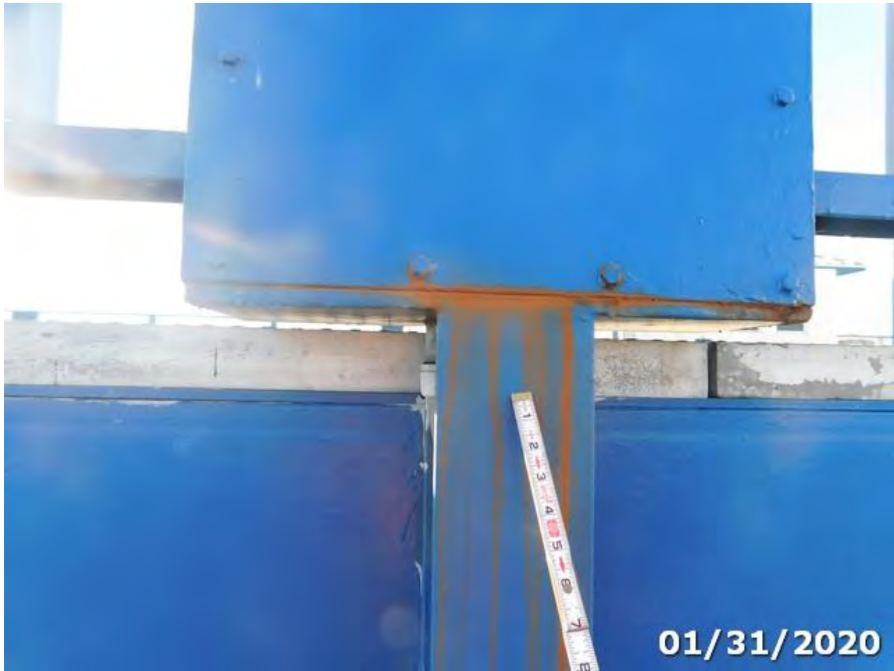
Photo 330-01 (Element/Env 330/4: Metal Bridge Railing)
