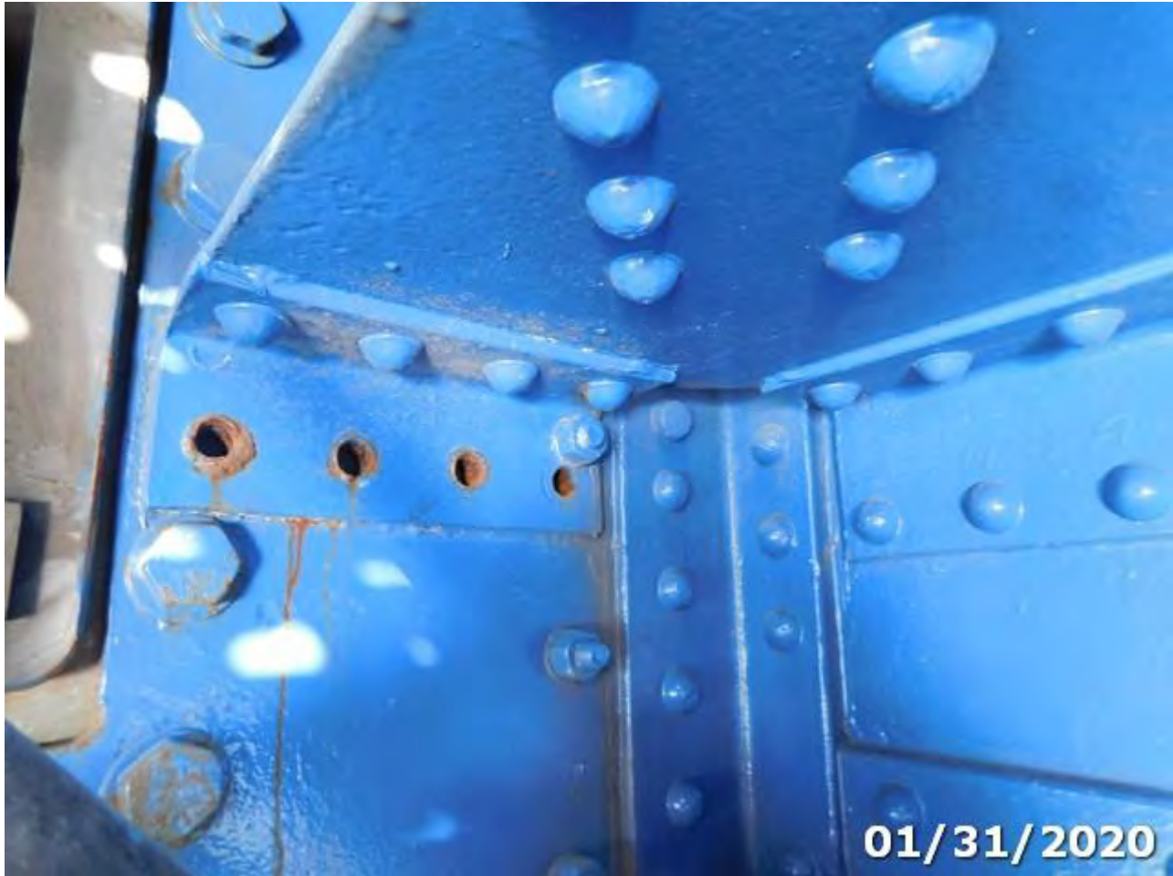
Photo 152-07 (Element/Env 152/4: Steel Floor Beam)
