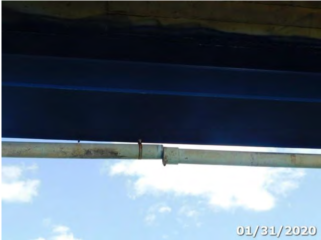
Photo 12-06 (Element/Env 12/4: Re Concrete Deck)
