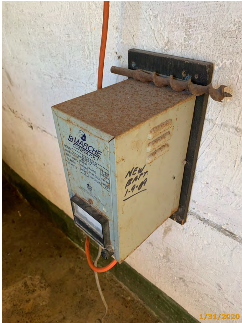
Photo 8545-E02 (Element/Env 8545/4: Emergency Drive)
