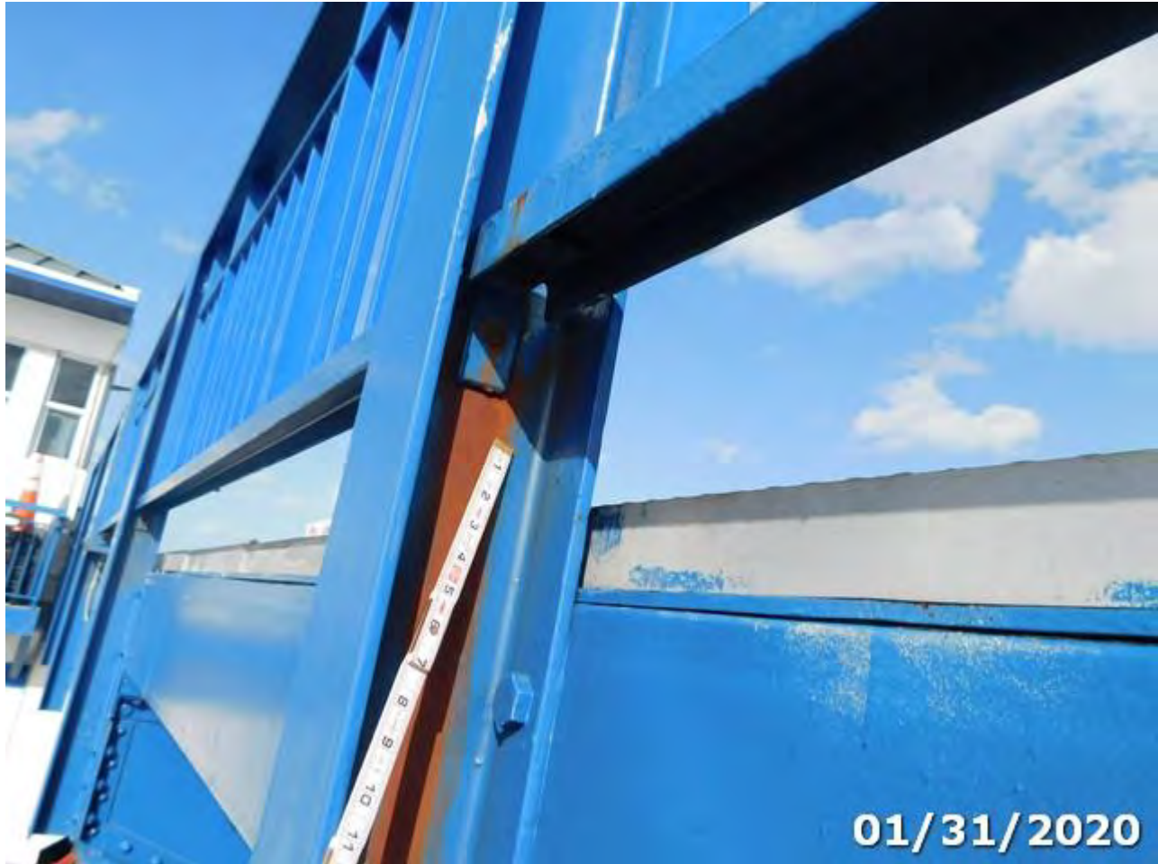
Photo 330-02 (Element/Env 330/4: Metal Bridge Railing)
