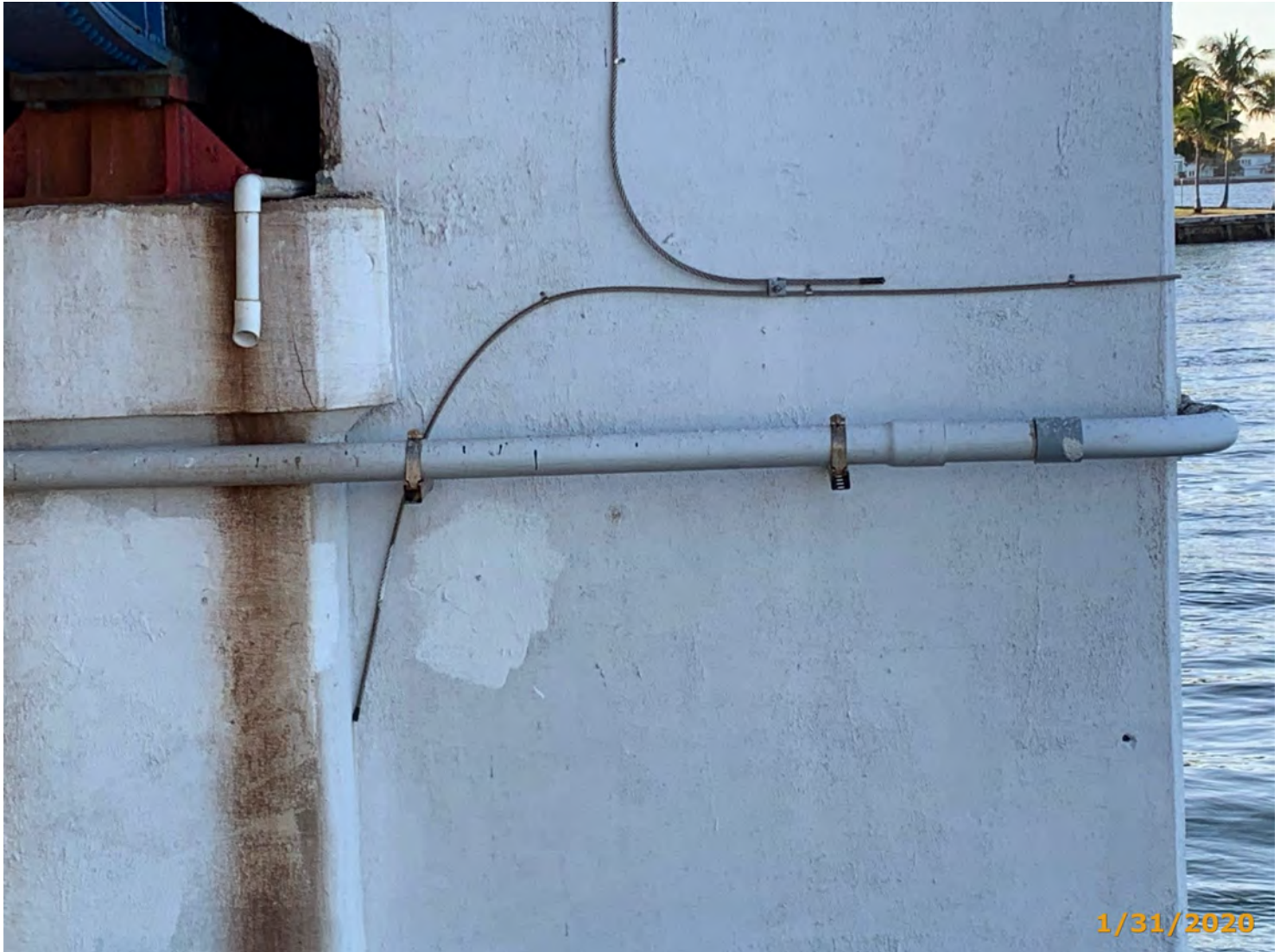
Photo 8572-E05 (Element/Env 8572/4:Conduit & Junction Box)
