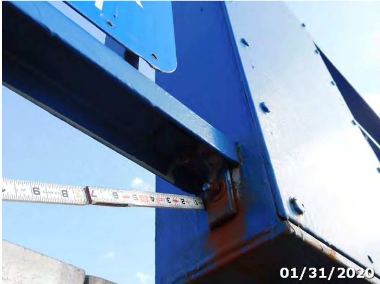
Photo 330-03 (Element/Env 330/4: Metal Bridge Railing)
