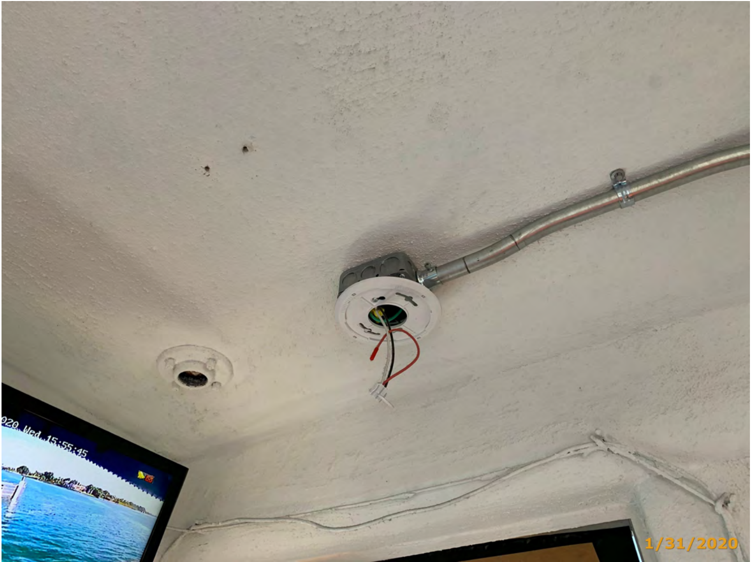
Photo 8572-E02 (Element/Env 8572/4:Conduit & Junction Box)
