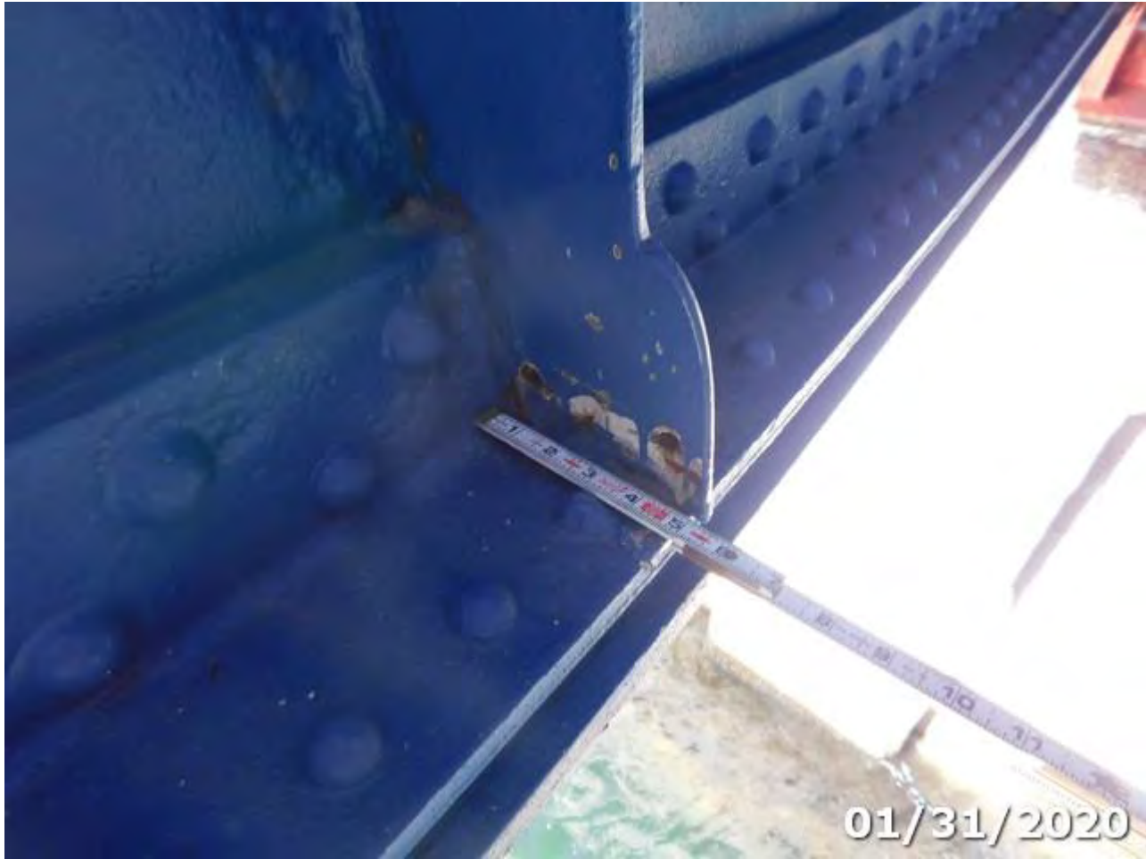
Photo 107-05 (Str Unit 0 Element/Env 107/4: Steel Opn Girder/Beam)
