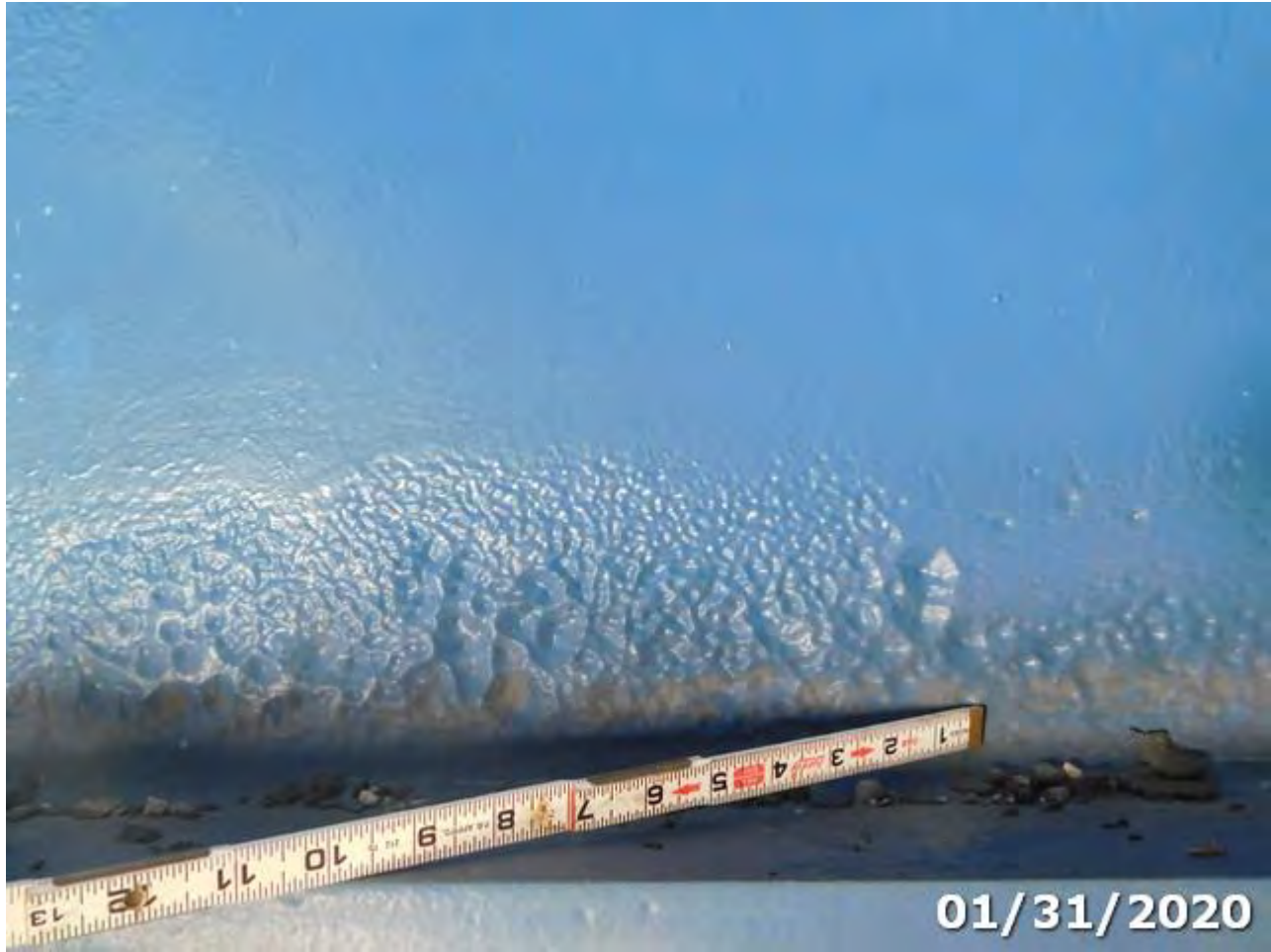
Photo 152-04 (Element/Env 152/4: Steel Floor Beam)
