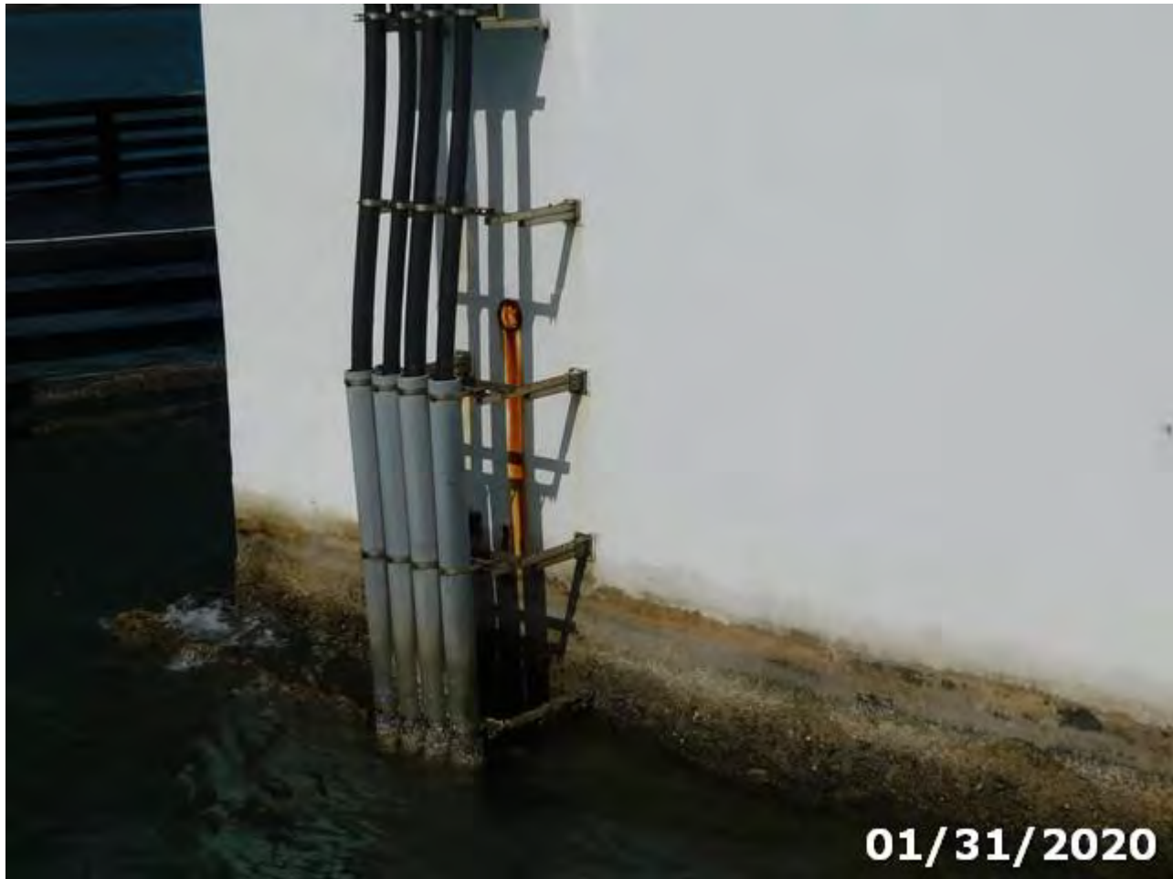
Photo 210-07 (Element/Env 210/4: Re Conc Pier Wall)
