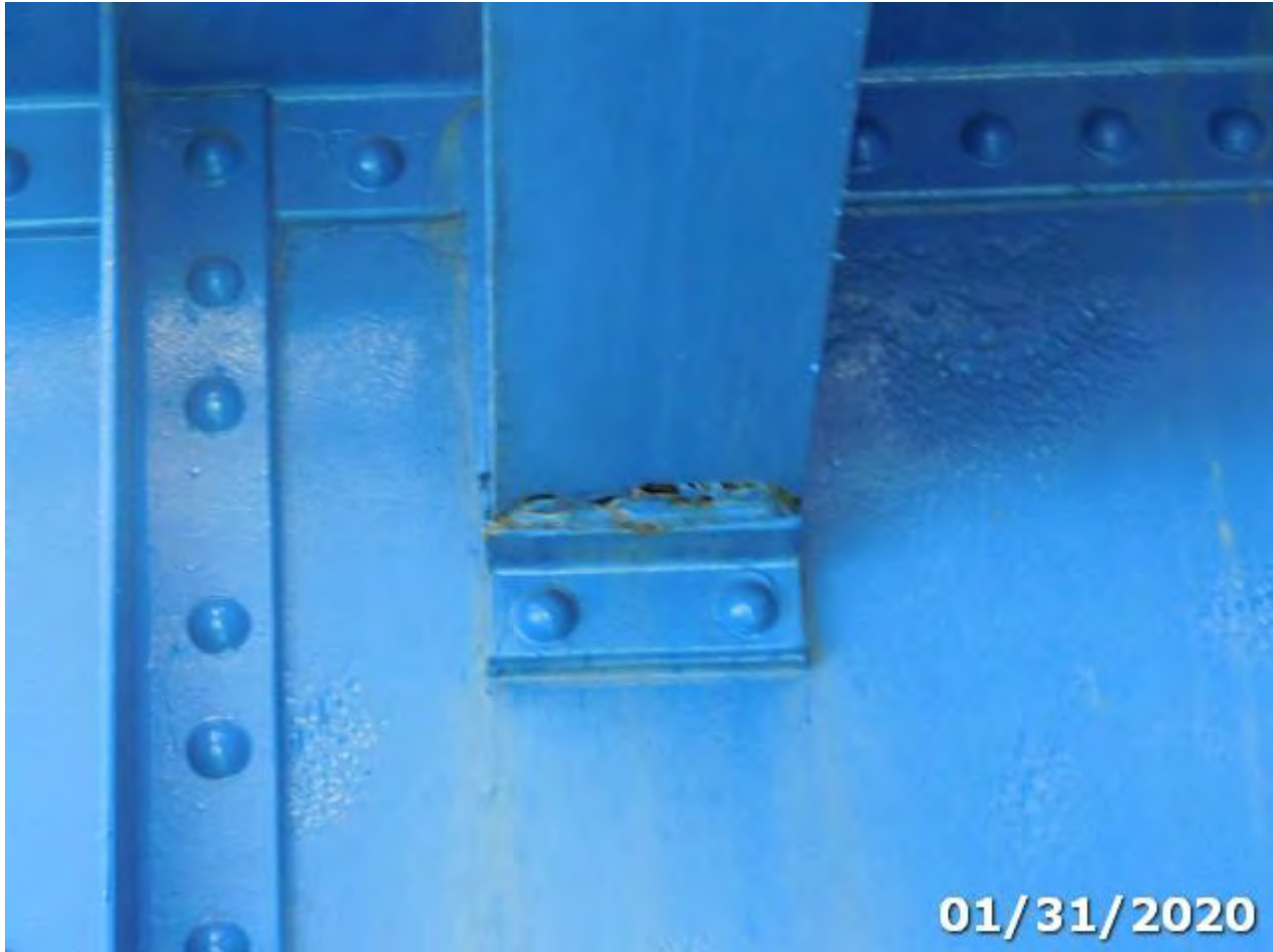
Photo 113-02 (Element/Env 113/4: Steel Stringer)
