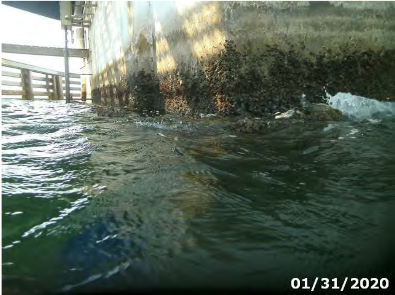
Photo 210-05 (Element/Env 210/4: Re Conc Pier Wall)
