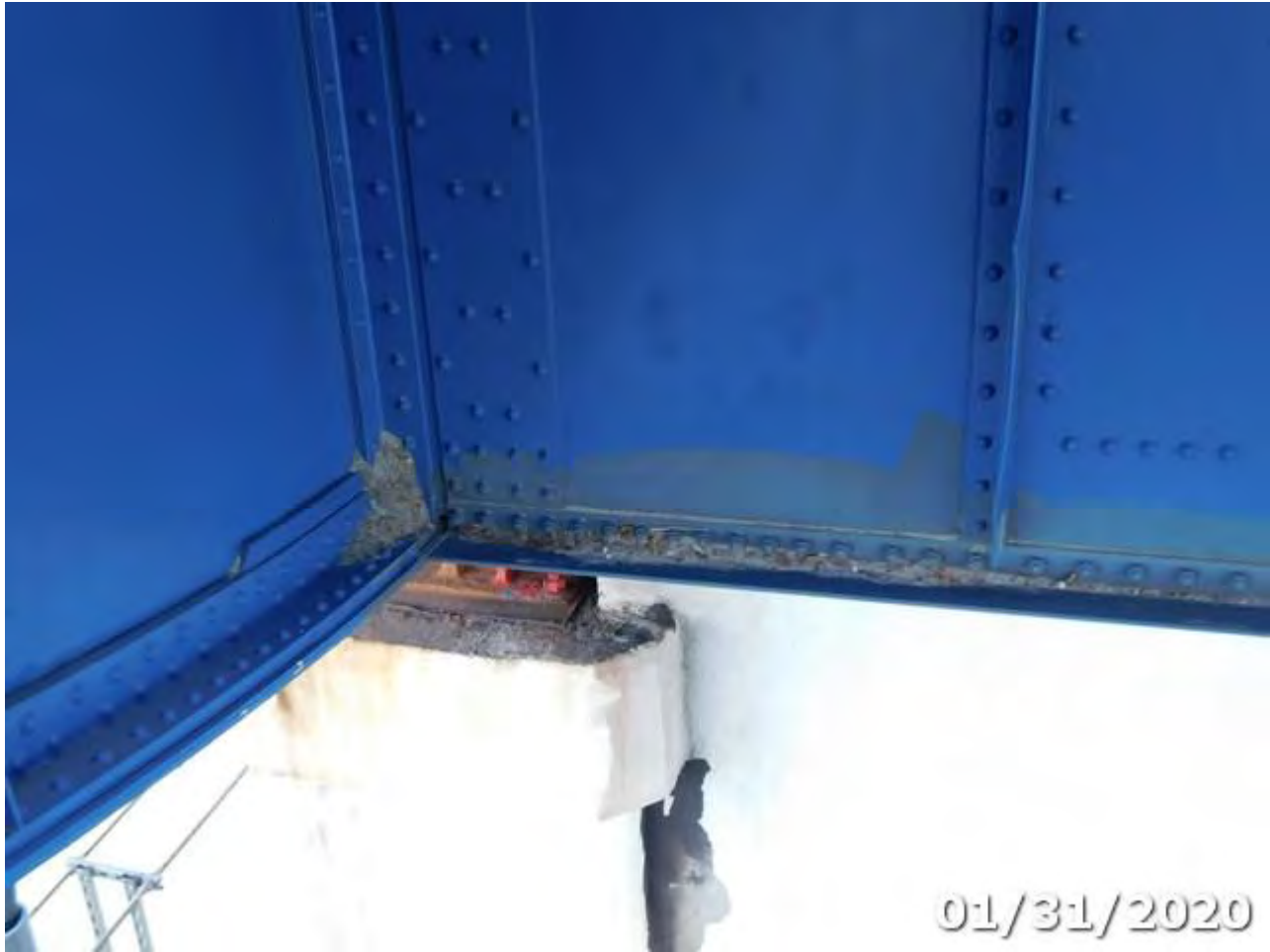
Photo 152-03 (Element/Env 152/4: Steel Floor Beam)
