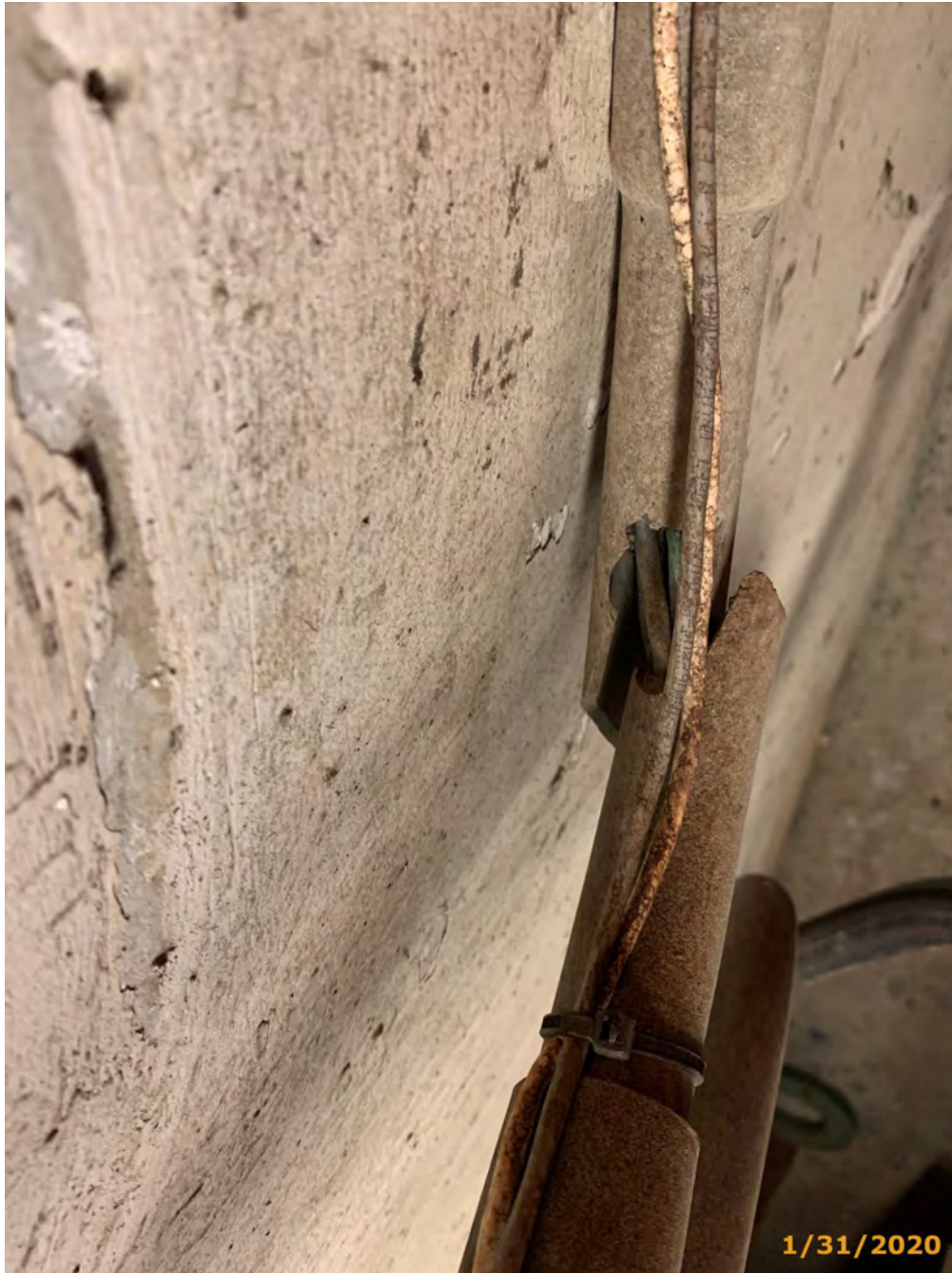
Photo 8572-E07 (Element/Env 8572/4:Conduit & Junction Box)
