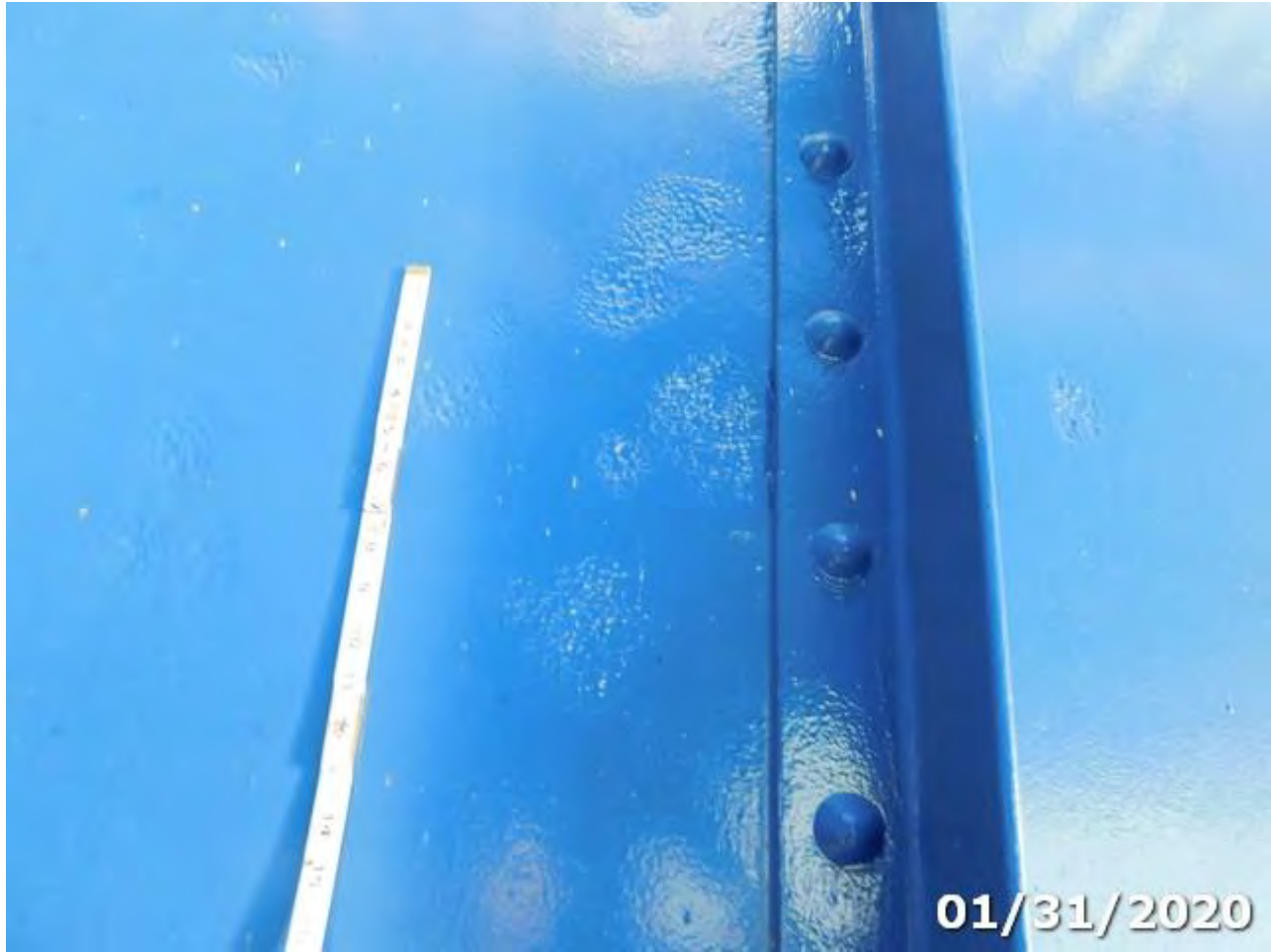
Photo 107-02 (Str Unit 0 Element/Env 107/4: Steel Opn Girder/Beam)
