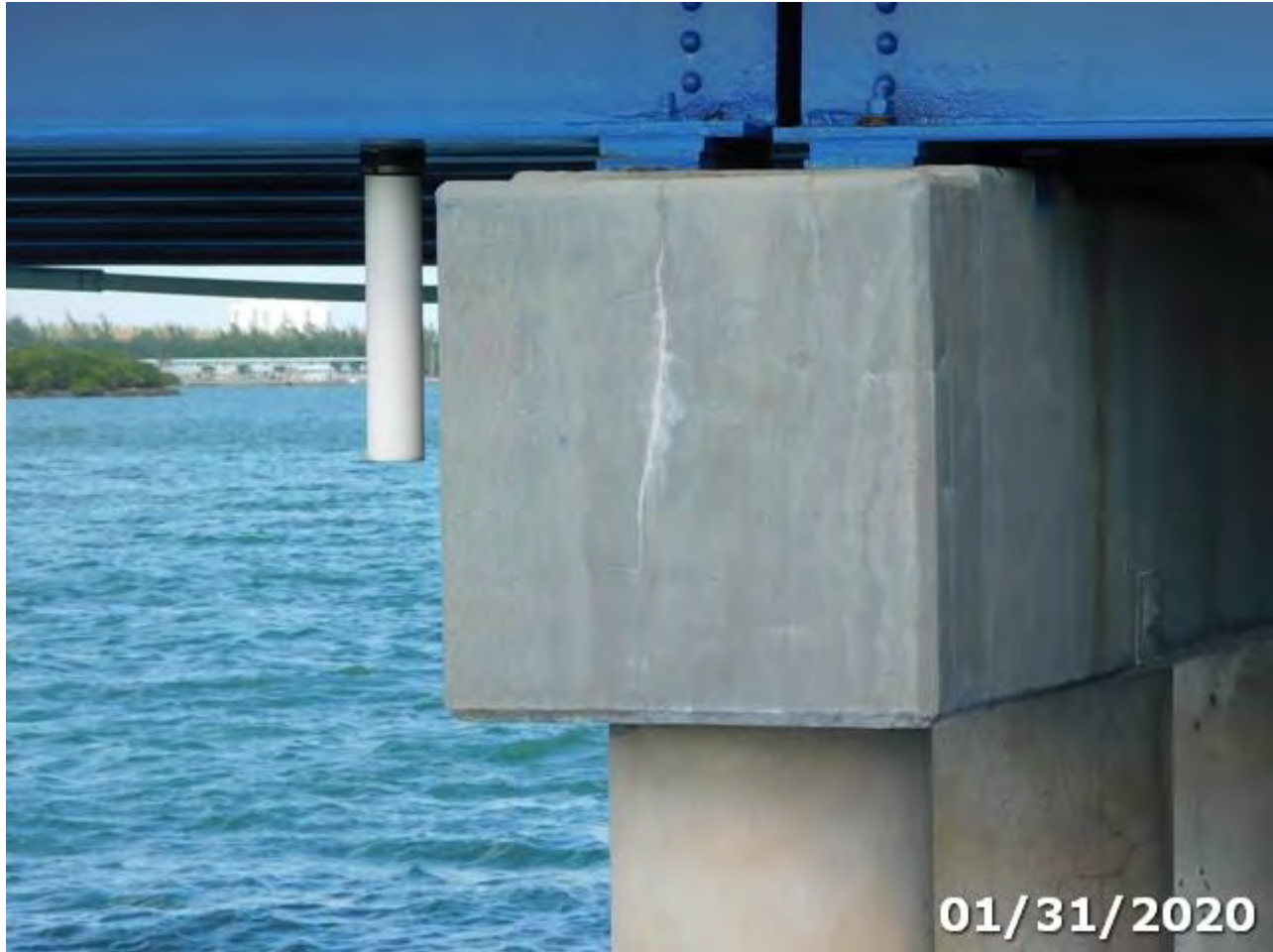
Photo 234-01 (Element/Env 234/4: Re Conc Pier Cap)
