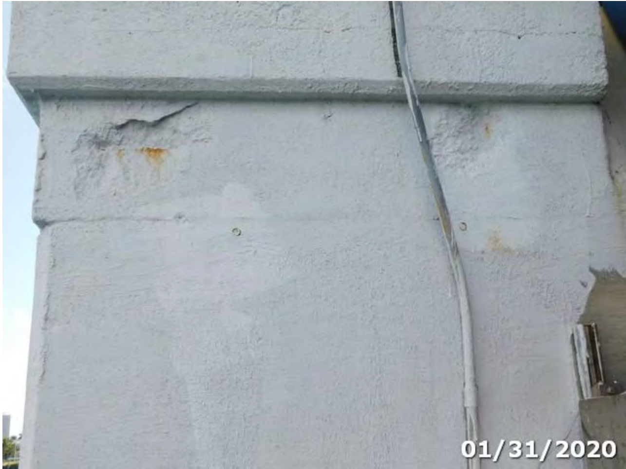
Photo 210-04 (Element/Env 210/4: Re Conc Pier Wall)
