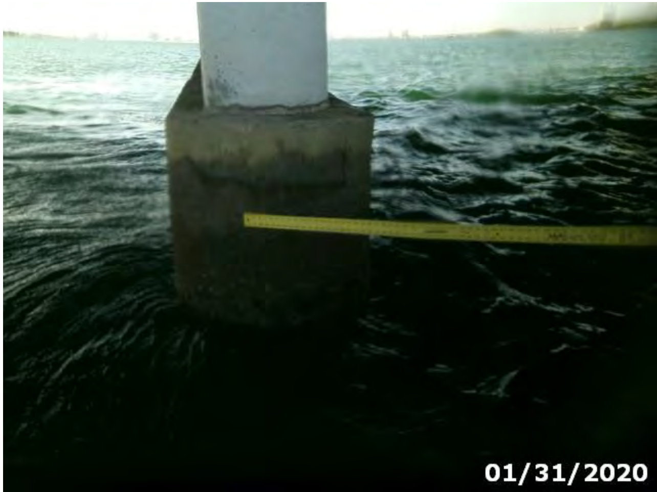
Photo 220-01 (Element/Env 220/4: Re Conc Pile Cap/Ftg)
