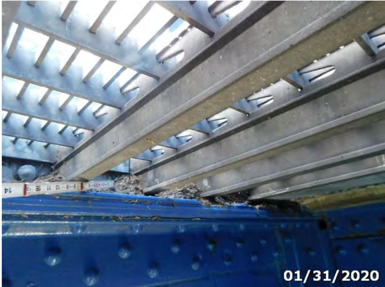
Photo 107-01 (Str Unit 0 Element/Env 107/4: Steel Opn Girder/Beam)
