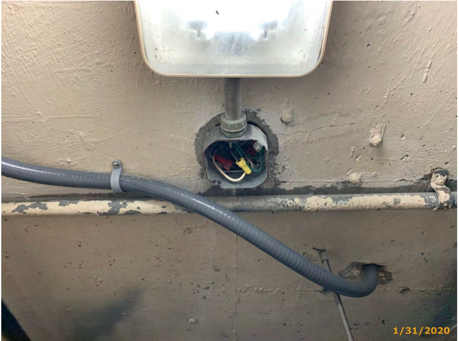
Photo 8572-E03 (Element/Env 8572/4:Conduit & Junction Box)
