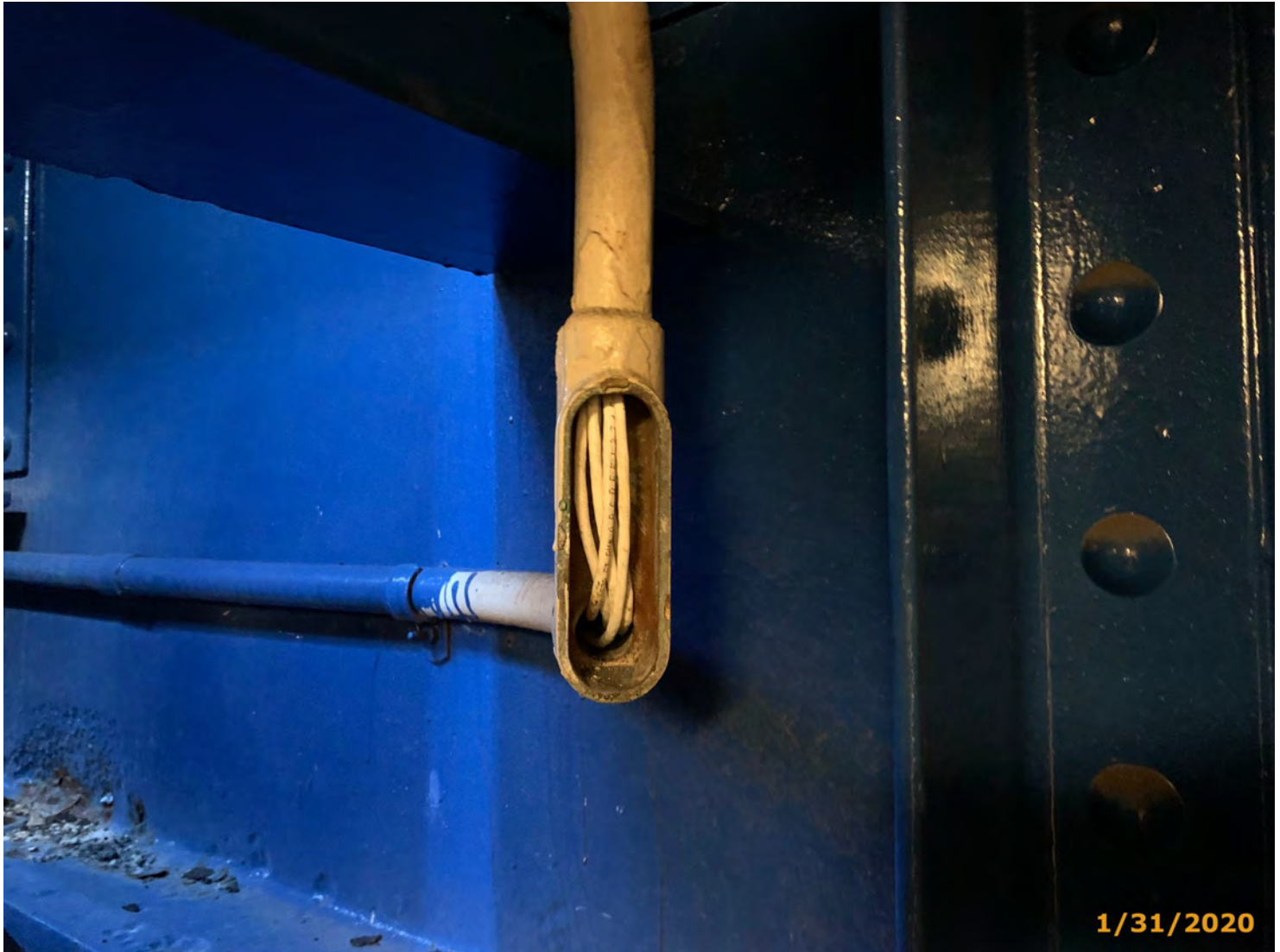
Photo 8572-E01 (Element/Env 8572/4: Conduit & Junction Box)
