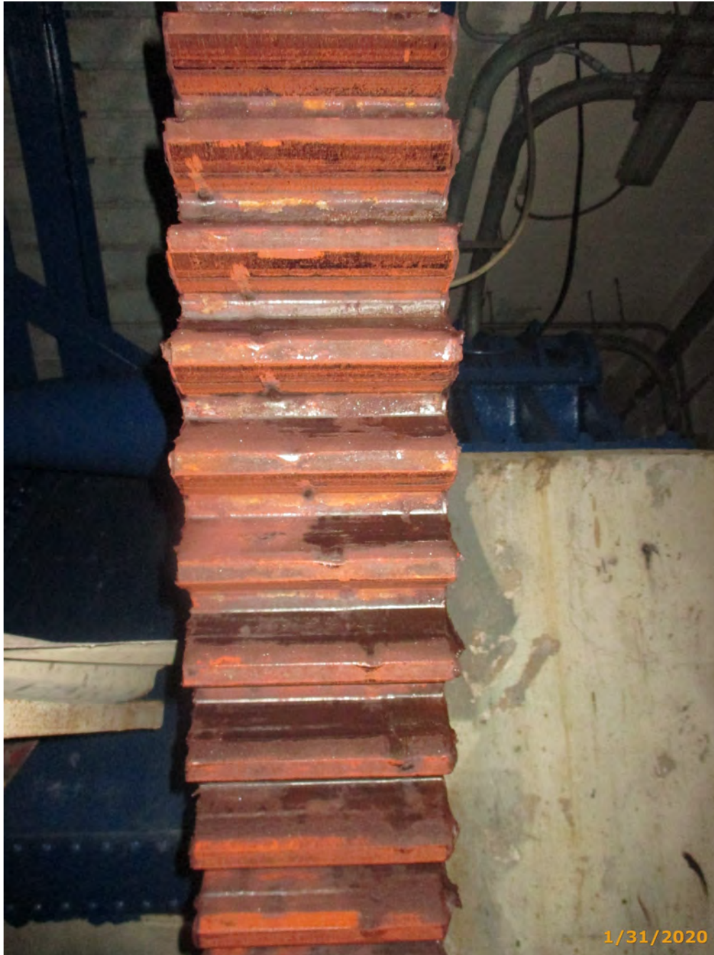
Photo 8540-M03 (Element/Env 8540/4: Open Gearing)
