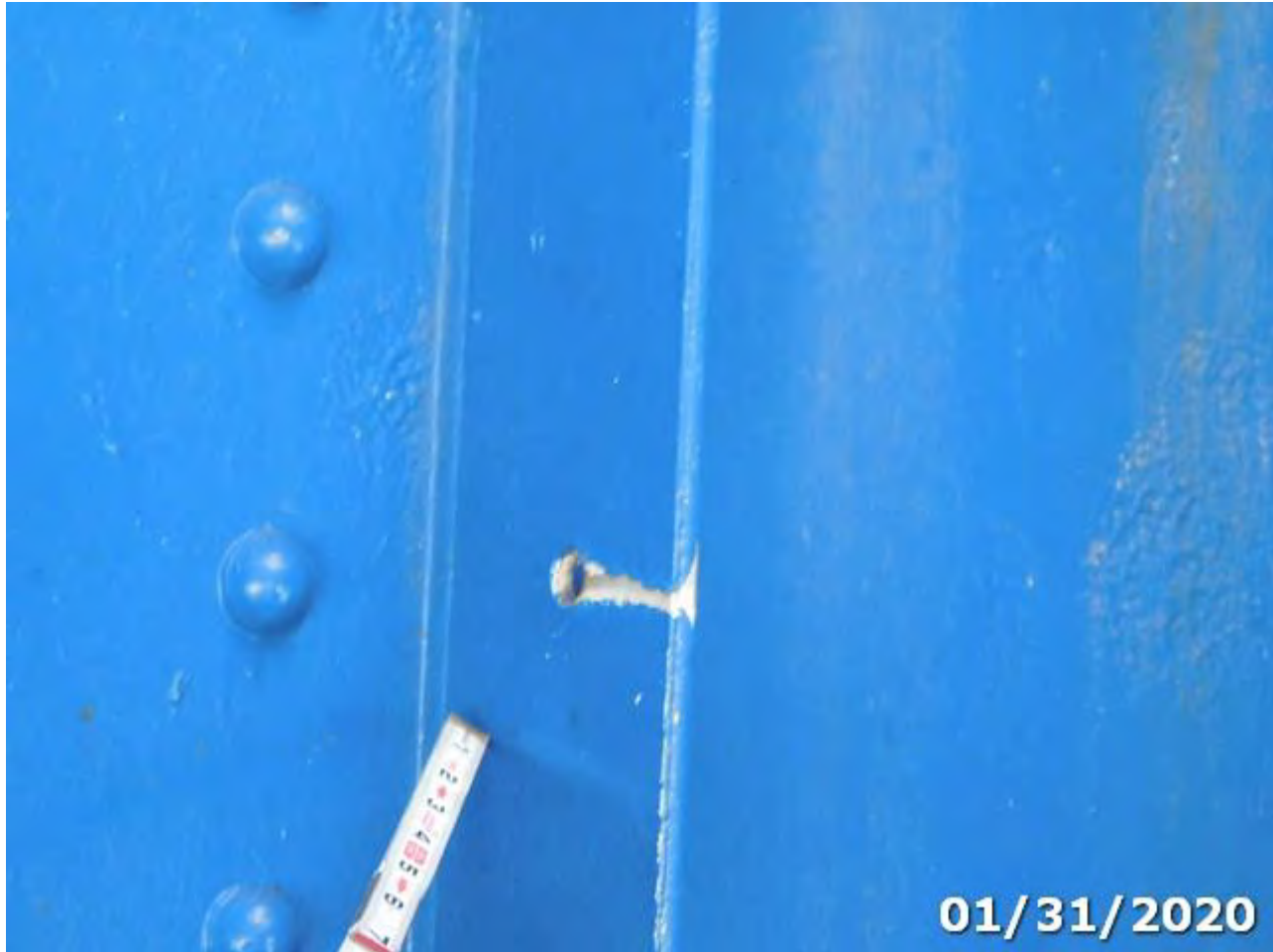
Photo 152-01 (Element/Env 152/4: Steel Floor Beam)
