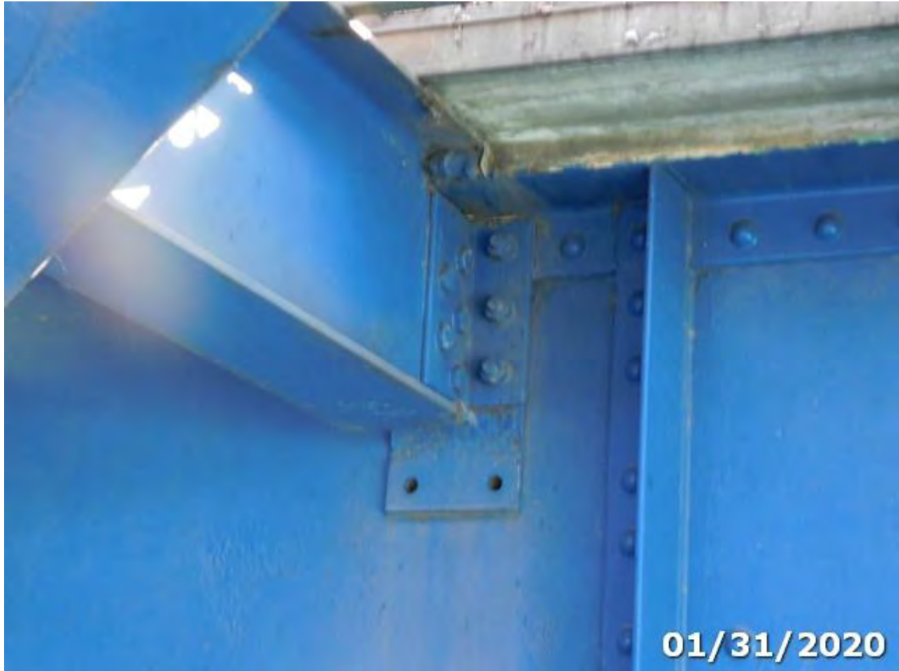
Photo 113-03 (Element/Env 113/4: Steel Stringer)
