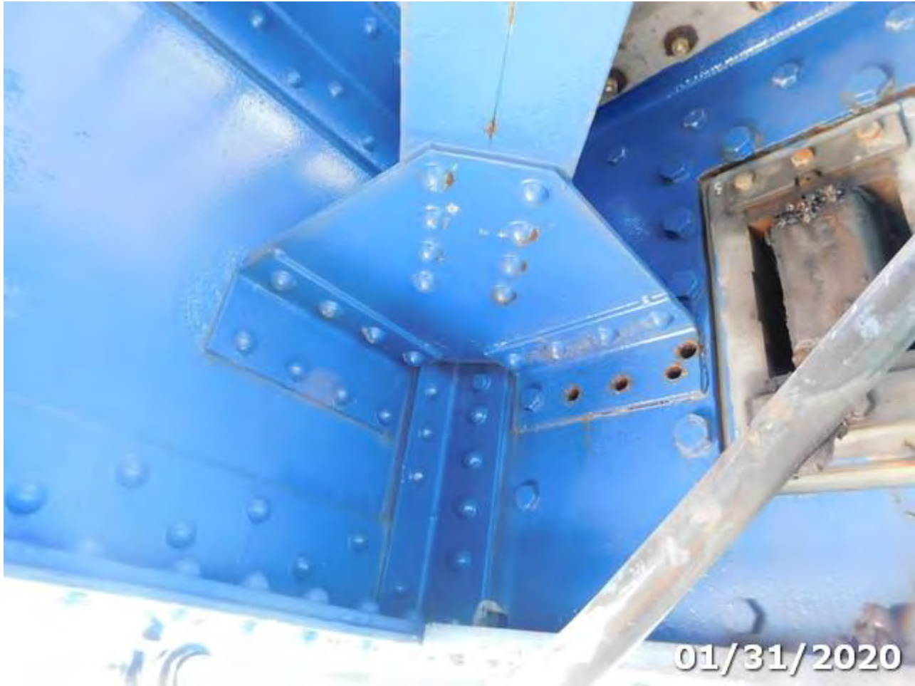
Photo 152-08 (Element/Env 152/4: Steel Floor Beam)
