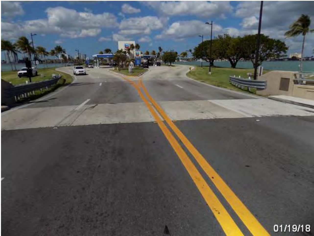
West Approach Looking West - 1/19/2018
