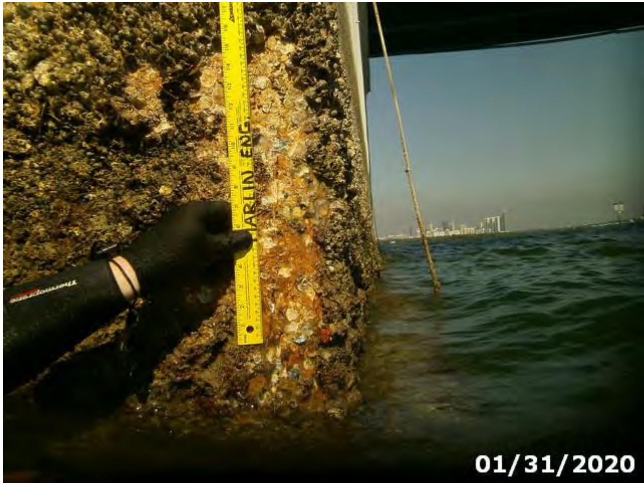
Photo 210-09 (Element/Env 210/4: Re Conc Pier Wall)
