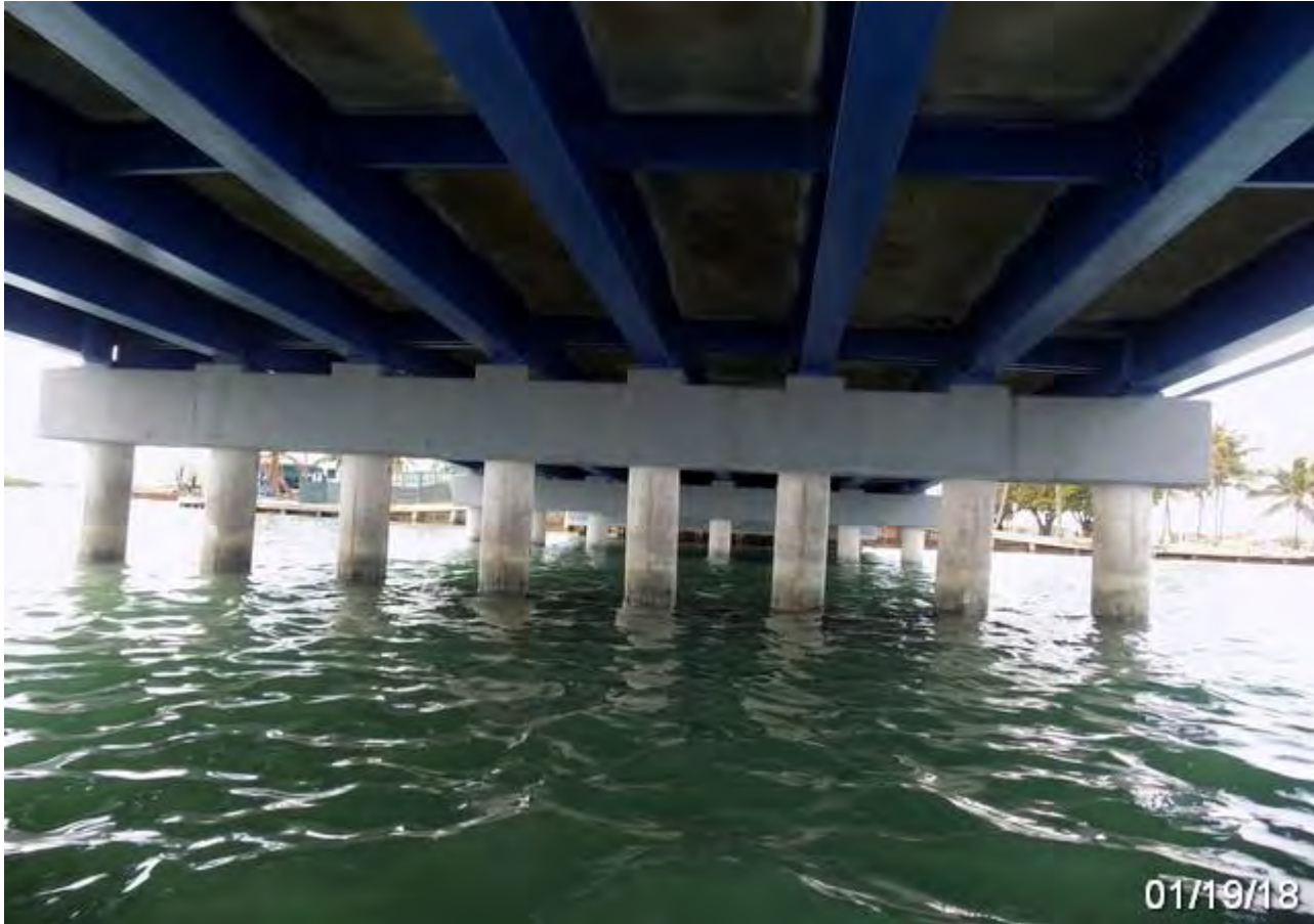
Typical Underside at Approach spans - 1/19/2018
