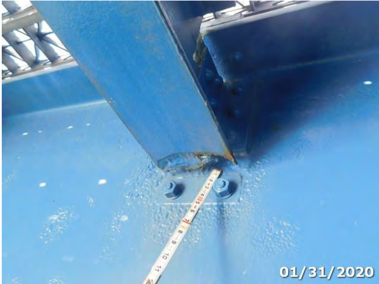
Photo 113-01 (Element/Env 113/4: Steel Stringer)
