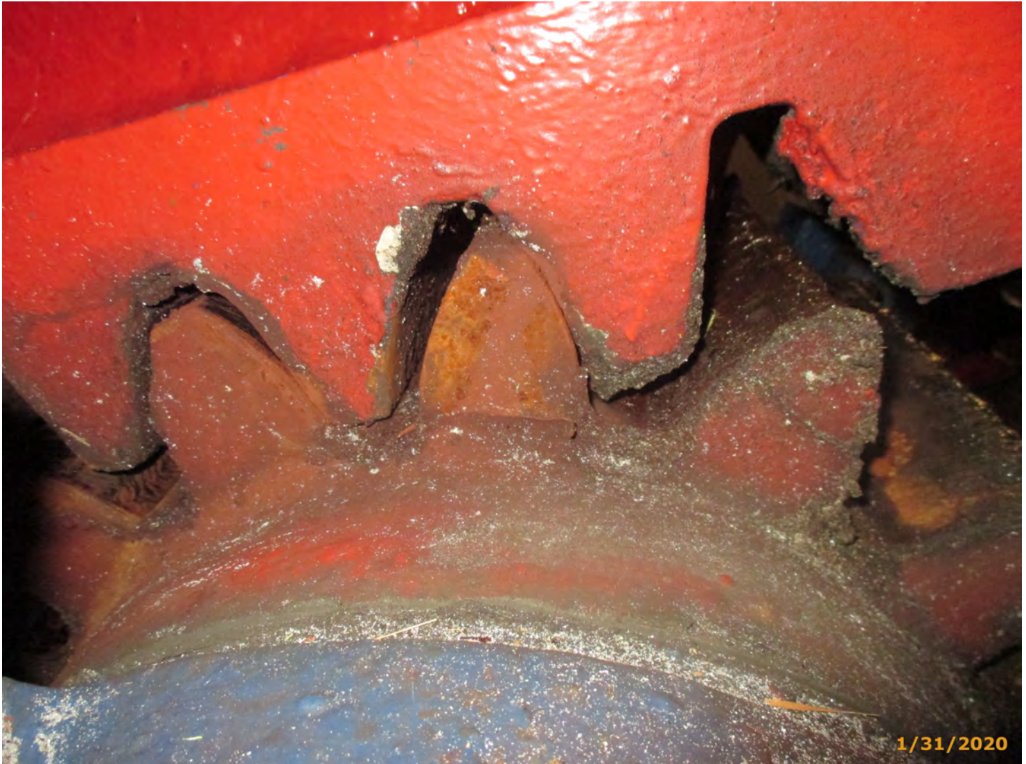
Photo 8540-M05 (Element/Env 8540/4: Open Gearing)
