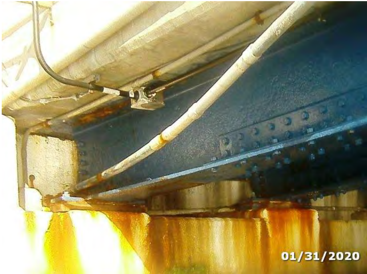
Photo 313-02 (Element/Env 313/4: Fixed Bearing)
