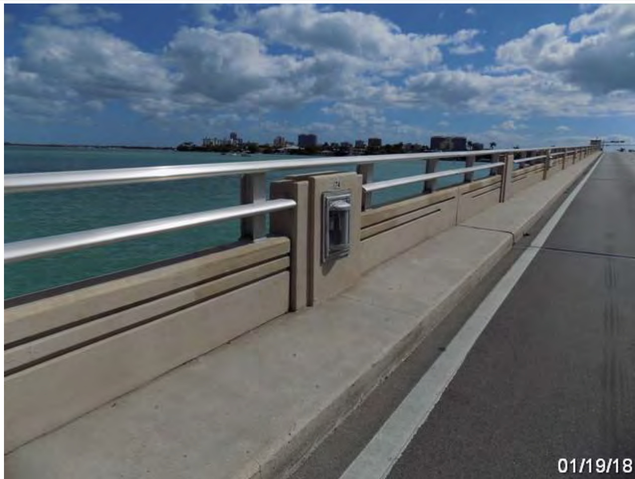
Typical Bridge Rail at Approach spans - 1/19/2018
