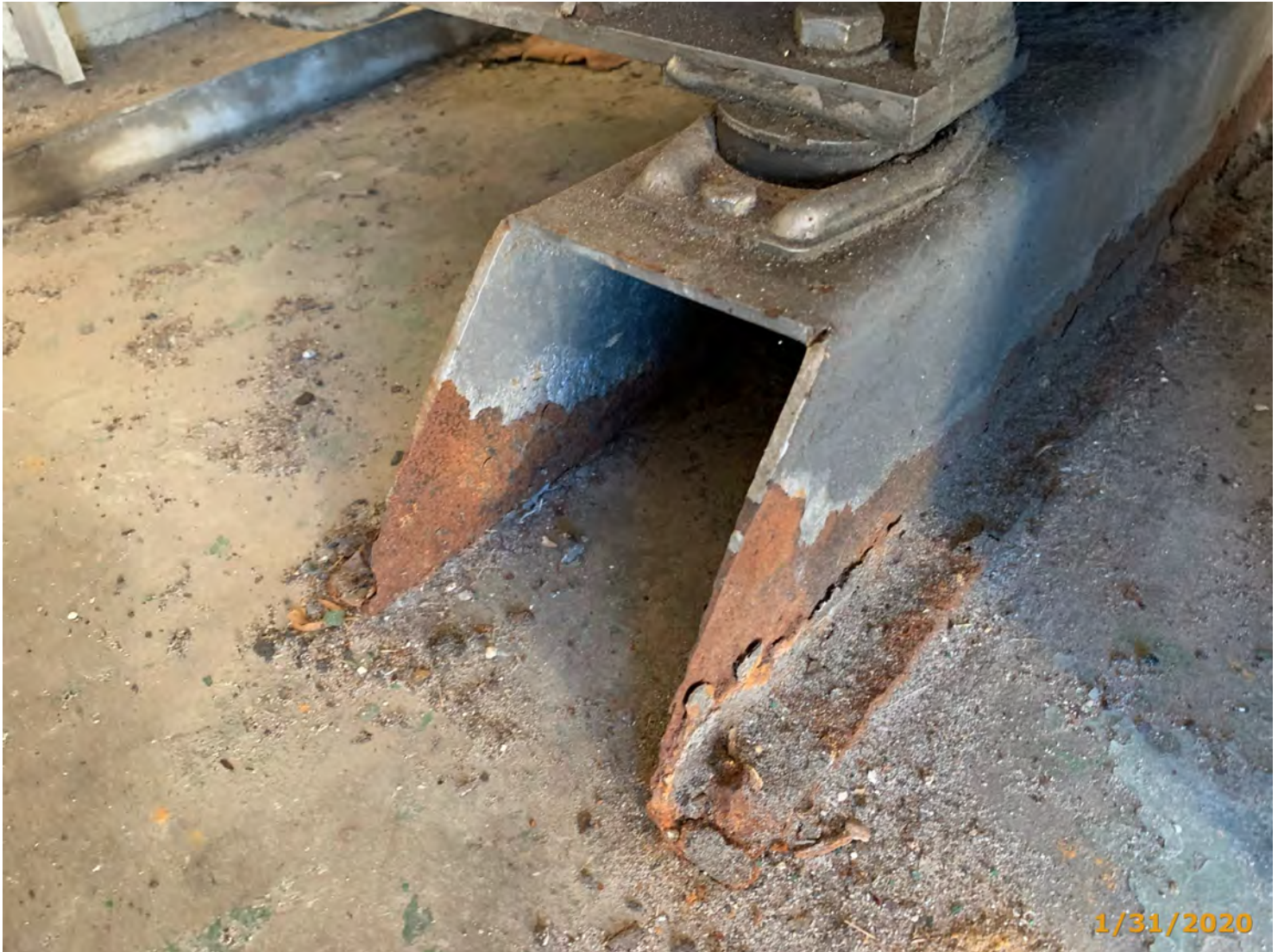
Photo 8545-E03 (Element/Env 8545/4: Emergency Drive)
