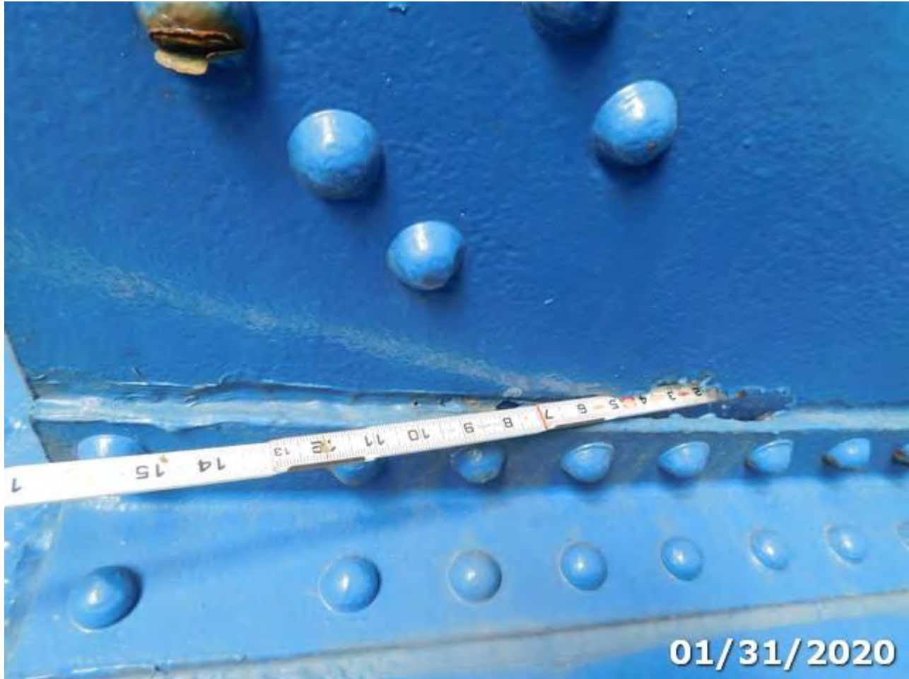
Photo 152-05 (Element/Env 152/4: Steel Floor Beam)
