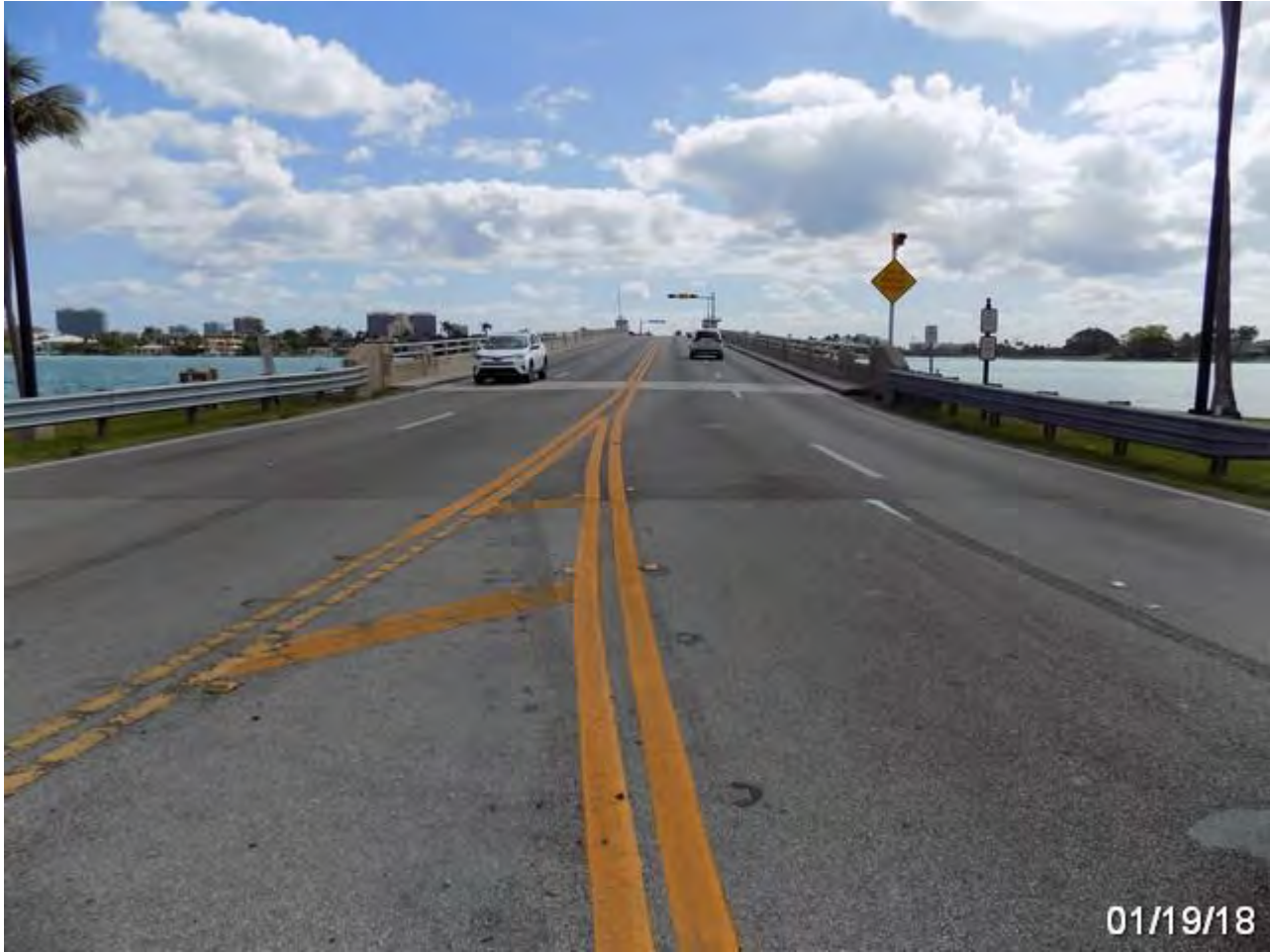
West Approach Looking East - 1/19/2018
