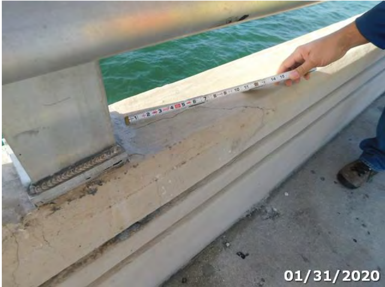
Photo 333-01 (Element/Env 333/4: Other Bridge Railing)
