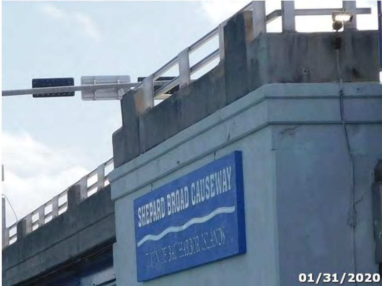
Photo 210-01 (Element/Env 210/4: Re Conc Pier Wall)
