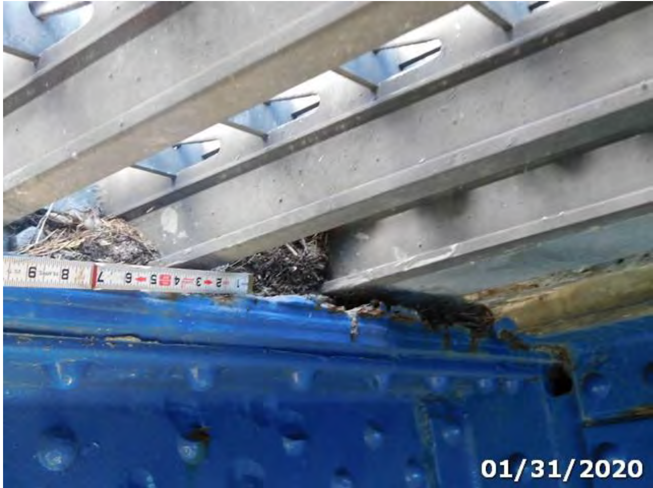
Photo 107-04 (Str Unit 0 Element/Env 107/4: Steel Opn Girder/Beam)
