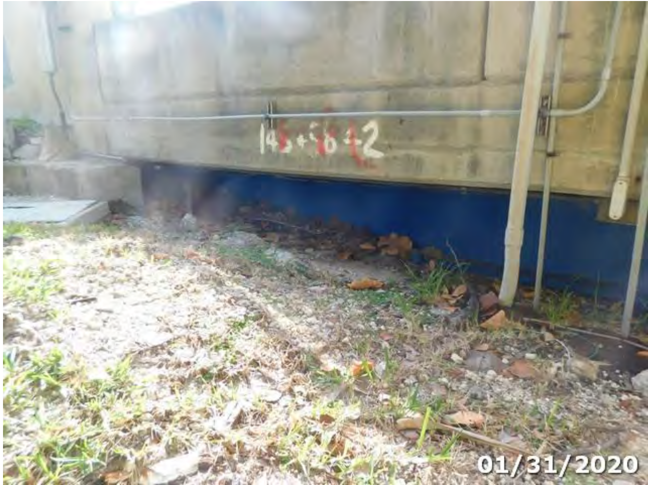
Photo 107-07 (Str Unit 1 Element/Env 107/4: Steel Opn Girder/Beam)
