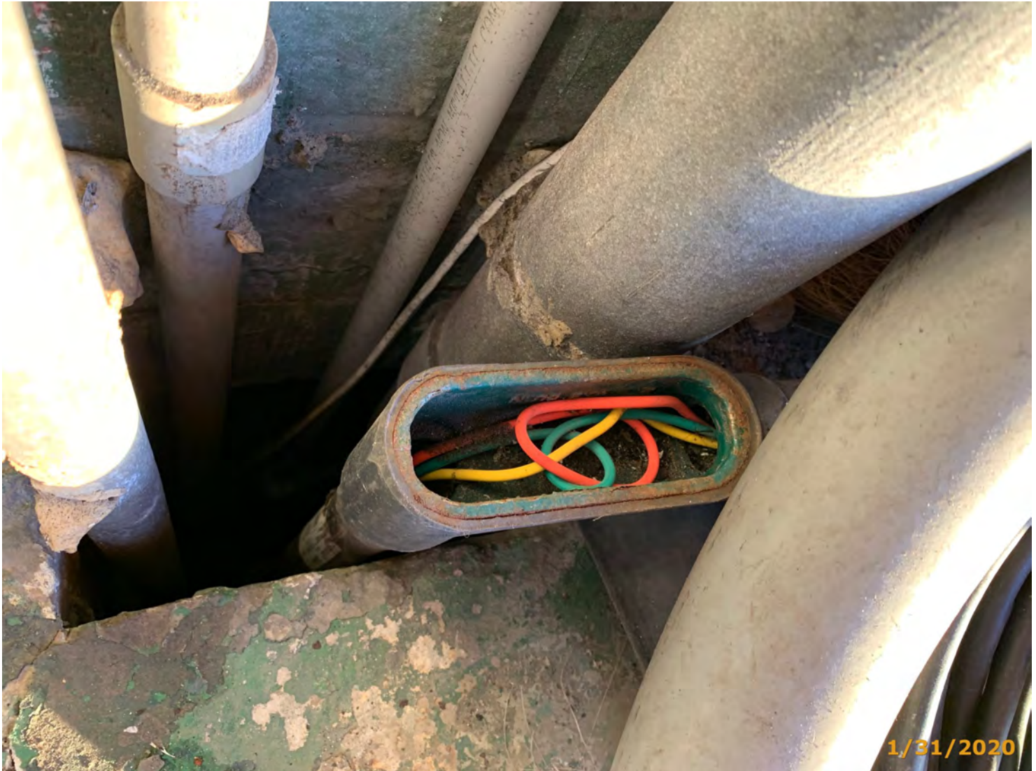
Photo 8572-E06 (Element/Env 8572/4:Conduit & Junction Box)
