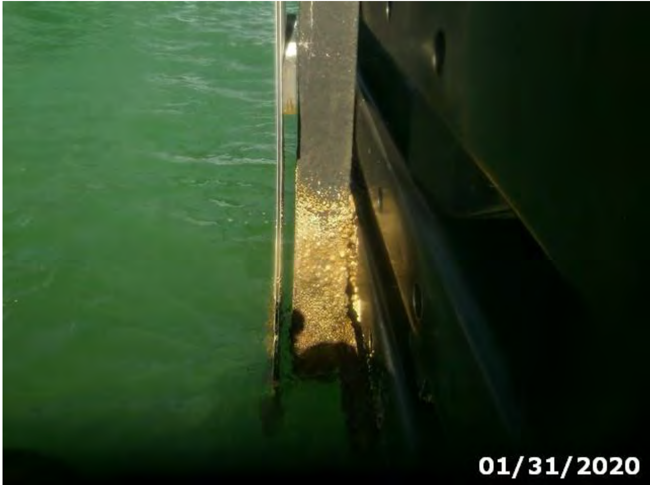
Photo 8390-01 (Element/Env 8390/4: Other Fender/Dolphin)
