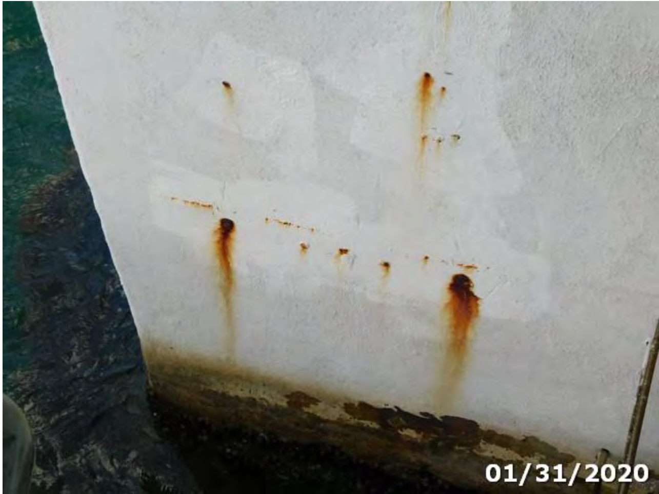
Photo 210-06 (Element/Env 210/4: Re Conc Pier Wall)
