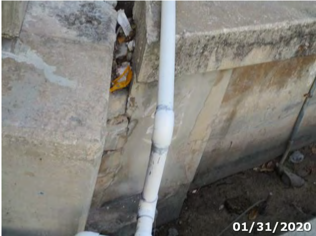
Photo 8475-01 (Element/Env 8475/4: R/Conc Walls)
