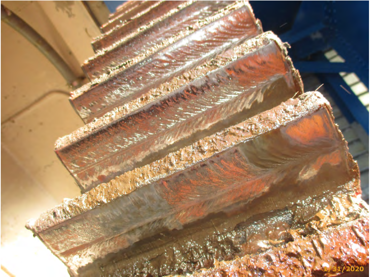
Photo 8540-M02 (Element/Env 8540/4: Open Gearing)
