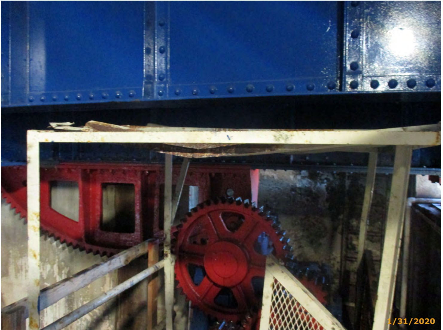
Photo 8540-M01 (Element/Env 8540/4: Open Gearing)
