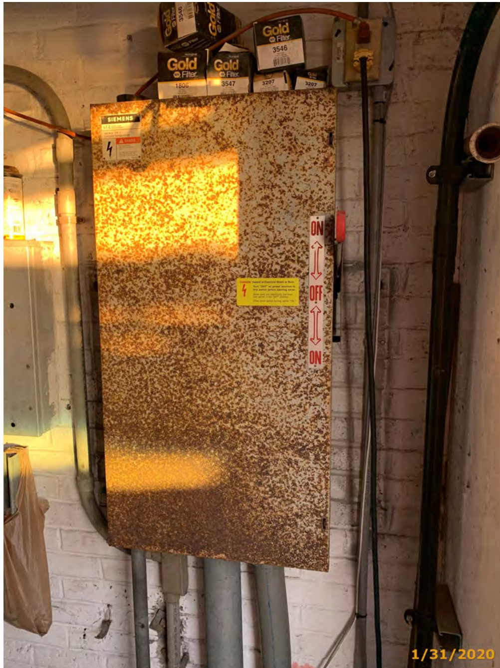
Photo 8545-E04 (Element/Env 8545/4: Emergency Drive)
