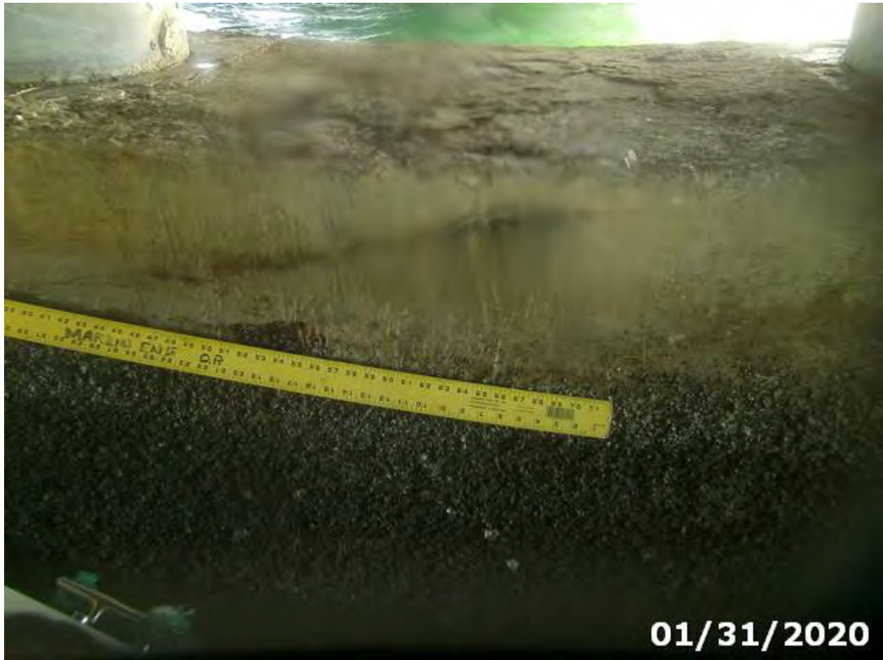
Photo 220-02 (Element/Env 220/4: Re Conc Pile Cap/Ftg)
