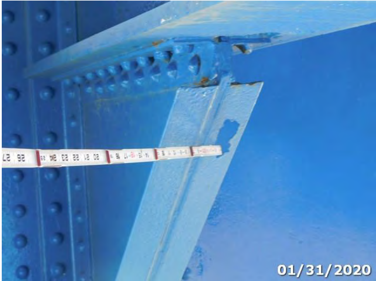
Photo 152-06 (Element/Env 152/4: Steel Floor Beam)
