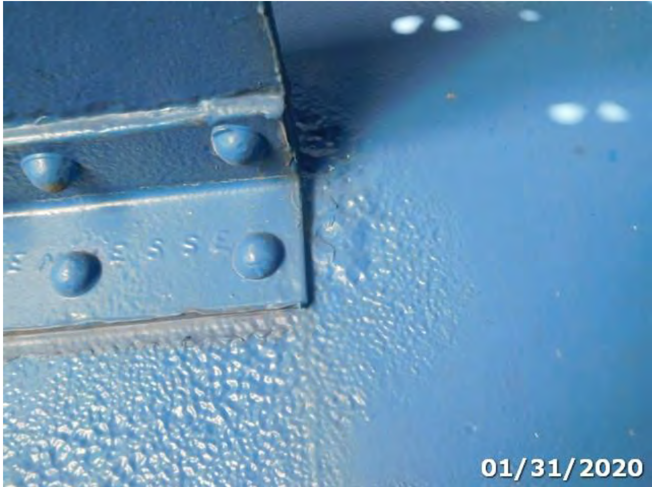
Photo 152-02 (Element/Env 152/4: Steel Floor Beam)
