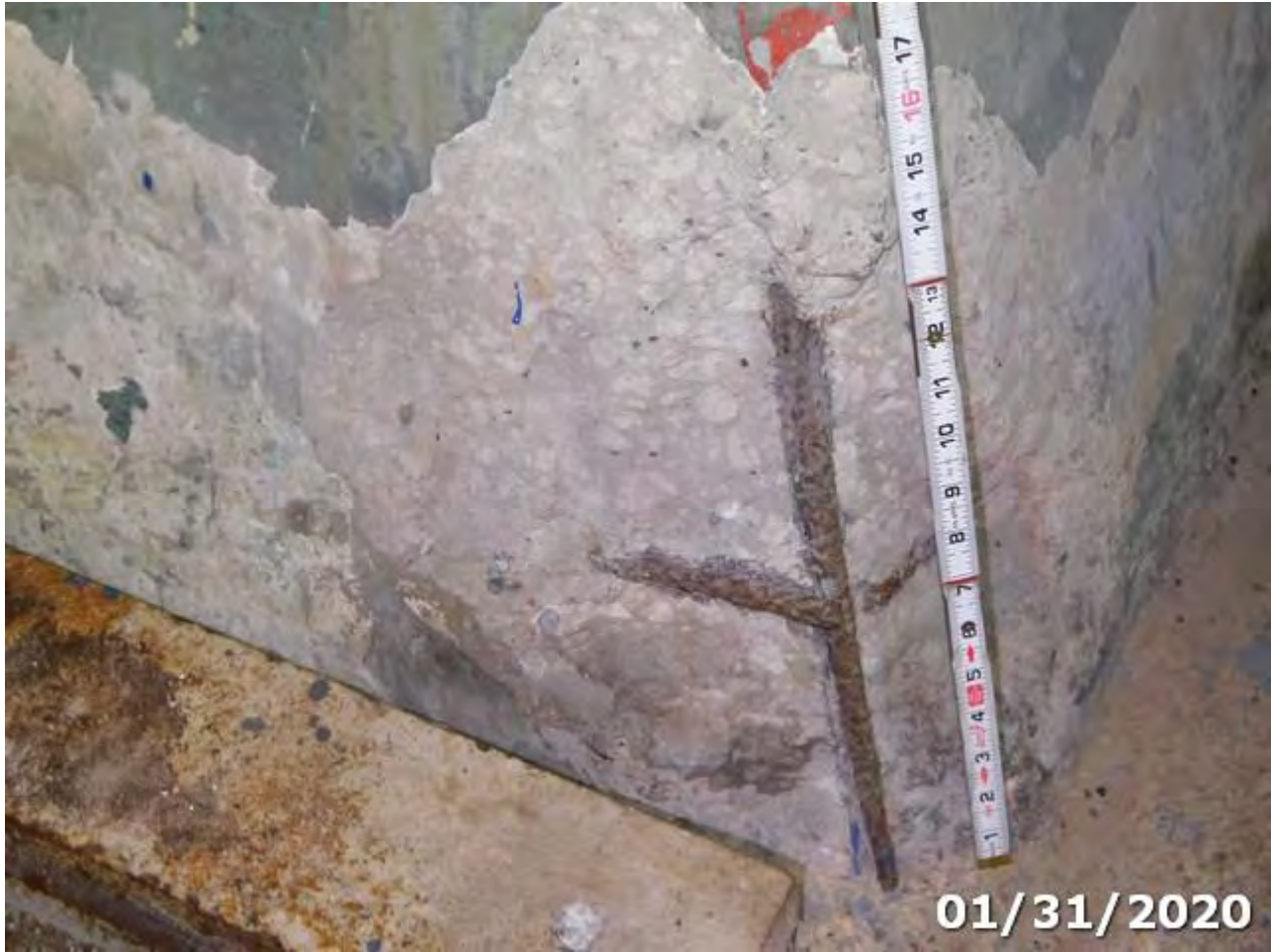
Photo 210-03 (Element/Env 210/4: Re Conc Pier Wall)
