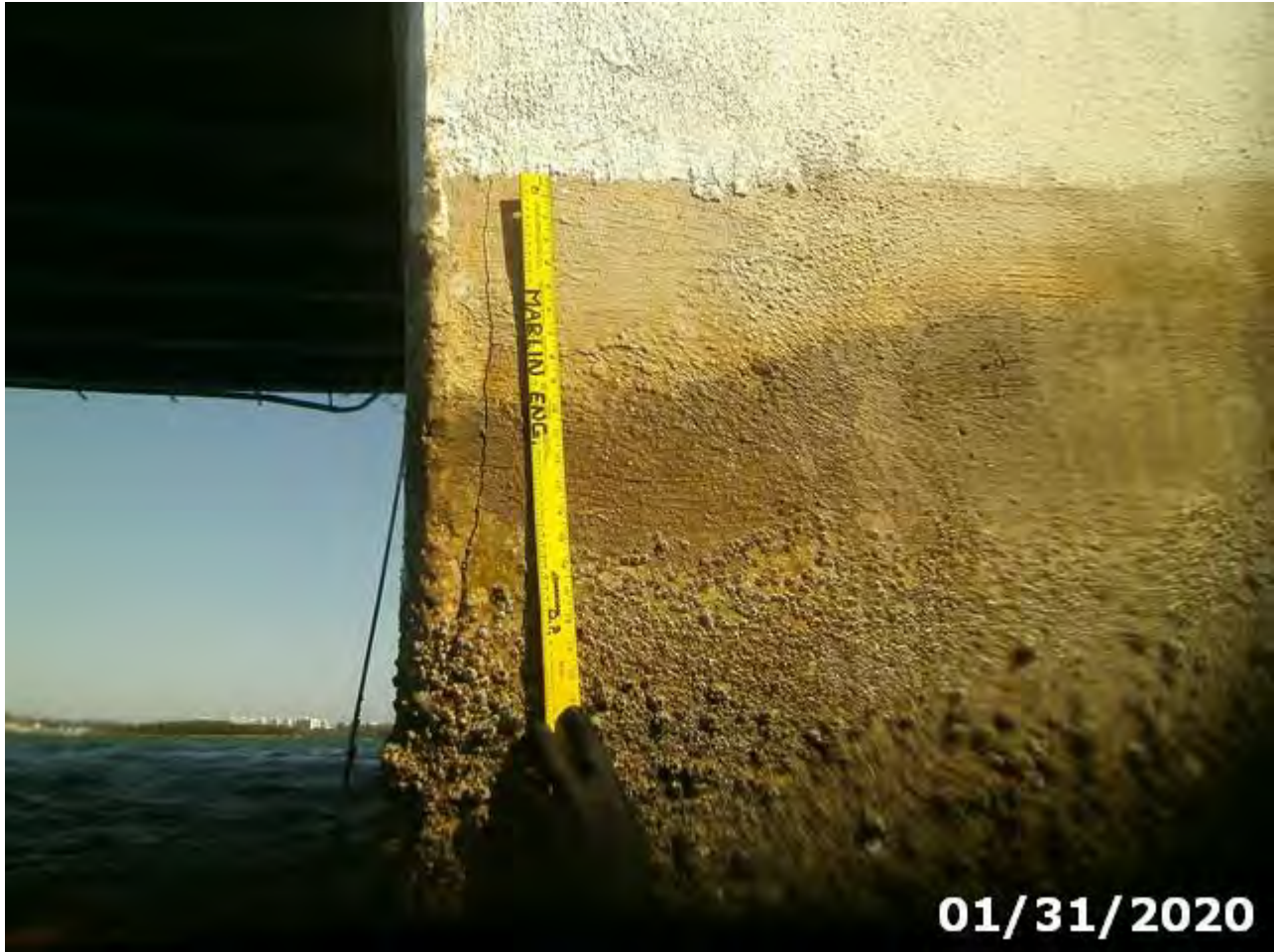
Photo 210-08 (Element/Env 210/4: Re Conc Pier Wall)
