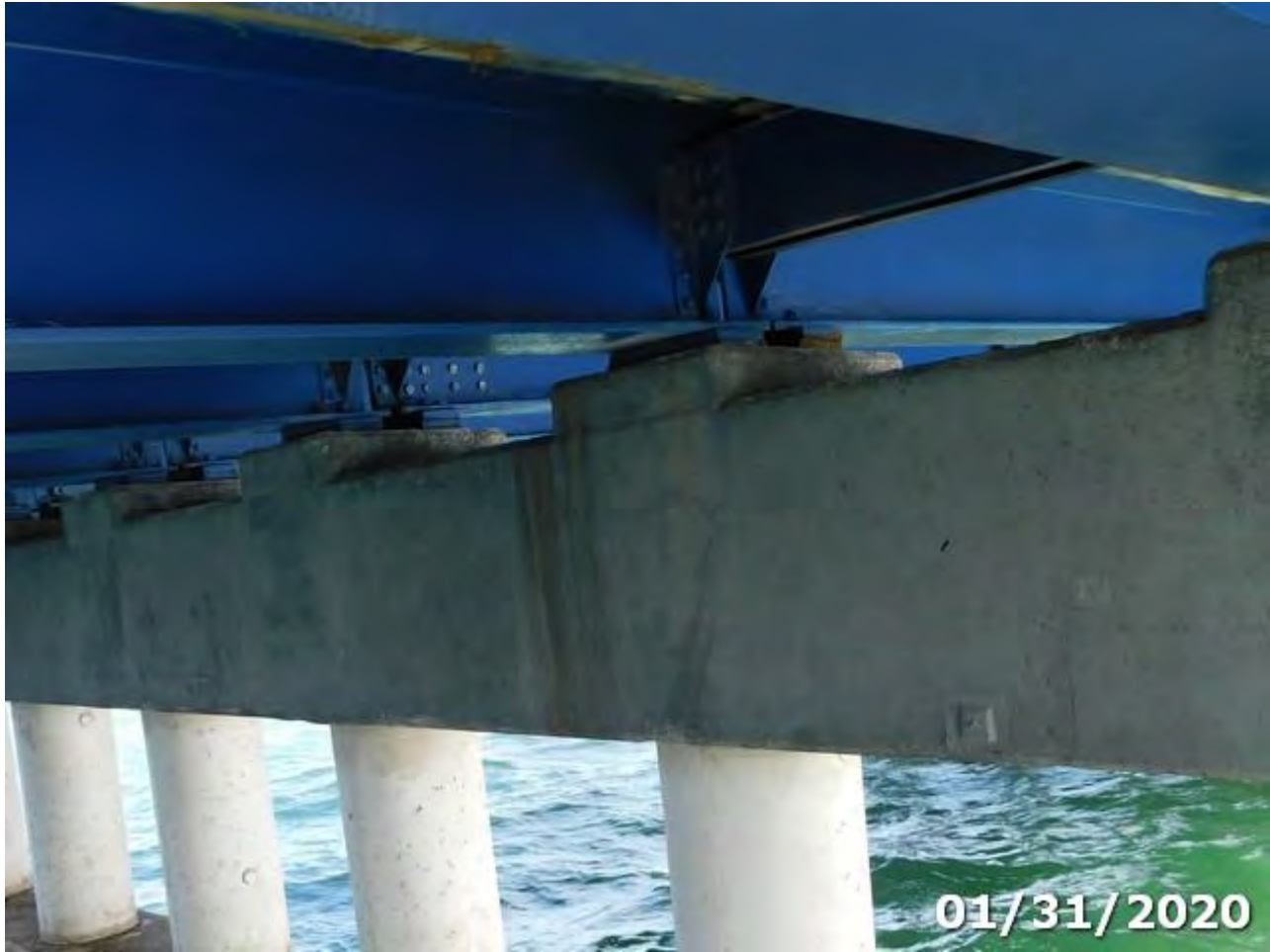
Photo 311-01 (Element/Env 311/4: Moveable Bearing)
