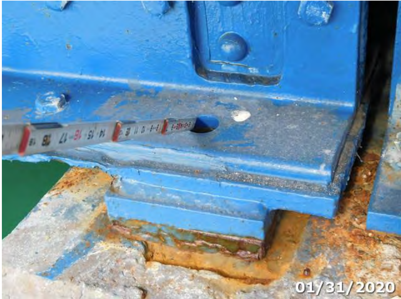
Photo 313-03 (Element/Env 313/4: Fixed Bearing)
