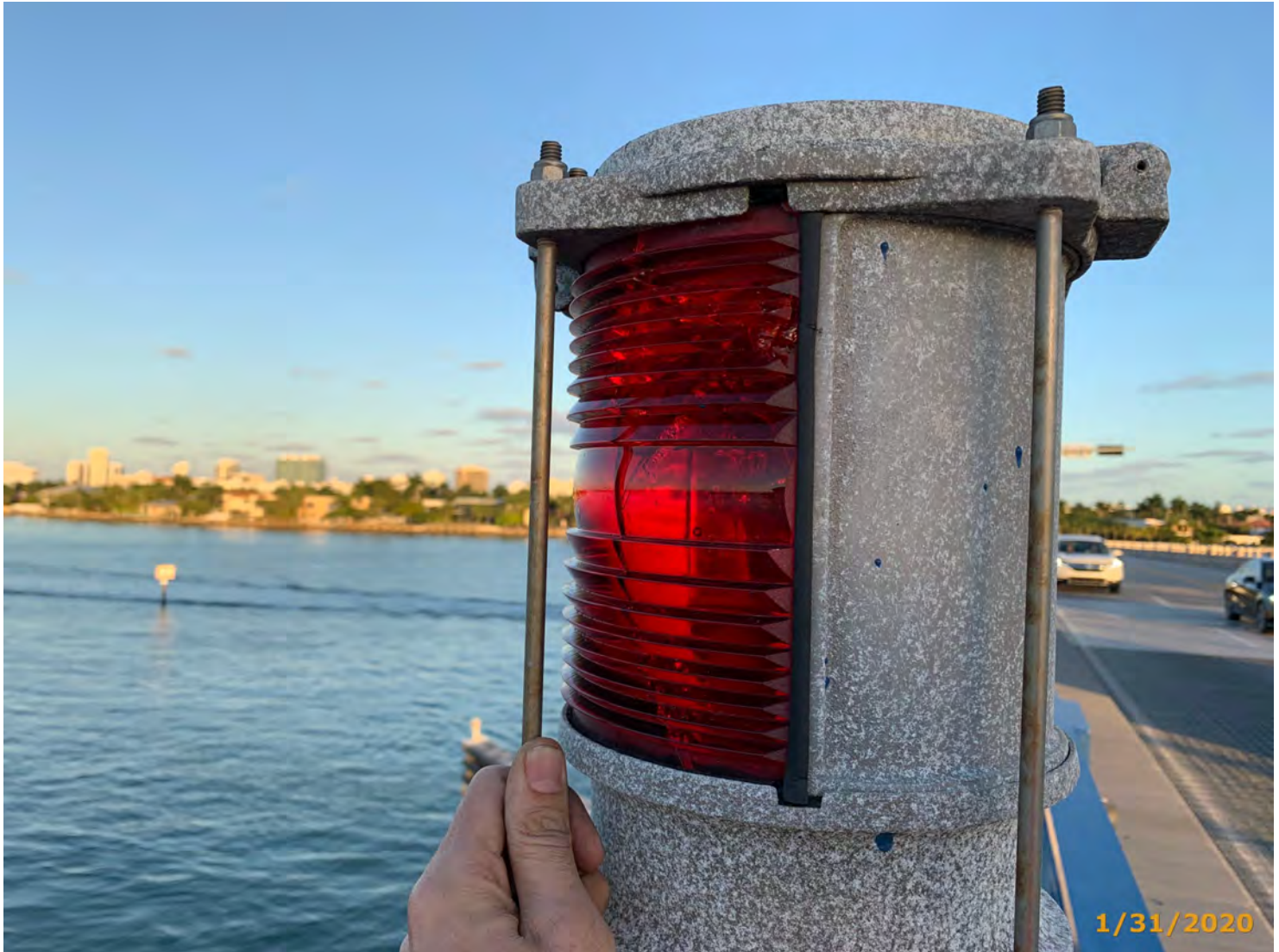
Photo 8580-E01 (Element/Env 8580/4: Navigational Lights)
