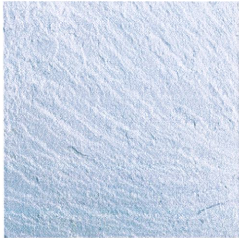
WHITE SLATE CLADDING ON PLANTER WALLS
