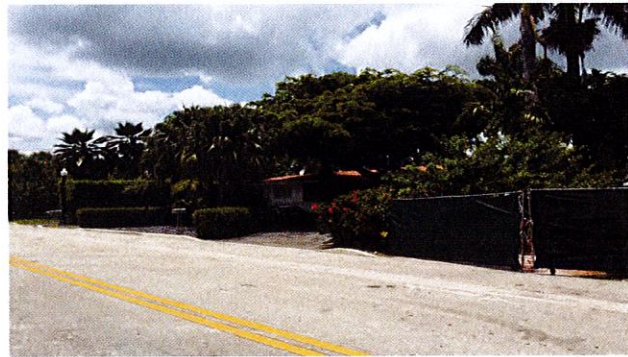
WEST SIDE ADJOINING LOT
