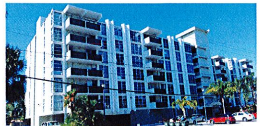
ADJACENT NORTH NEIGHBOR
