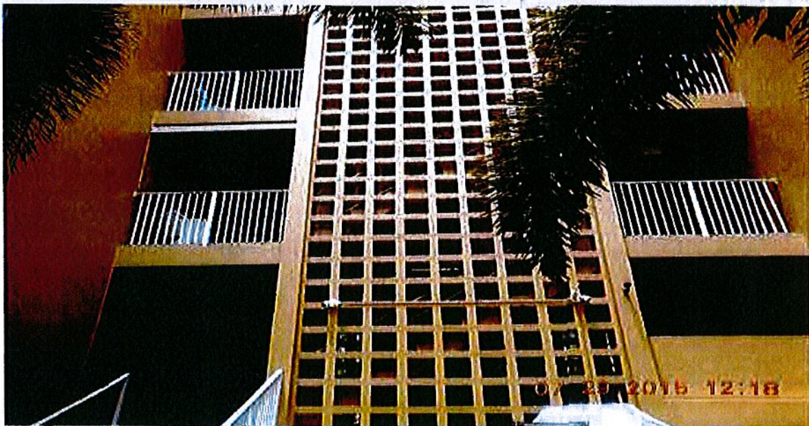
Stairwell view- No violations observed.
