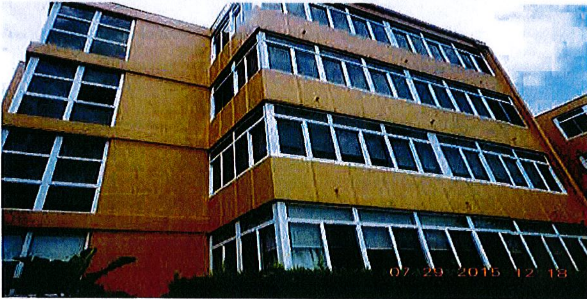
Rear view- No violations observed.
