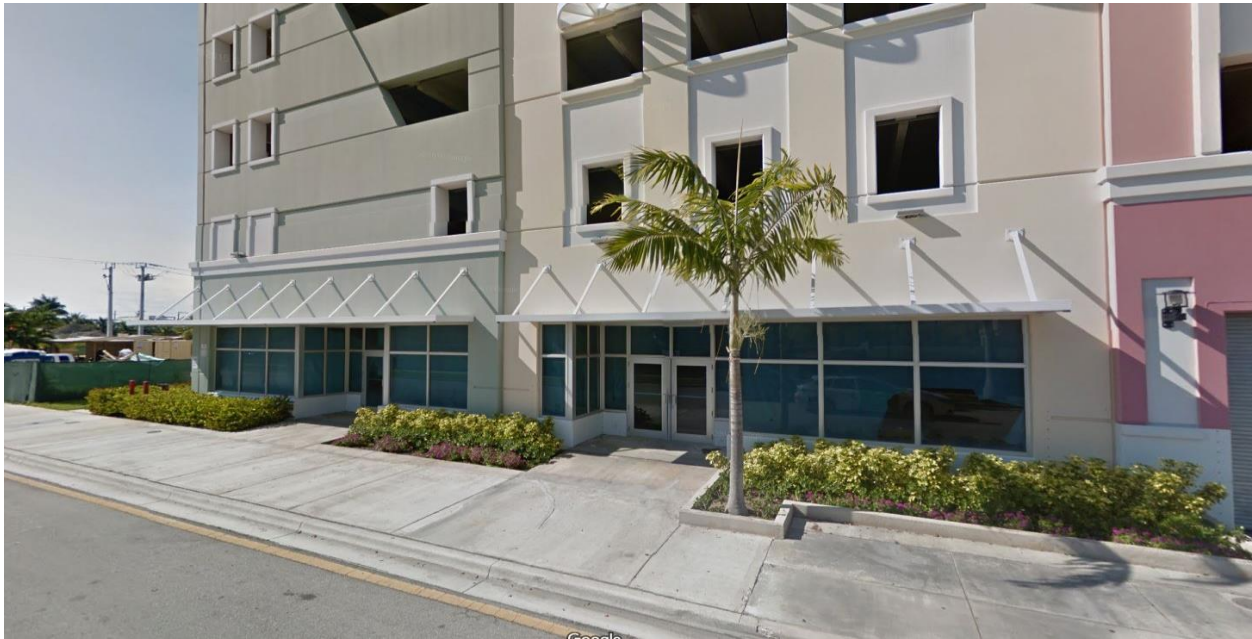
Figure 1 – Exterior view of proposed Bay Harbor Community Center
