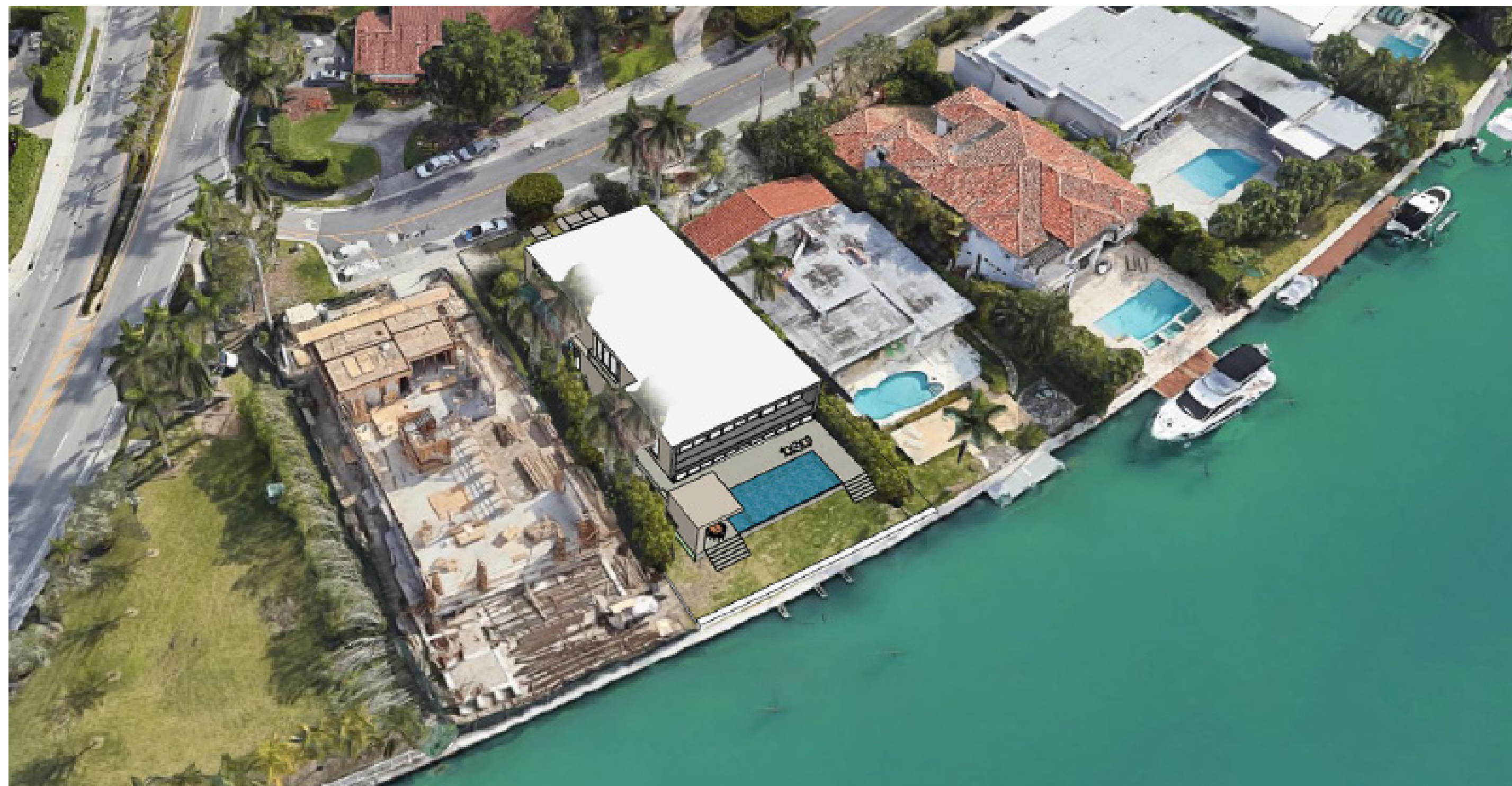
WEST (REAR) AERIAL VIEW
