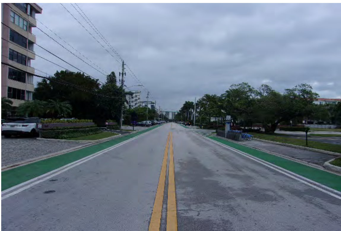
LOOKING NORTHERLY ON WEST BAY HARBOR ISLAND DRIVE – SUBJECT TO RIGHT
