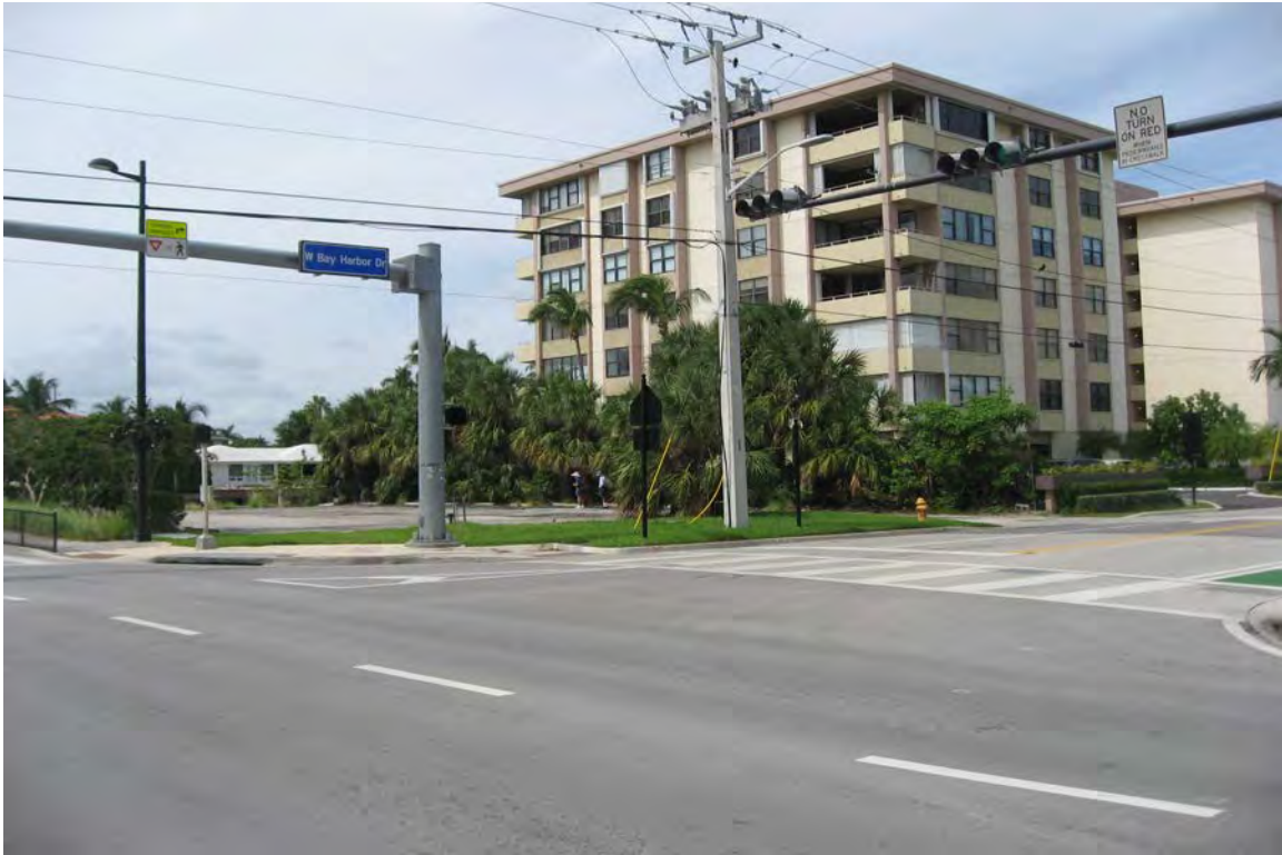
LOOKING NORTHWESTERLY AT SUBJECT FROM WEST BAY HARBOR DRIVE
