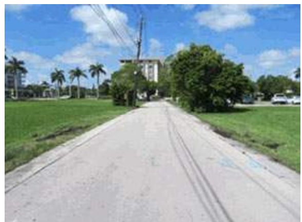
Right-of-Way - Facing West
