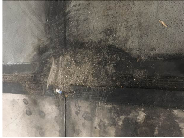
Expansion joint at ramp
