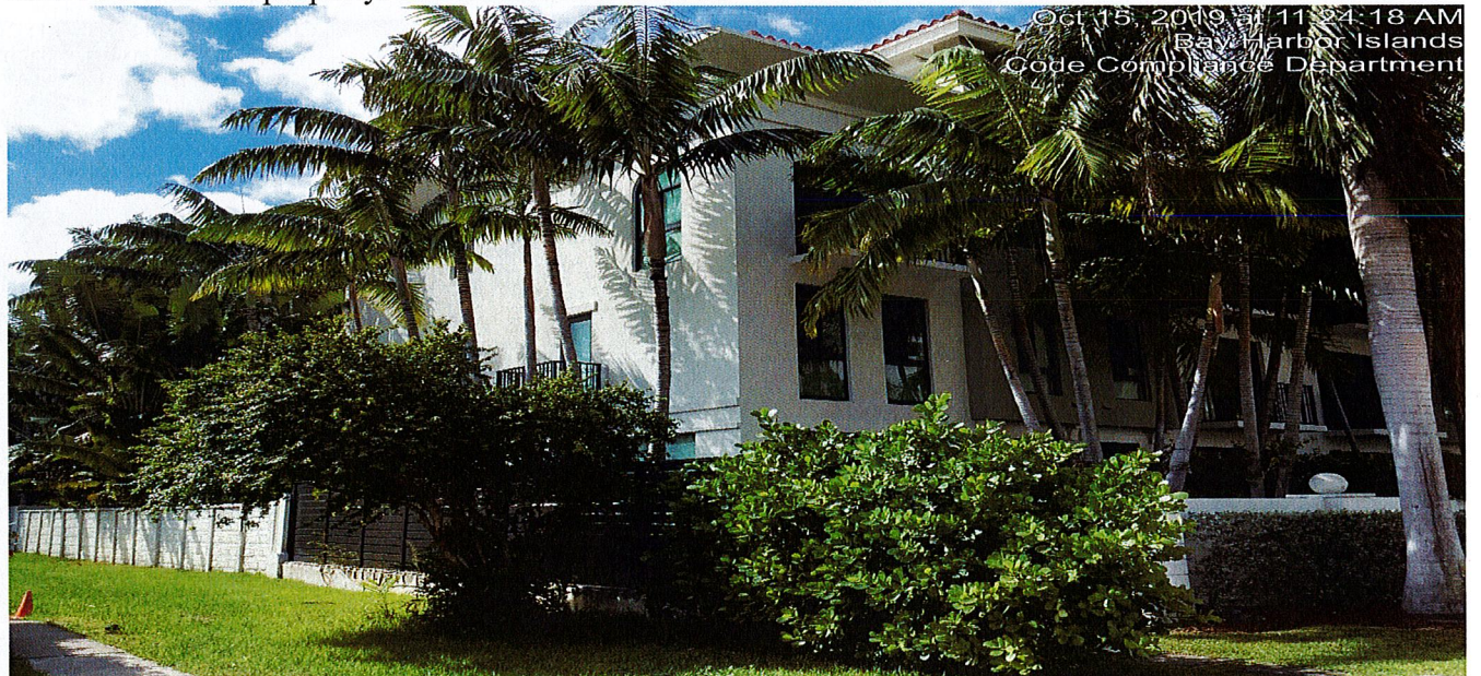
No violations observed on the east side of the building.
