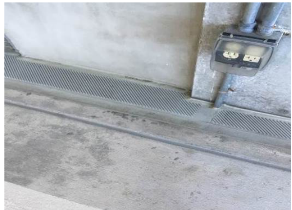
Premold expansion joint at stair/elevator tower
