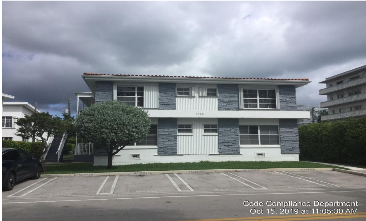
Front View of the property- Tree removed and not replaced.
