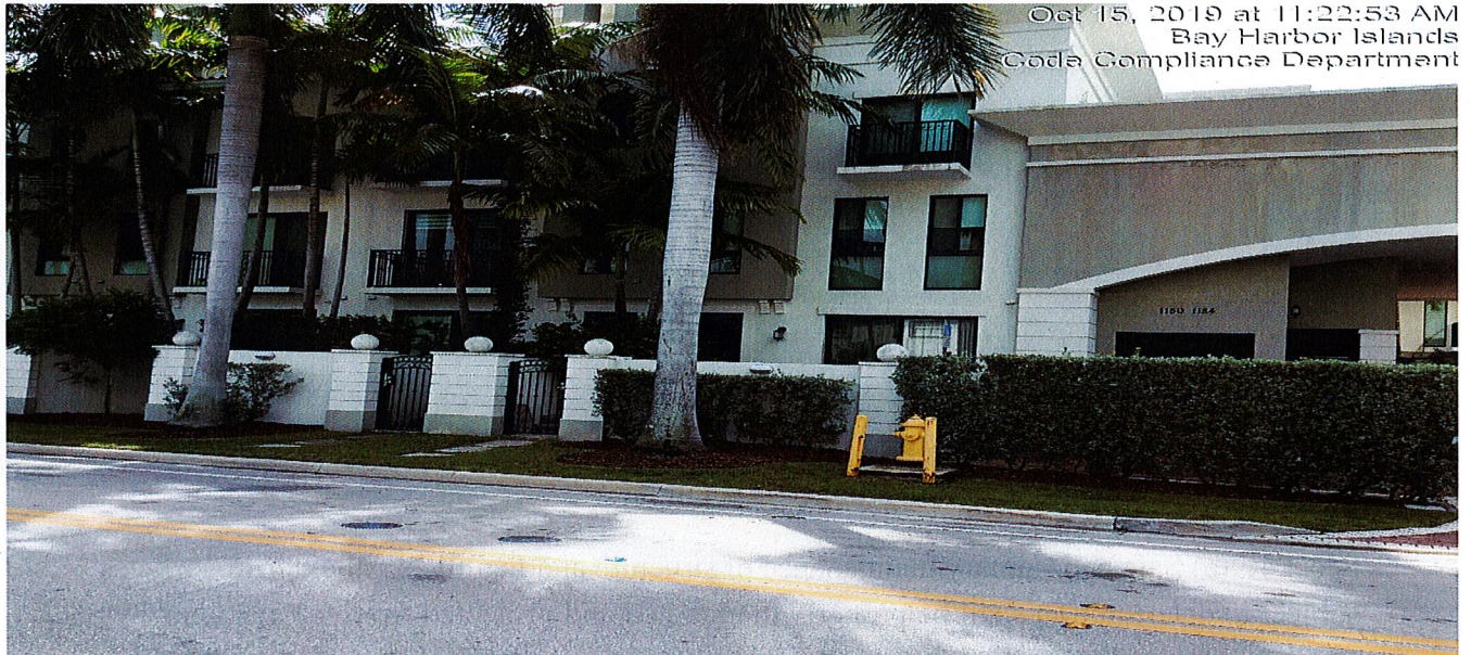
Street view of the property. No violations observed.
