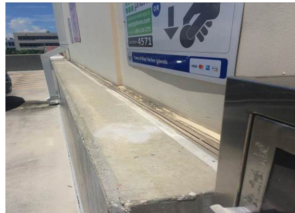
Comp. seal expansion joint along top spandrel
